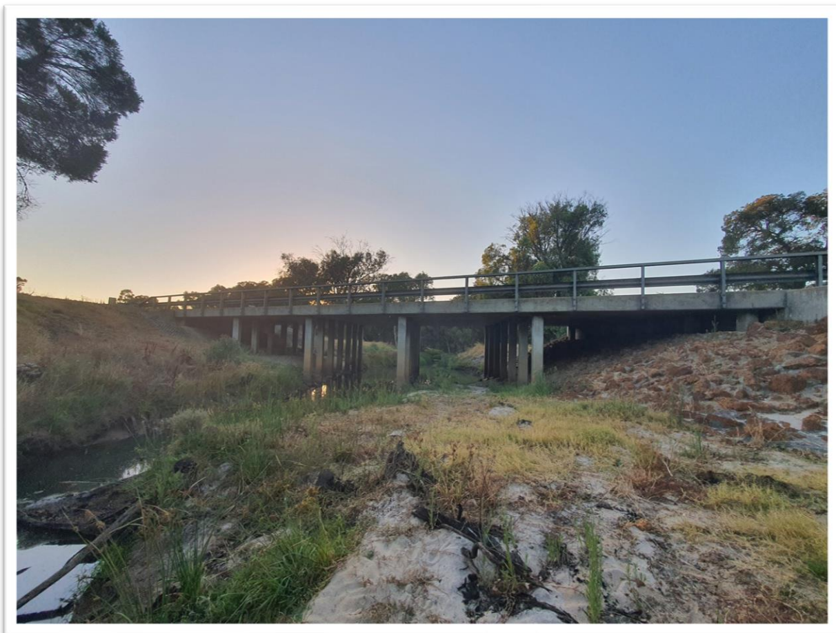
Plate 2: Abba River Bridge Looking Upstream
