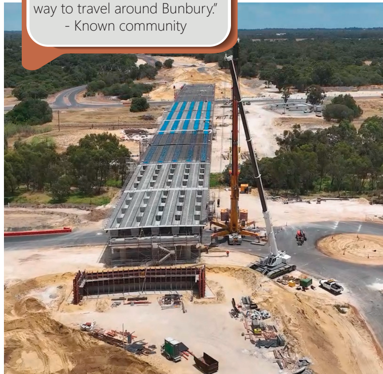
The Golding Crescent and Boyanup-Picton Road overpass bridge
