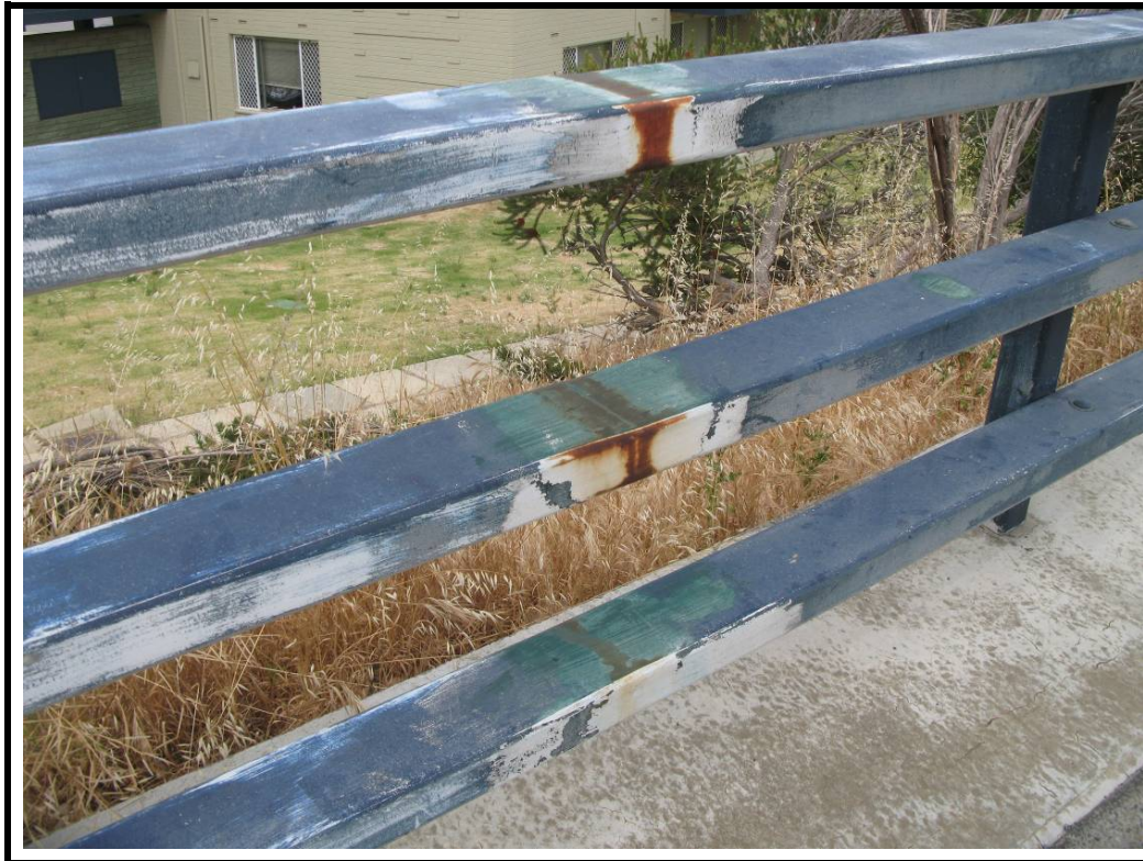
Photo No. 5: Corrosion to welded splices on guardrail, weathered paint system
