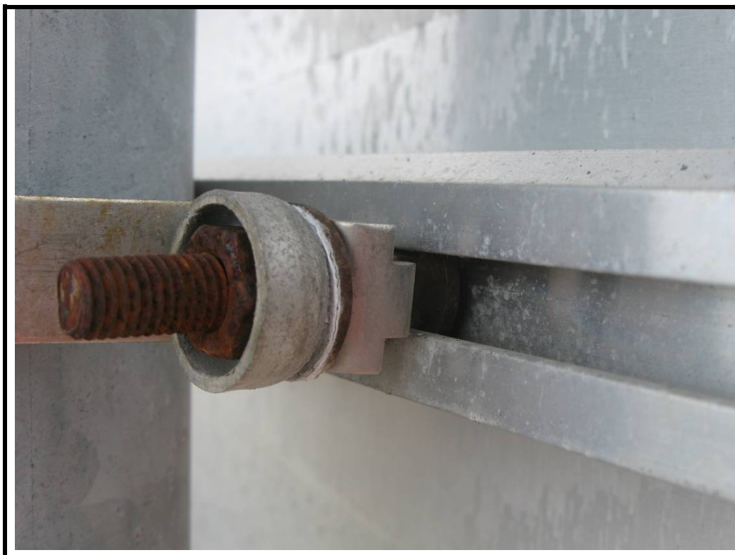
Photo No. 20: Galvanic corrosion to sign mounting bolts (typical)
