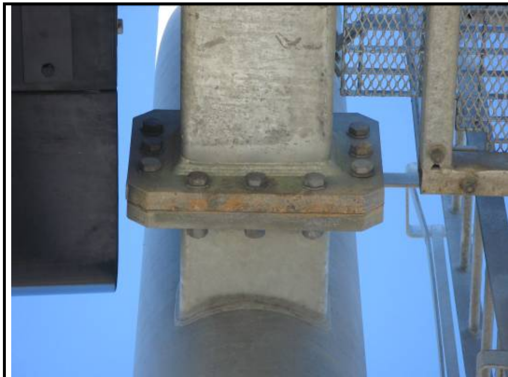
Photo No. 4: Lower bolted connection between beam and column, note minor discolouration
