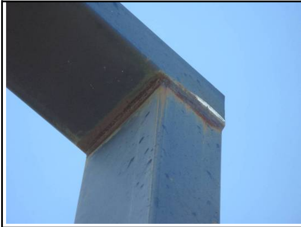
Photo No. 5: LHS connection of Gantry Column to Gantry Beam, note corrosion
