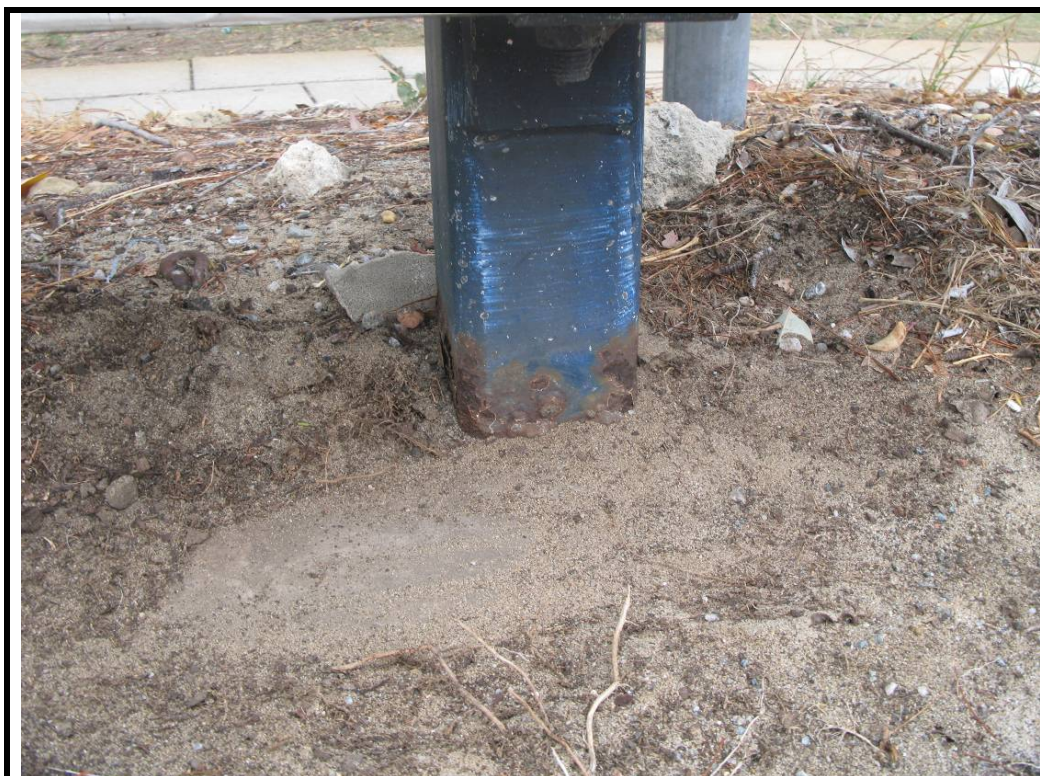
Photo No. 6: Corrosion at foot of guardrail posts
