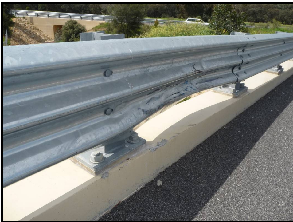
Photo 2 - MINOR IMPACT DAMAGE TO BARRIER, CONNECTION STILL OKAY (Indicative photo only, representative of similar defects for a gantry)
