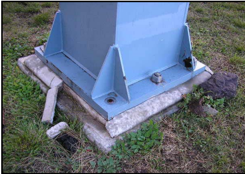
Photo 15 - FAILED ANCHOR BOLTS – NO WASHERS – CRACKED MORTAR UNDER BASE PLATE – MINOR CORROSION TO GUSSET AND BASE PLATES (FOR LEVEL 2 INSPECTION OF ANCHOR BOLTS: CS4, FAILED BOLTS) (FOR LEVEL 2 INSPECTION OF MORTAR GROUT PAD: CS3, SOME MORTAR LOSS) (FOR LEVEL 2 INSPECTION OF GUSSET: CS2, SURFACE CORROSION)
