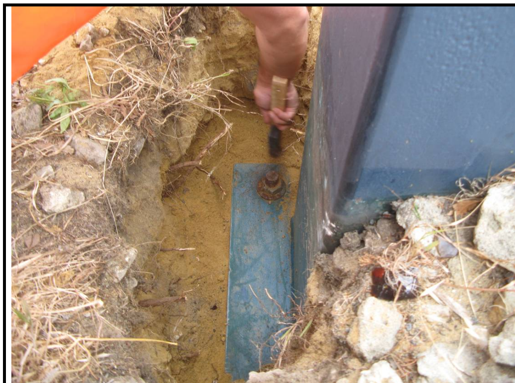
Photo No. 18: LHS column base plate exposed
