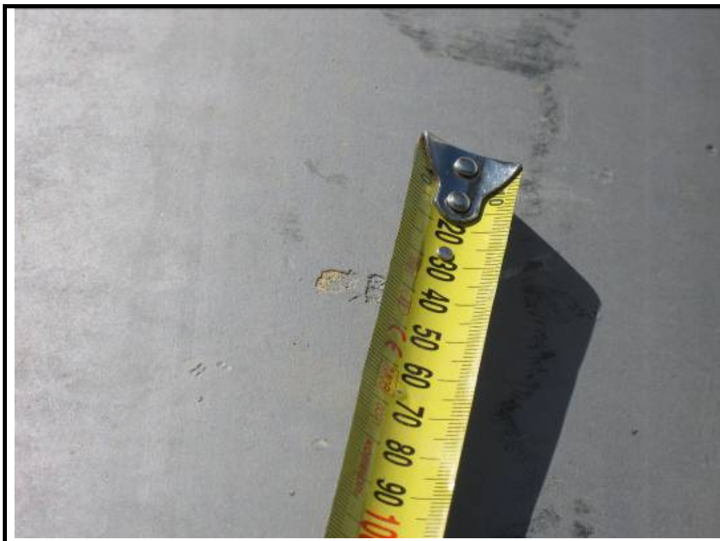
Photo No. 6: Minor chip to column surface (typical)
