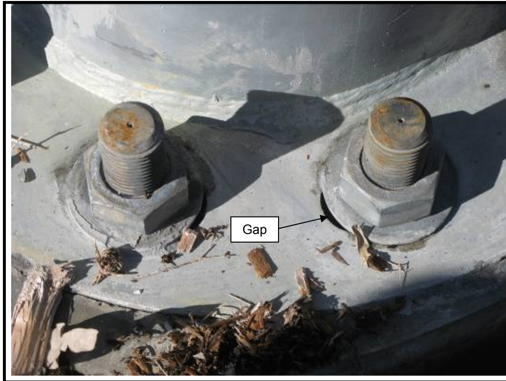
Photo No. 7: Base plate weld to column – also note surface corrosion to HD bolts and gap
