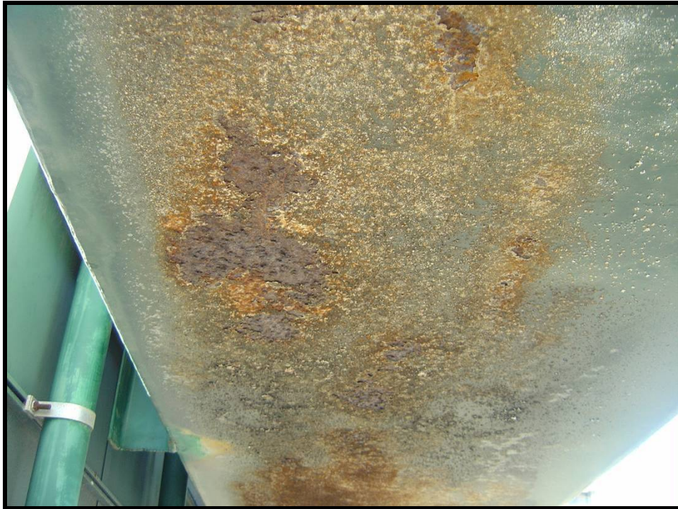
Photo 4 - ADVANCED CORROSION TO SOFFIT OF GANTRY BEAM (FOR LEVEL 2 INSPECTION: CS3, PITTING IN ISOLATED AREAS)
