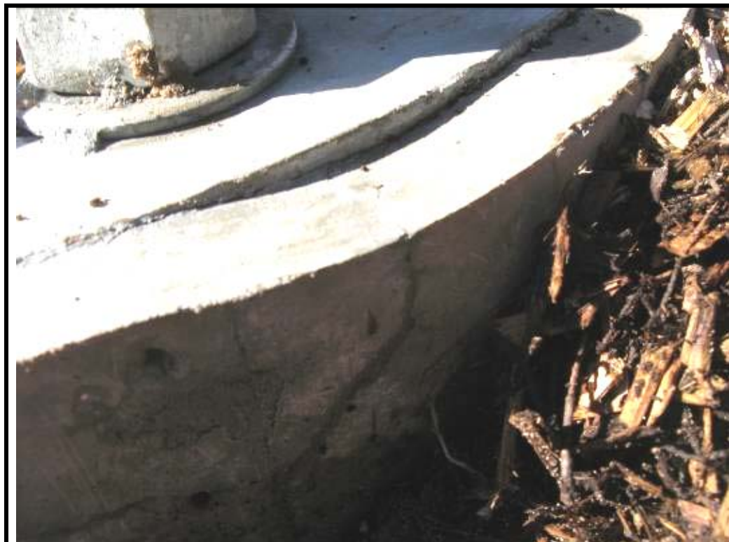
Photo No. 8: Hairline crack to mortar
