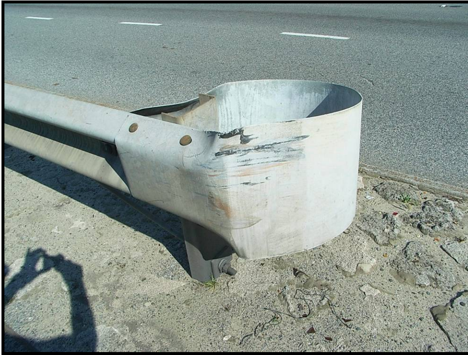
Photo 3 - MINOR IMPACT DAMAGE TO END TERMINAL (ALSO NOTE, END TERMINAL IS SUB-STANDARD) (Indicative photo only, representative of similar defects for a gantry)
