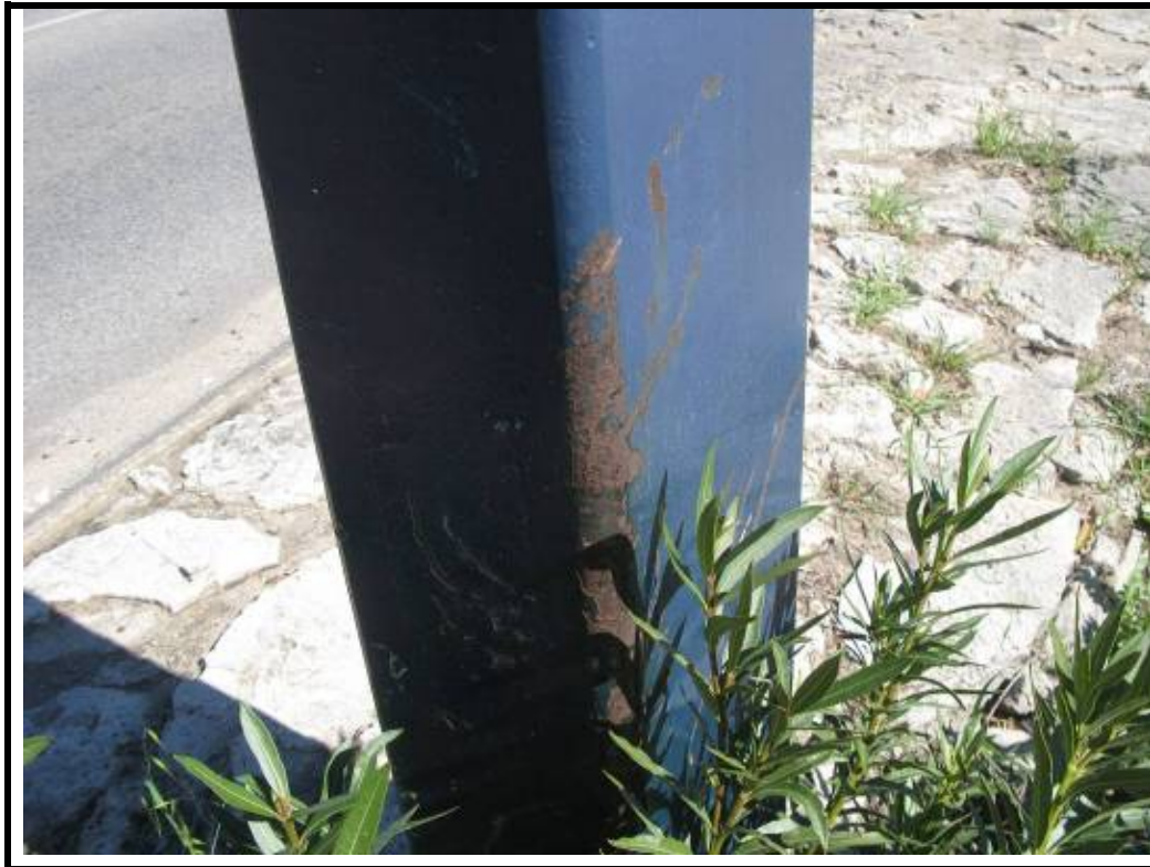
Photo No. 7: Surface corrosion to RHS column, note stone pitching
