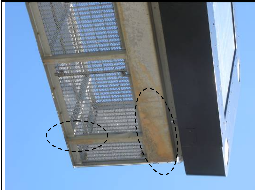
Photo No. 5: Possible corrosion to underside of cantilever end of beam and walkway support
