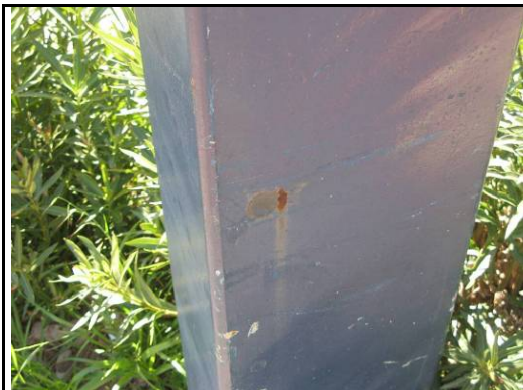
Photo No. 8: Surface corrosion to LHS column
