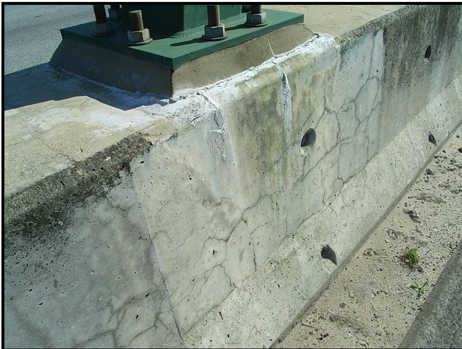
Photo 13 - CRACKING TO FOOTING (FOR LEVEL 2 INSPECTION: CS2, FINE CRACKING WITH NO SPALLING)
