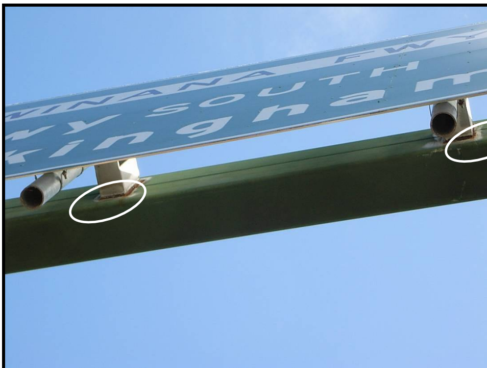
Photo 21 - CORROSION TO SIGN MOUNTING BRACKET WELDS (FOR LEVEL 2 INSPECTION: CS2, MINOR CORROSION)
