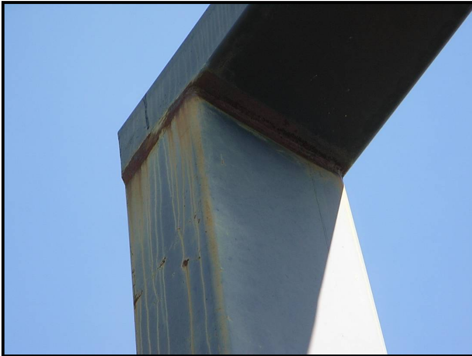
Photo 6 - CORROSION TO WELDS AT BEAM AND COLUMN CONNECTION (FOR LEVEL 2 INSPECTION: CS2, INSIGNIFICANT SECTION LOSS)
