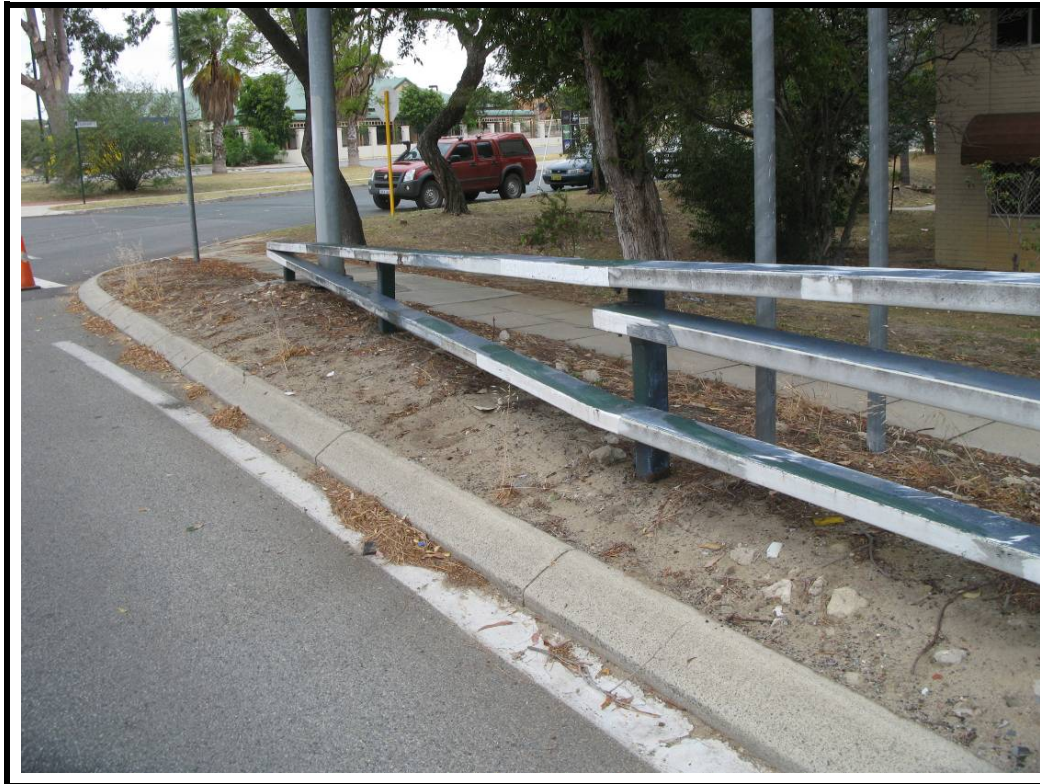
Photo No. 7: Substandard end terminal
