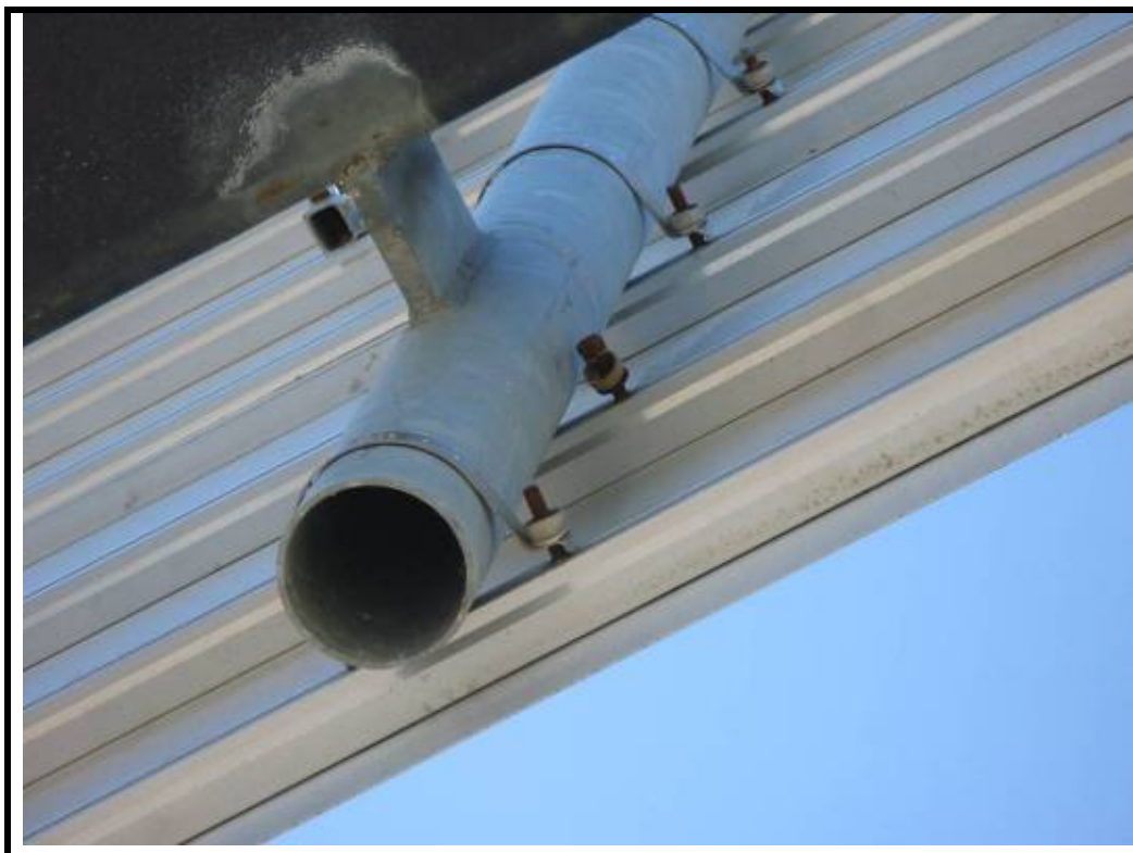
Photo No. 10: Corroded sign attachment bolts
