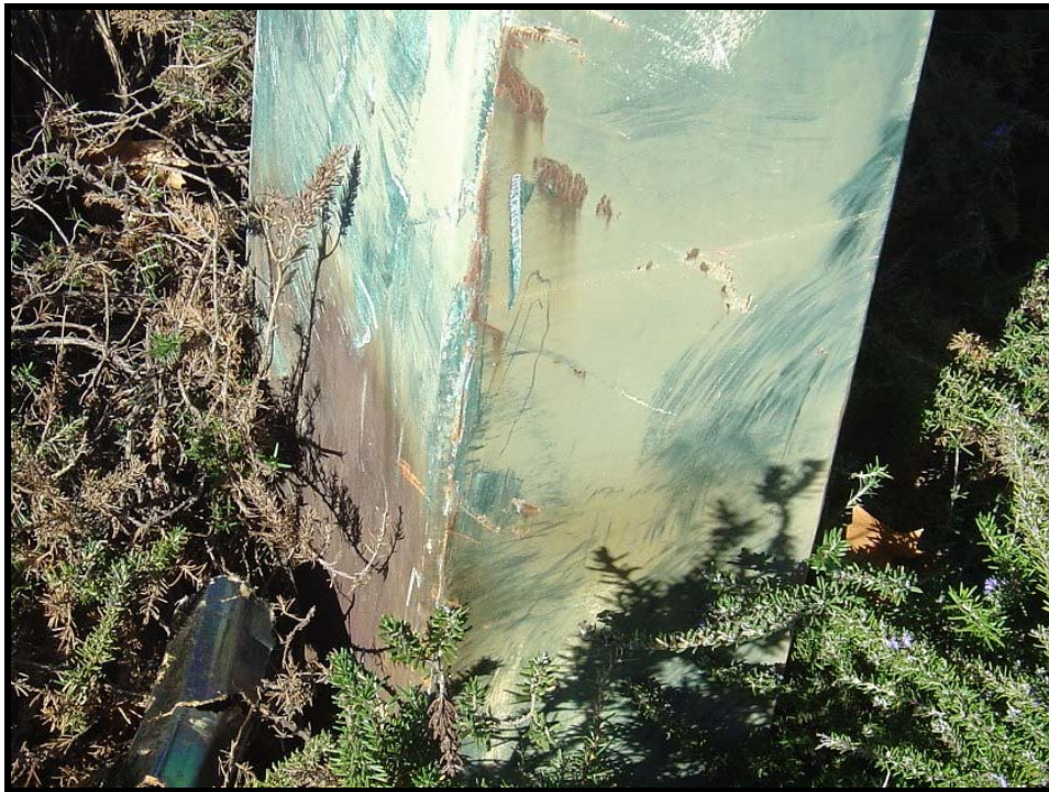
Photo 10 - IMPACT DAMAGE, CORROSION AND DETERIORATED PAINTWORK AT GROUND LEVEL OF COLUMN 1 RIGHT HAND SIDE (FOR LEVEL 2 INSPECTION: CS2, NO DISTORTION OF SHAPE)
