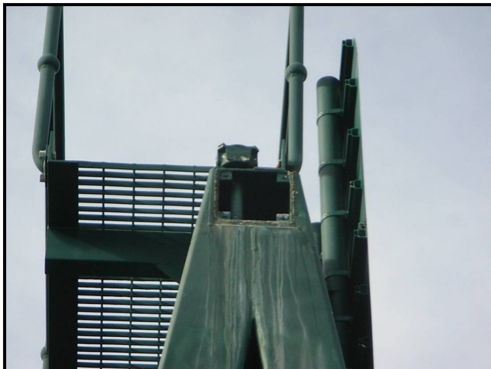
Photo 18 - MISSING ACCESS PLATE AT LEFT HAND SIDE OF GANTRY BEAM
