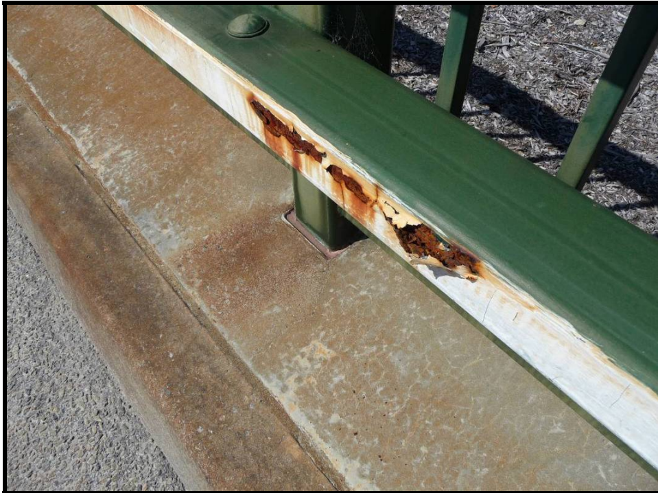
Photo 1 - CORROSION TREATMENT REQUIRED TO LEFT HAND SIDE BARRIER (Indicative photo only, representative of similar defects for a gantry)
