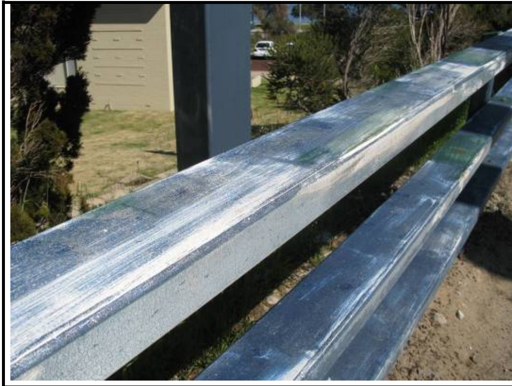
Photo No. 3: 3-rail Barrier protection to LHS column, note weathered paint condition
