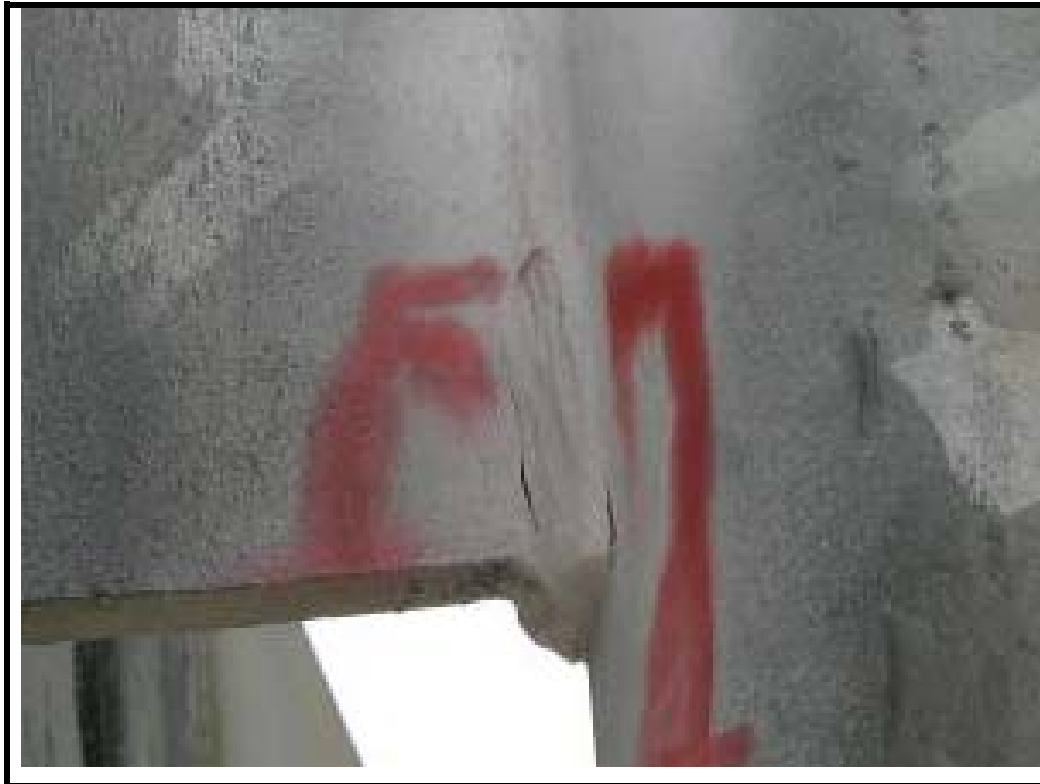
Photo No. 13: Sign connection 1 – close up of lack of fusion
