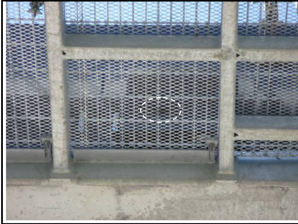
Photo No. 9: Possible corrosion to access walkway
