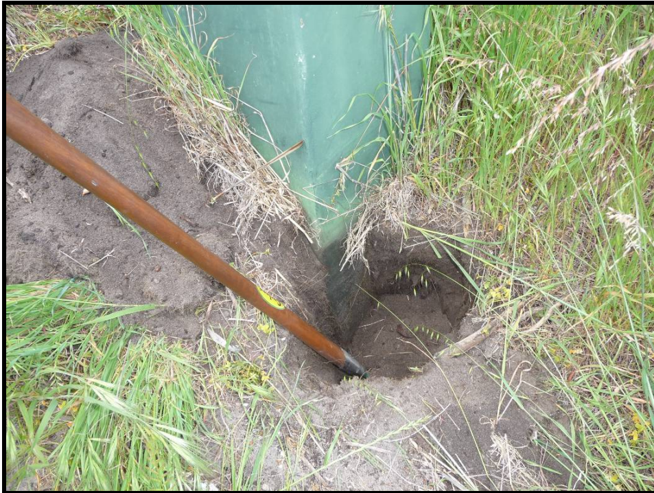
Photo 12 - FOOTING GREATER THAN 500 mm BELOW GROUND LEVEL
