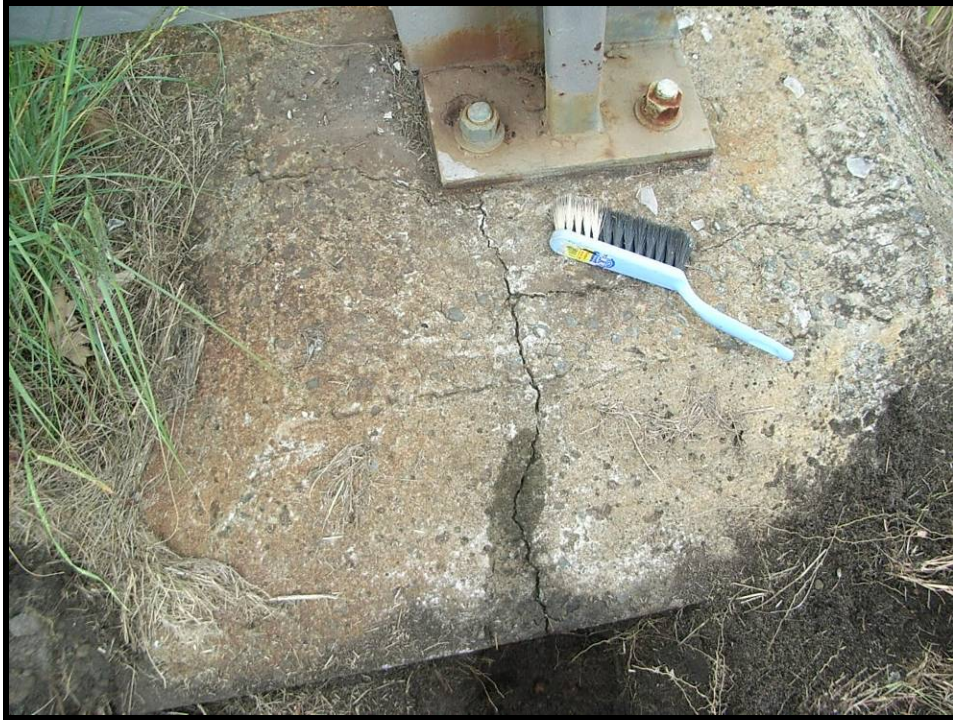
Photo 14 - SHRINKAGE CRACKING TO CONCRETE FOOTING (FOR LEVEL 2 INSPECTION OF FOOTING: CS3, MEDIUM CRACKING)
