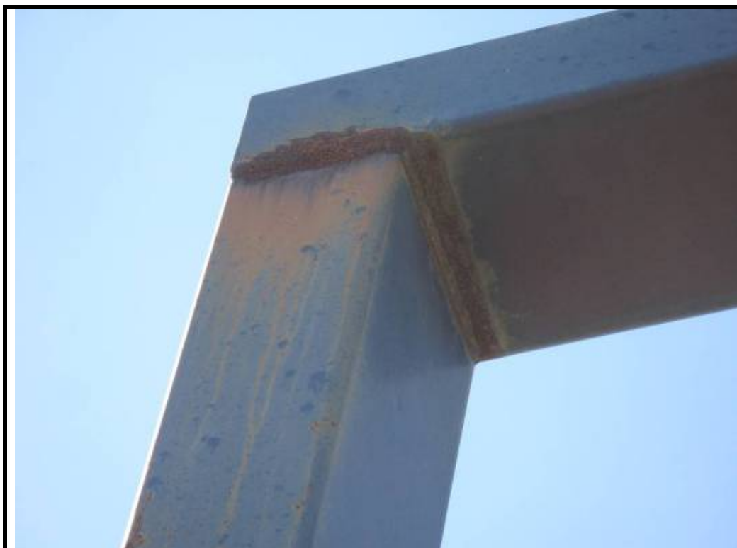
Photo No. 4: RHS connection of Gantry Column to Gantry Beam, note corrosion
