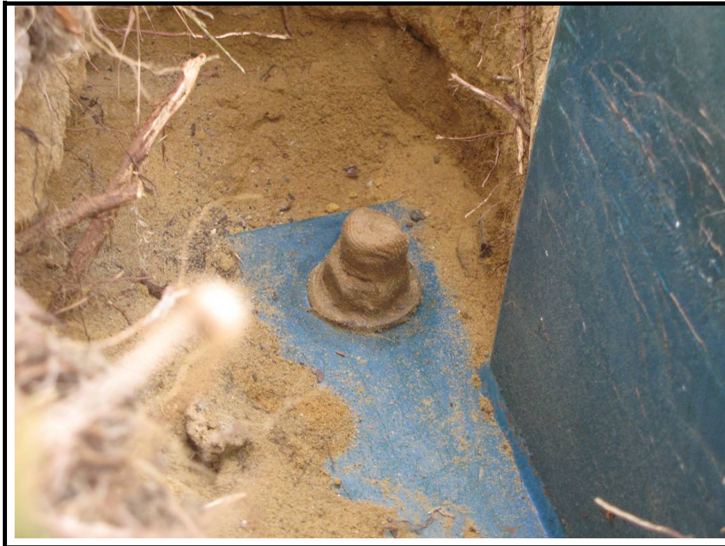
Photo No. 19: HD bolt following treatment with Denso Tape
