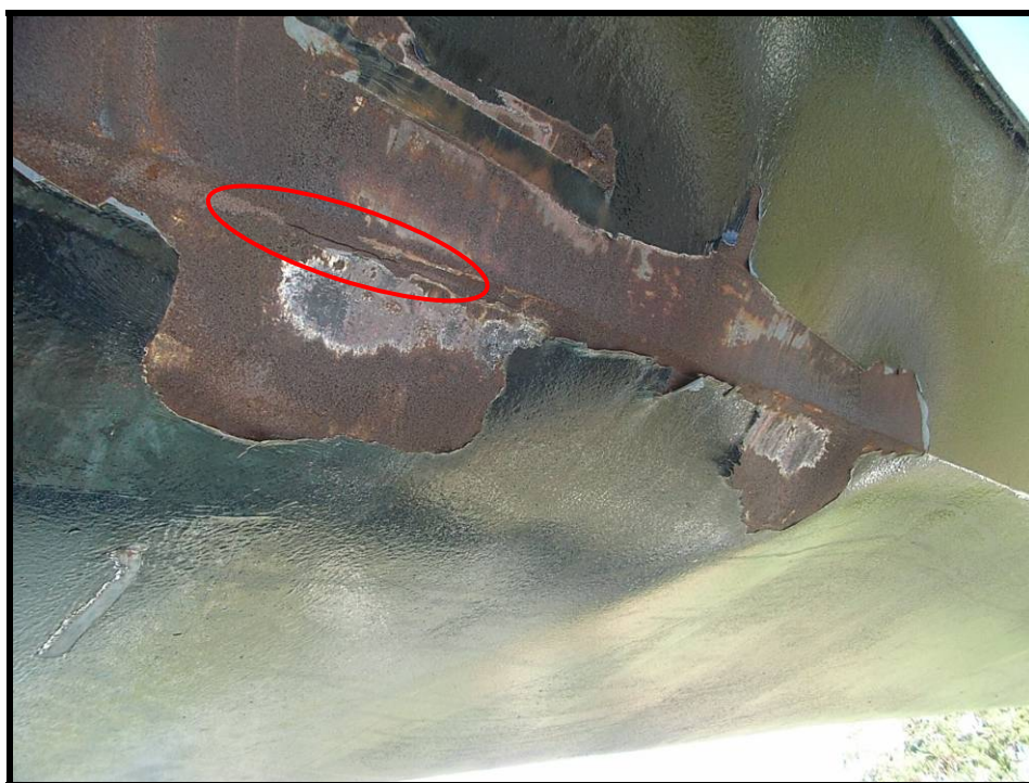
Photo 9 - IMPACT DAMAGE TO SOFFIT, CAUSING CRACK IN WEB/SOFFIT WELD (REFER FOR ENGINEERING INSPECTION AND ASSESSMENT) (FOR LEVEL 2 INSPECTION: CS4, STEEL CRACKING) (Indicative photo only, representative of similar defects for a gantry)
