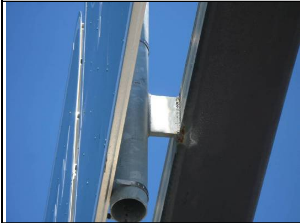
Photo No. 9: Corrosion between sign fixing bracket and gantry beam (typical)
