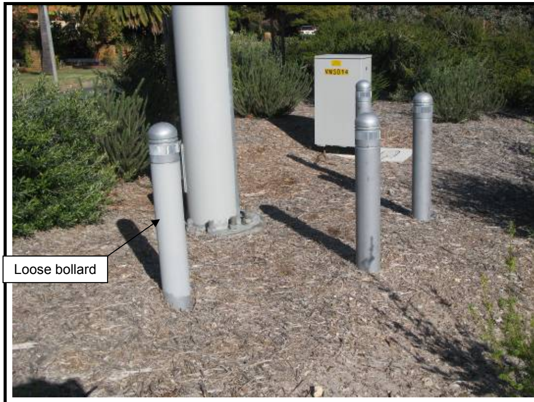
Photo No. 3: 4No. Bollards with reflective tape. 1No. Bollard loose
