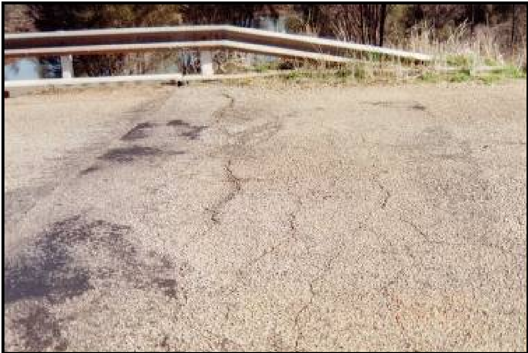
Photo 8 - LARGE TRANSVERSE CRACKS IN ROAD APPROACH
