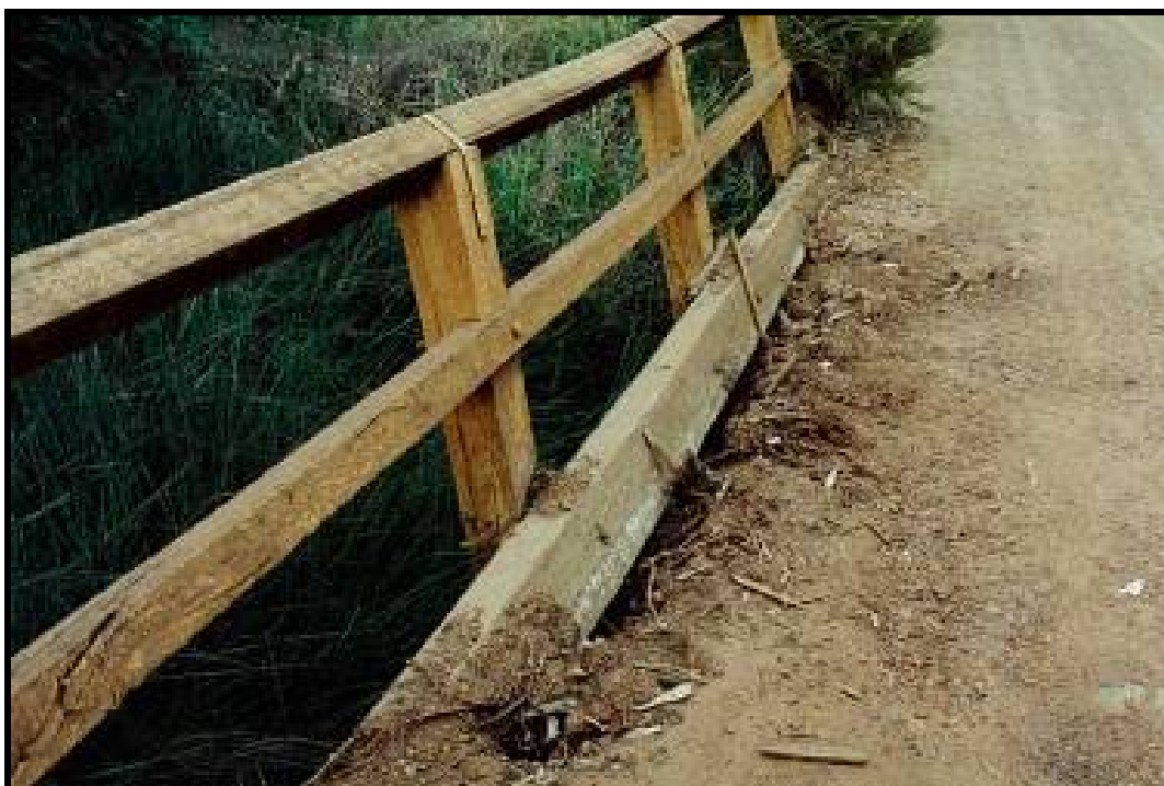
Photo 20 - RAILING LEANING OVER AND KERB DETACHING FROM DECK
