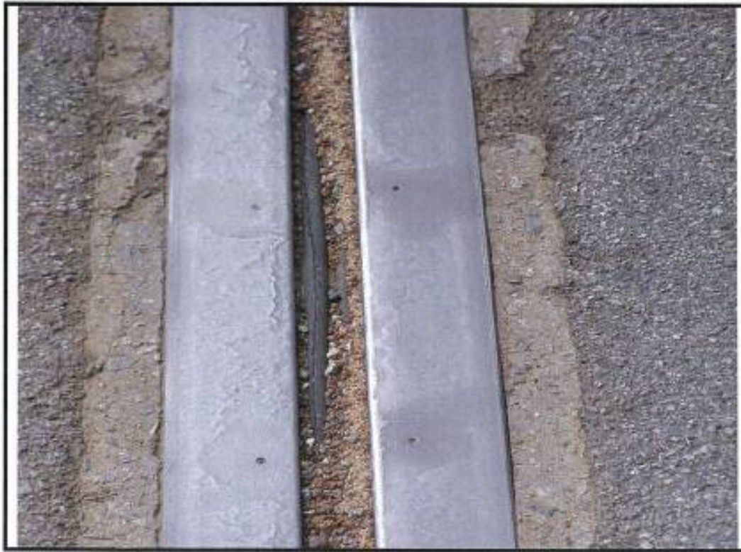
Photo No. 5: Top Surface of Wabo Rubber is Perished
