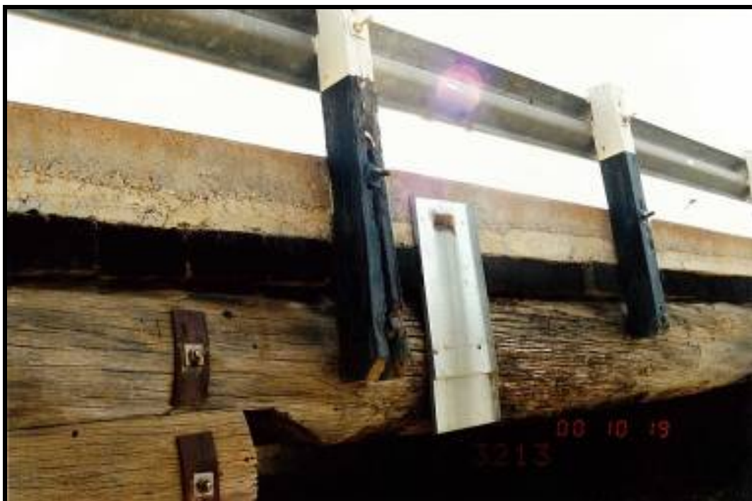
Photo 19 - LARGE VERTICAL SPLIT IN TIMBER POST
