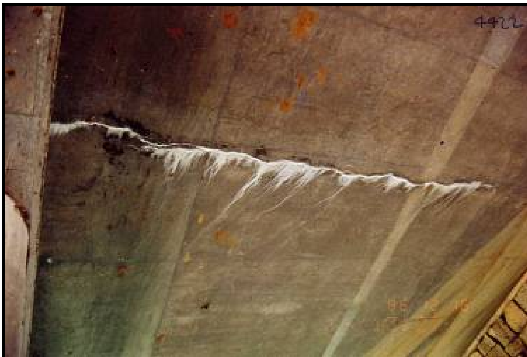
Photo 61 - EFFLORESCENCE FROM CRACK IN DECK SOFFIT
