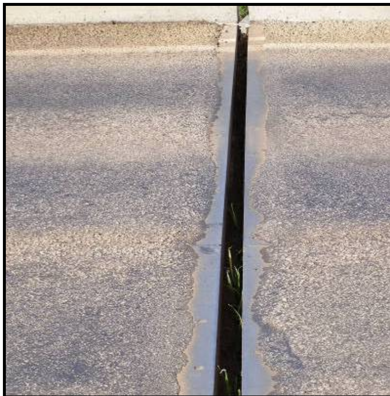
Photo 46 - MISSING SEAL IN DECK JOINT
