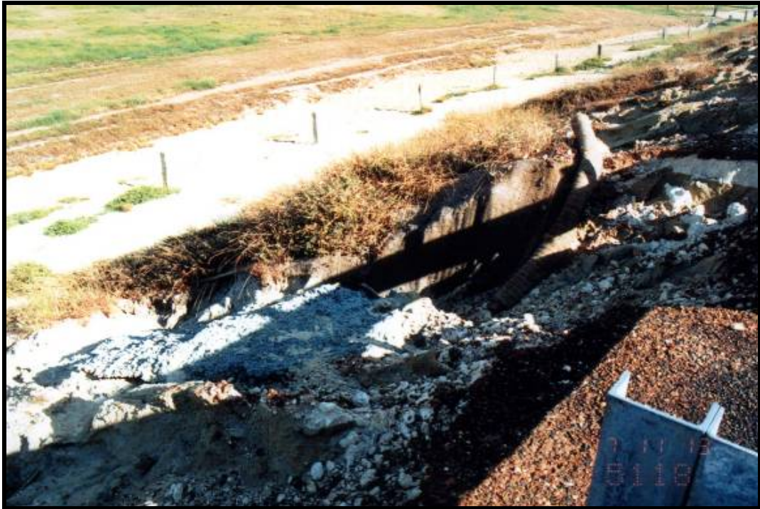
Photo 31 - SCOURING OF EMBANKMENT CAUSED BY EXCESSIVE ROAD RUNOFF
