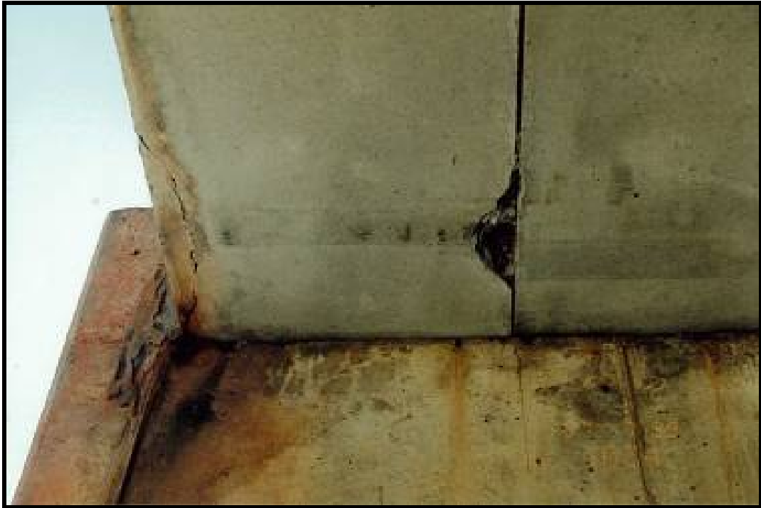
Photo 65 - DAMAGED SECTION OF BEAM (No change since previous inspection)
