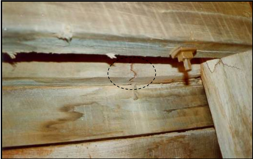
Photo 67 - FAILED REAR HALFCAP
