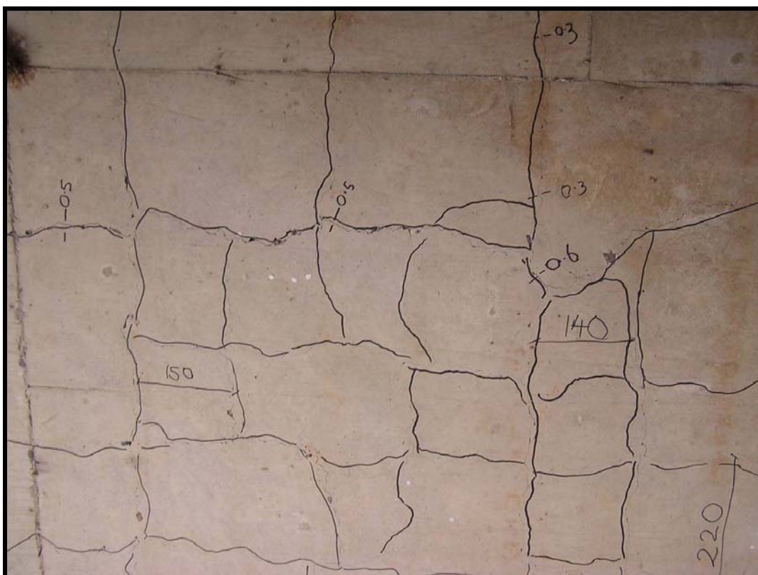
Photo 64 - MEDIUM SIZED CRACKS FORMING DECK BLOCK CRACKING (NOTE: Mapping is not required for L1 inspection but block cracking should be noted)
