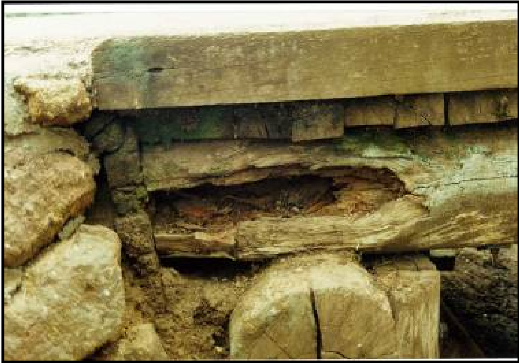
Photo 59 - LARGE ROT ZONE IN THE END OF THE OUTSIDE STRINGER
