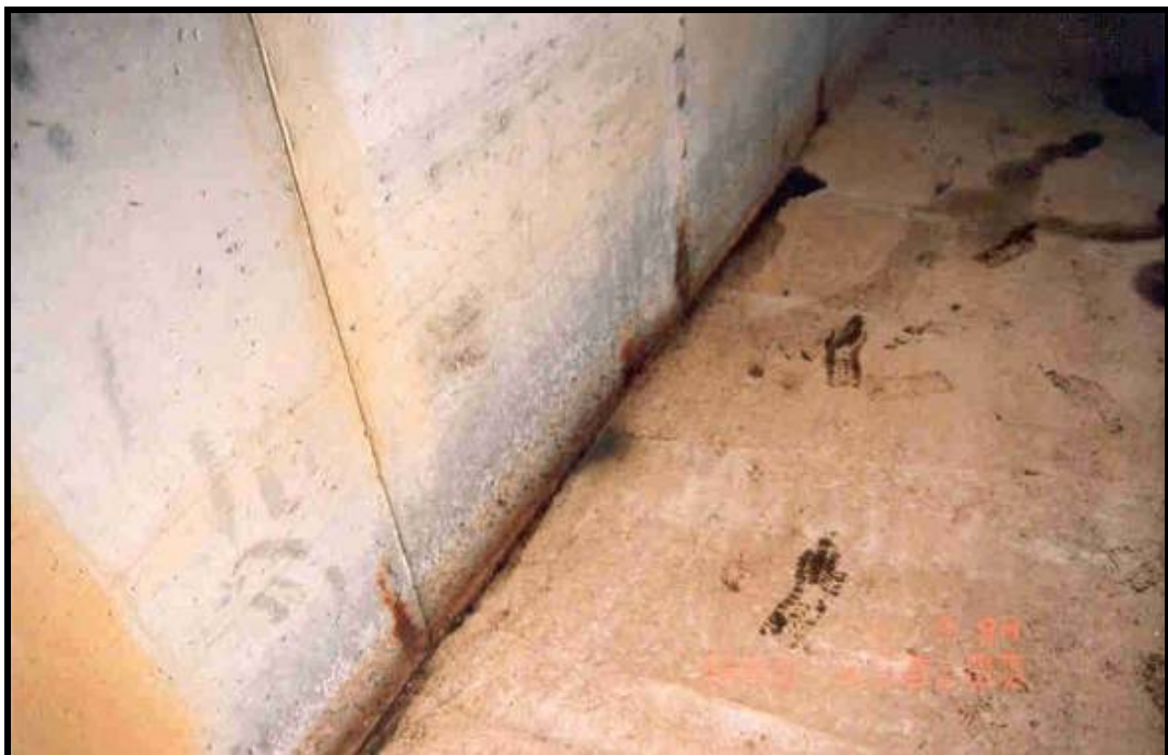
Photo 88 - PRECAST BOX UNIT RUST STAINING, BOTTOM CORNERS OF THE LEGS
