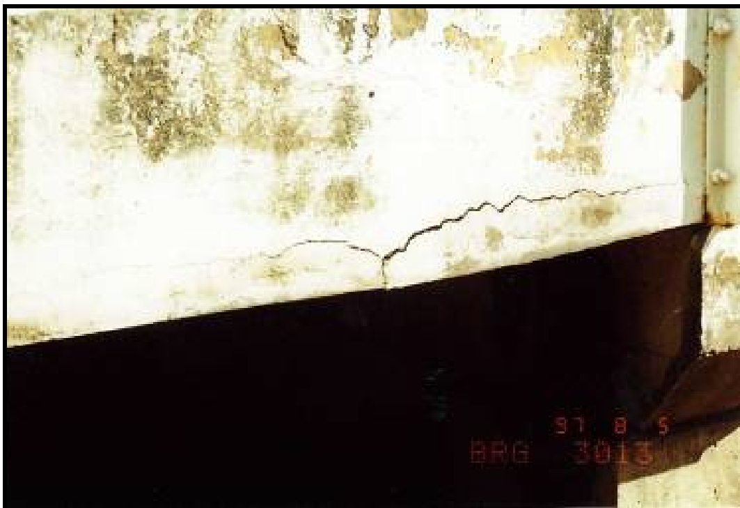
Photo 63 - HEAVY HORIZONTAL CRACK IN SIDE OF DECK
