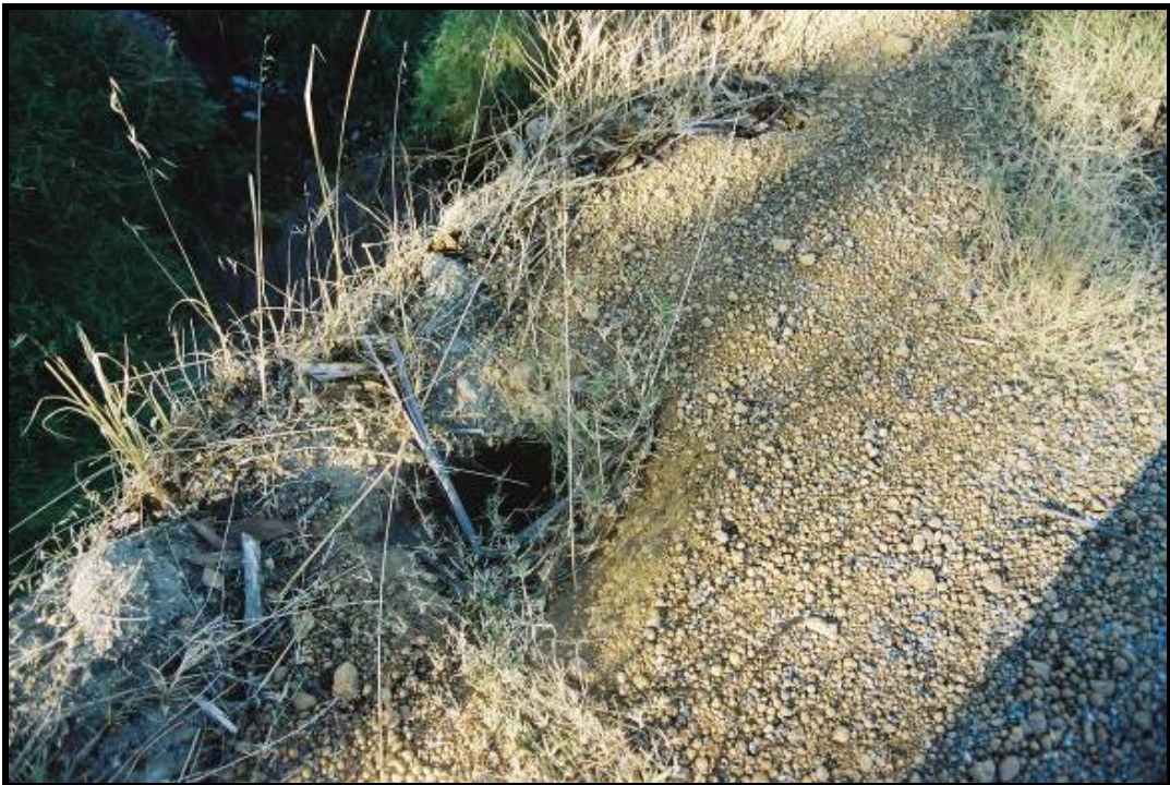
Photo 12 - HOLE IN ROAD SHOULDER
