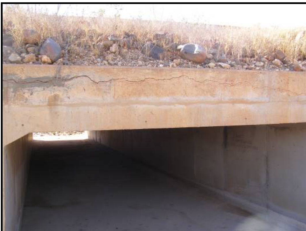
Photo No. 4: Headwall LHS, Heavy Crack over Barrel 3
