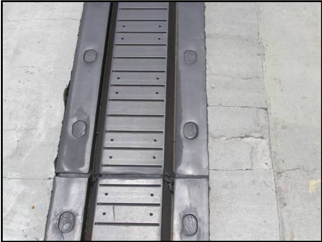
Photo 49 - CRACKS AND SPALLS TO CONCRETE AT DECK JOINT
