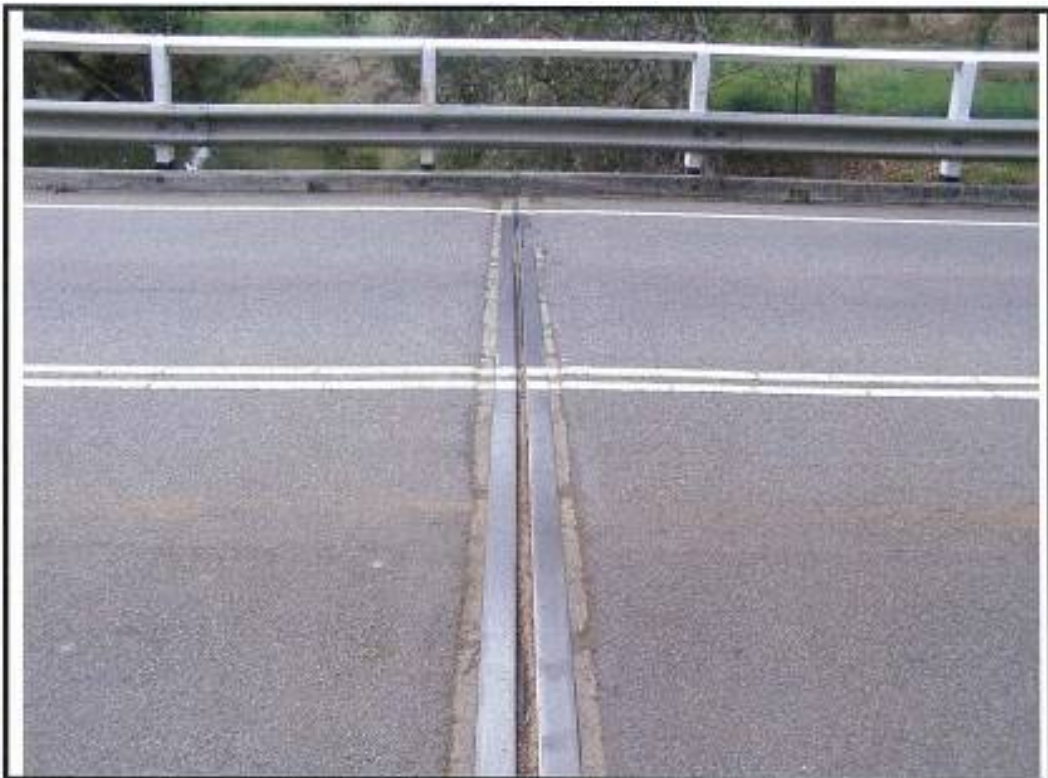
Photo No. 4: Centre Expansion Joint, Full of Debris
