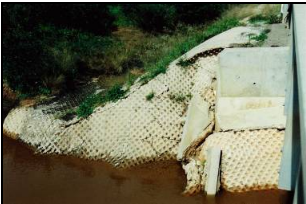
Photo 37 - REVETMENT MATTRESS DAMAGE AT ABUT 1 RHS
