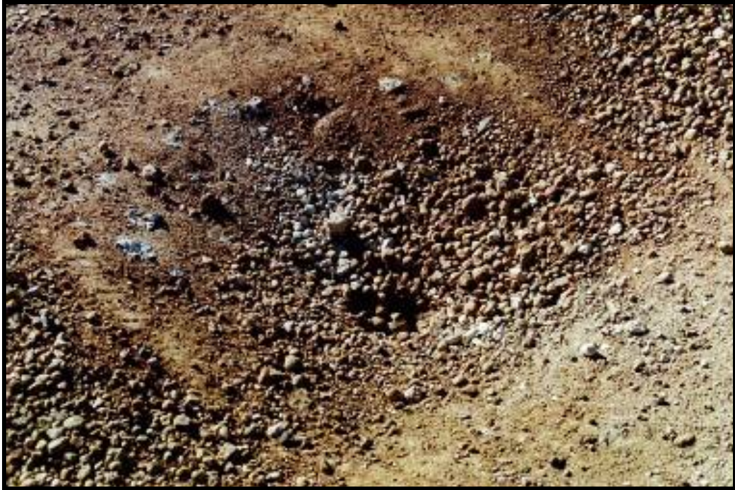
Photo 7 - POTHOLE IN GRAVEL ROAD SURFACE (Failed stringer and decking subsequently found underneath)
