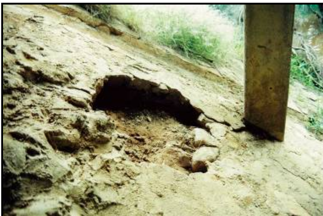
Photo 38 - SMALL SECTION OF STONE PITCHING MISSING AT ABUT 1
