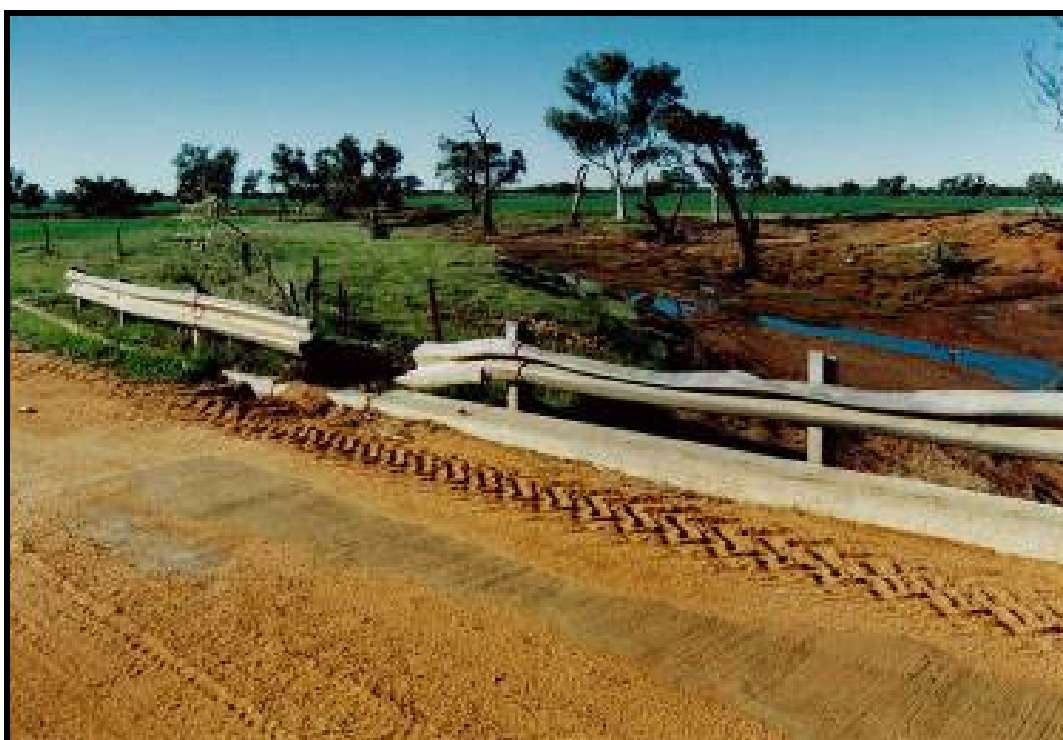
Photo 16 - IMPACT DAMAGE TO RHS GUARDRAIL
