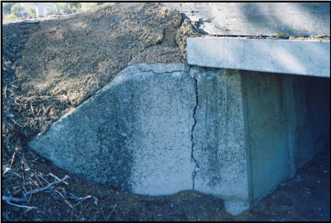
Photo 86 - PRECAST BOX UNIT WING WALL HAS HEAVY VERTICAL CRACK BUT APPEARS STABLE
