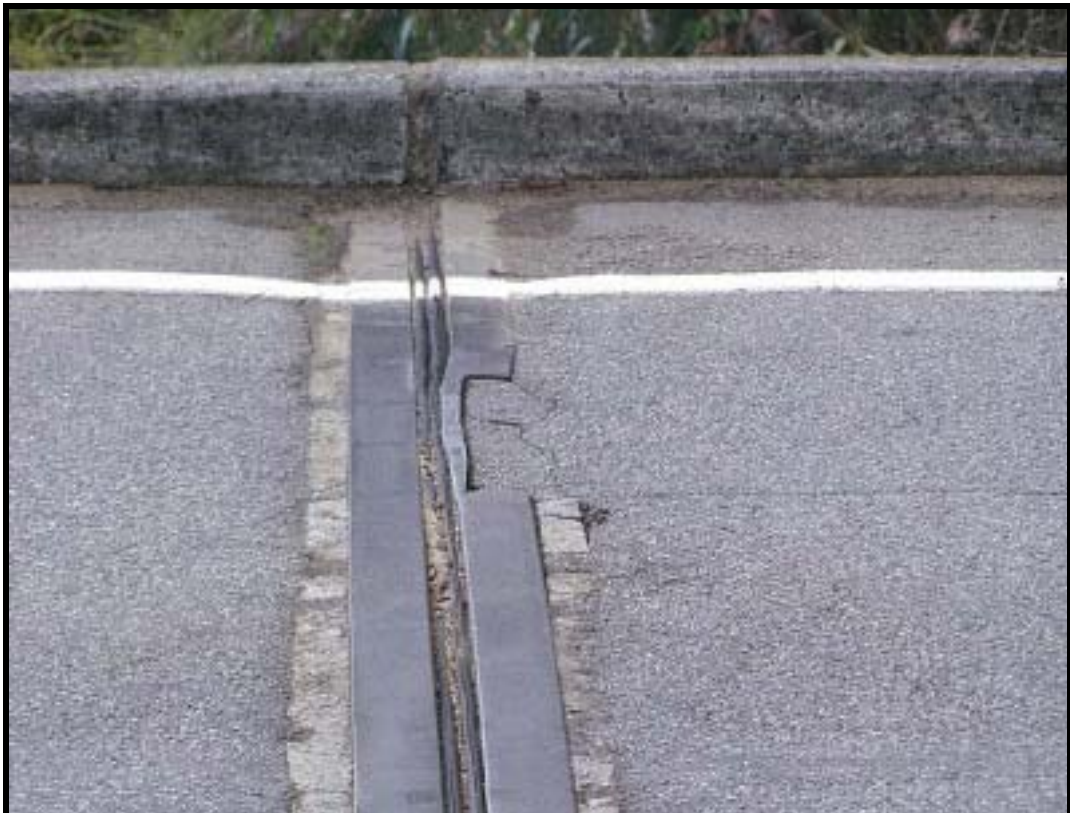
Photo 50 - DAMAGED SECTION OF STEEL ANGLE BEARINGS (TIMBER AND NON-TIMBER BRIDGES)
