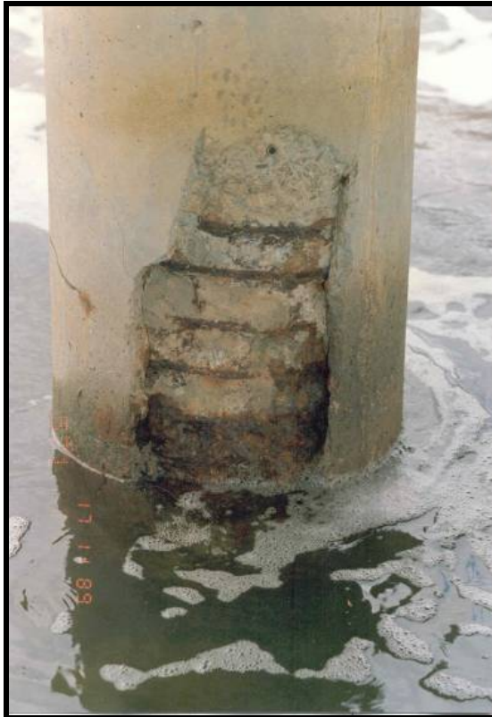
Photo 79 - CORROSION OF REINFORCEMENT ACCOMPANIED BY SPALLING
