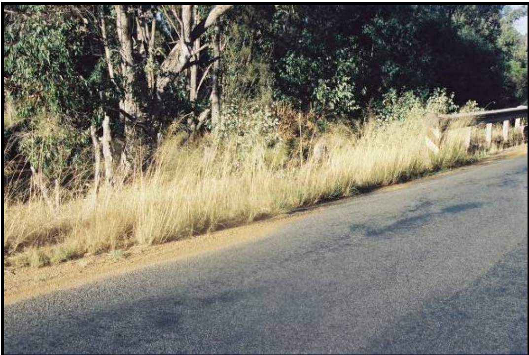
Photo 26 - EXCESSIVE VEGETATION GROWTH ALONG ROAD SHOULDER (Potential Fire Hazard)
