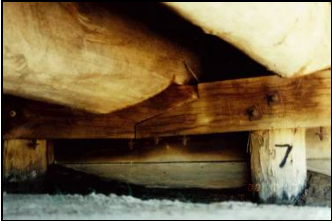
Photo 69 - HALFCAP BOWING AT JOINT LOCATION
