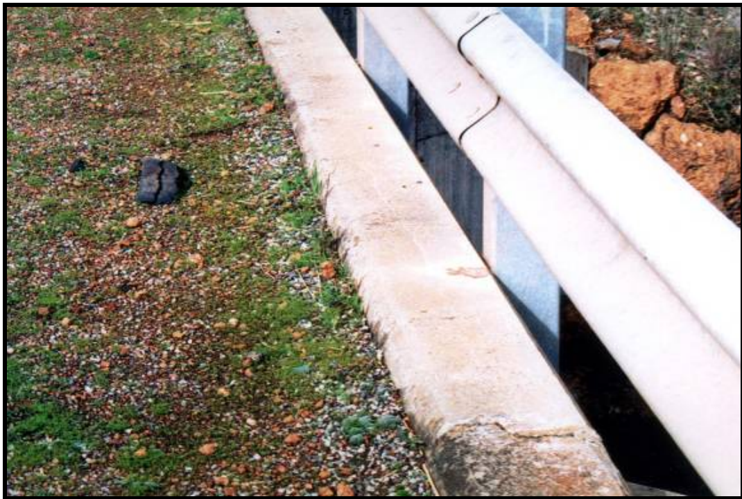
Photo 22 - SCUPPERS ARE BLOCKED BY EXCESSIVE ROAD DEBRIS
