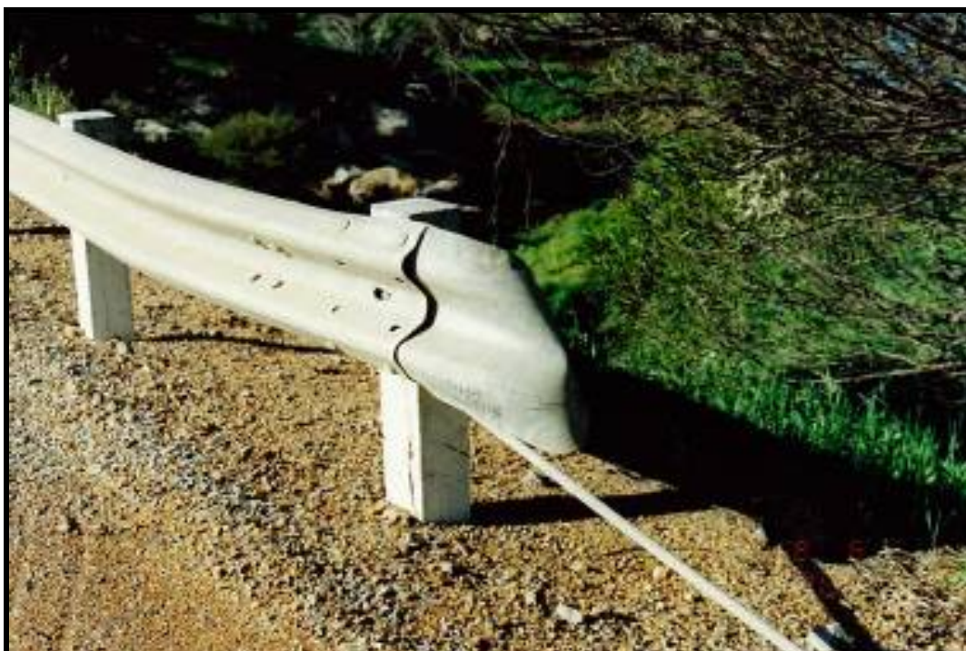
Photo 15 - DAMAGED FISHTAIL AT ABUT 1 RHS
