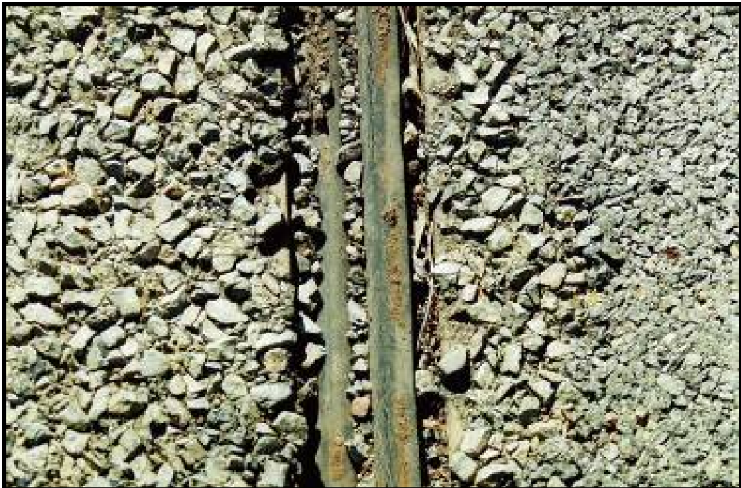
Photo 48 - CLOSE UP OF WABO JOINT
