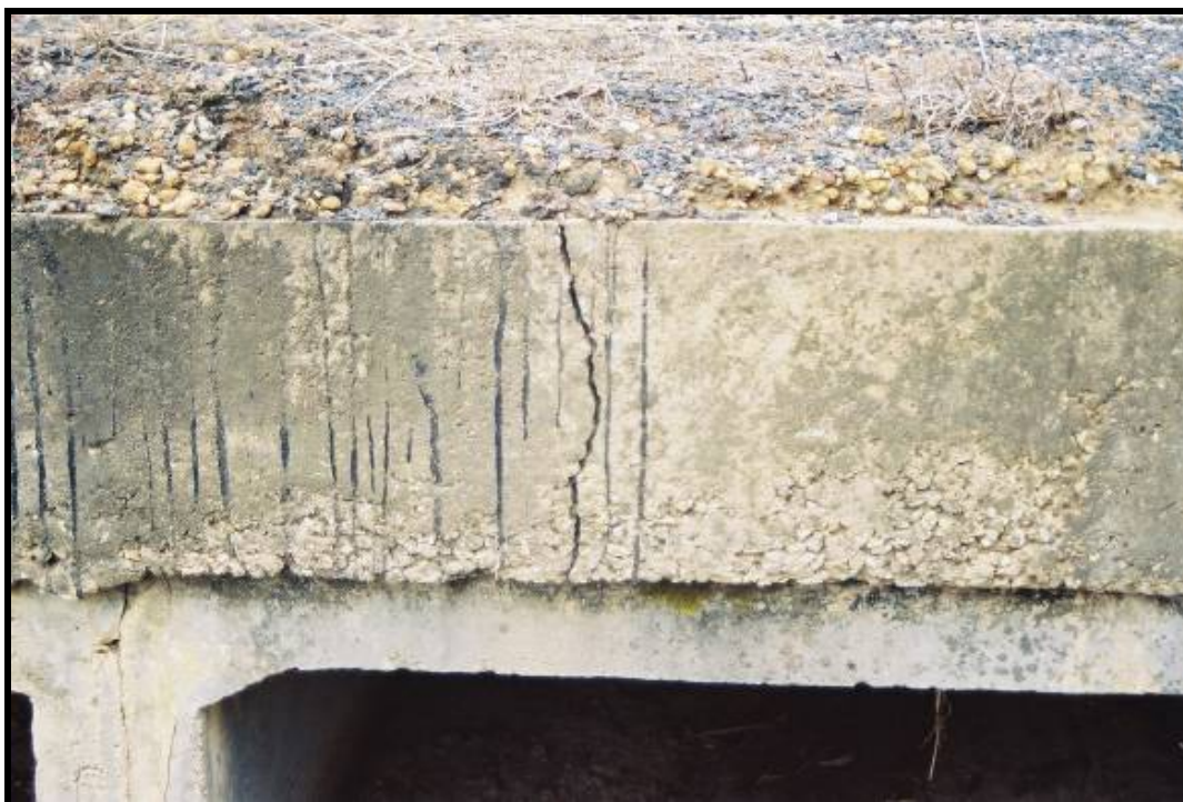
Photo 84 - PRECAST BOX UNIT HEADWALL HAS HONEYCOMBING, HEAVY CRACK
