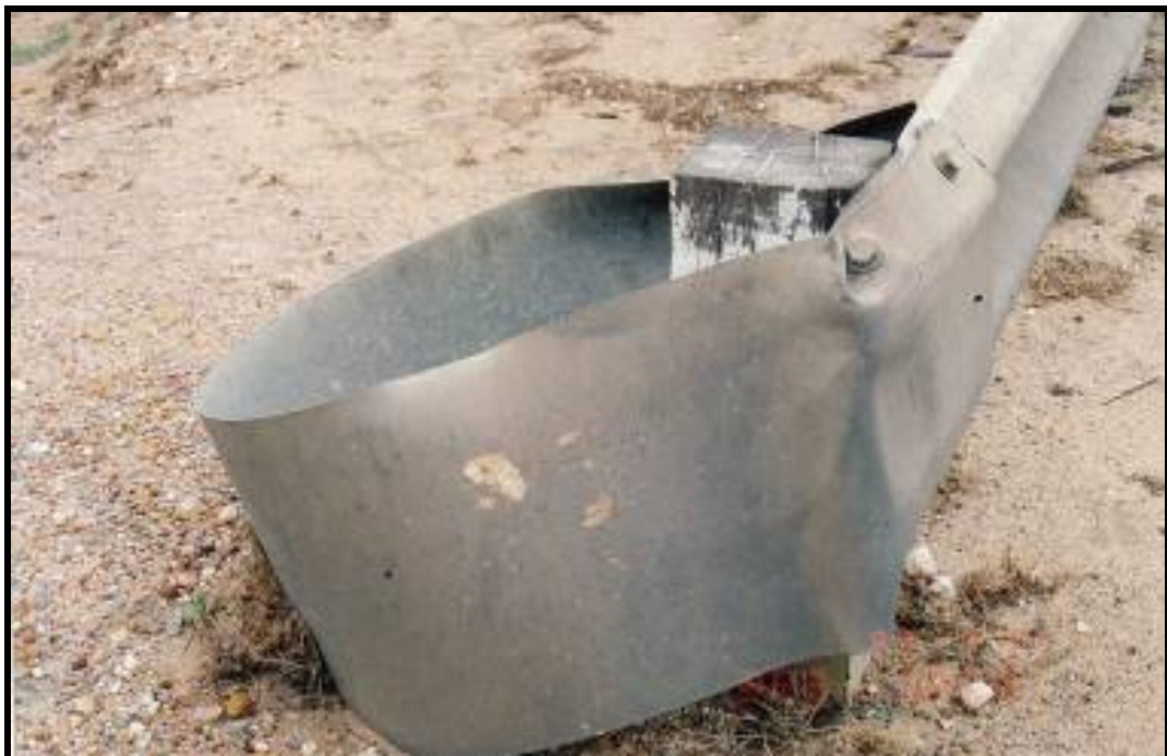
Photo 14 - IMPACT DAMAGE TO BULL NOSE
