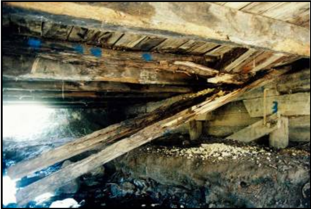
Photo 55 - FAILED STRINGER AND DECKING (Related to pothole shown at Photo 7)
