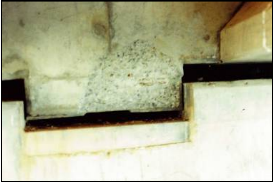
Photo 83 - SPALLED CONCRETE AT ABUT 1 SHEAR KEY
