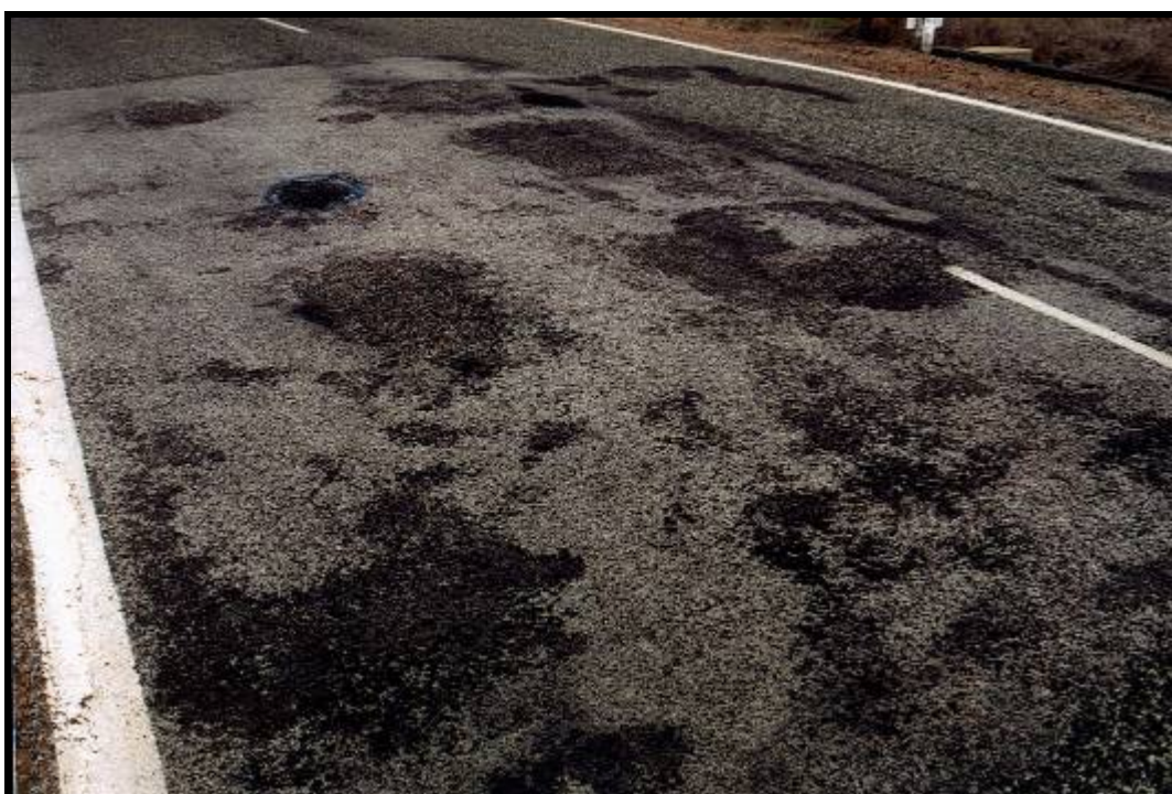
Photo 4 - POOR ROAD SURFACE, POTHOLE, BUMPS, CRACKS, WHEEL RUTS
