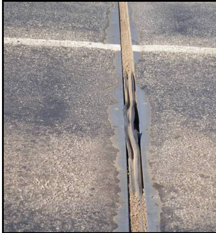
Photo 45 - DAMAGED SEAL IN DECK JOINT
