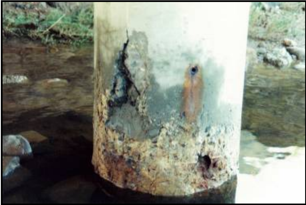
Photo 75 - BADLY DAMAGED COLUMN
