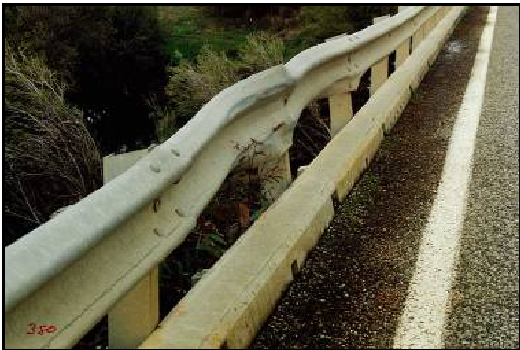
Photo 17 - IMPACT DAMAGE ALONG FLEX-BEAM
