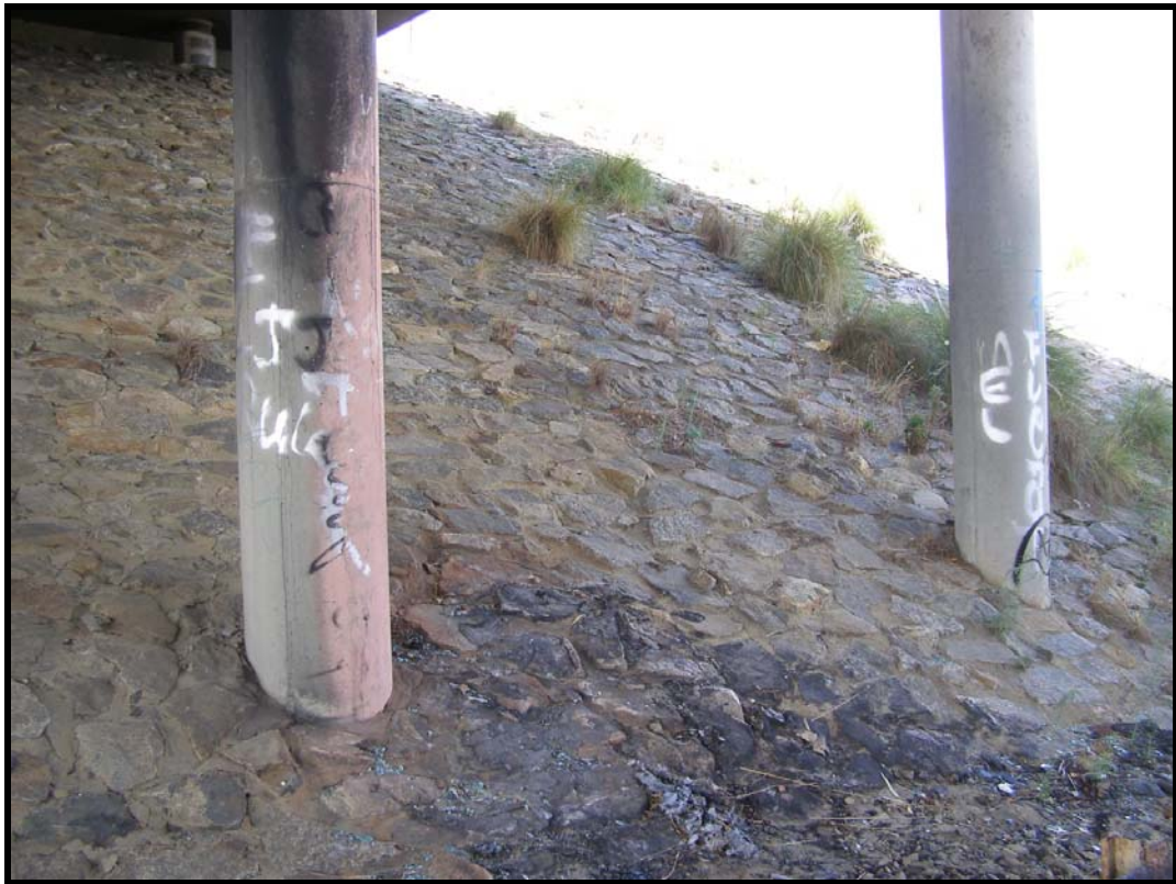
Photo 80 - FIRE DAMAGE TO CONCRETE COLUMN
