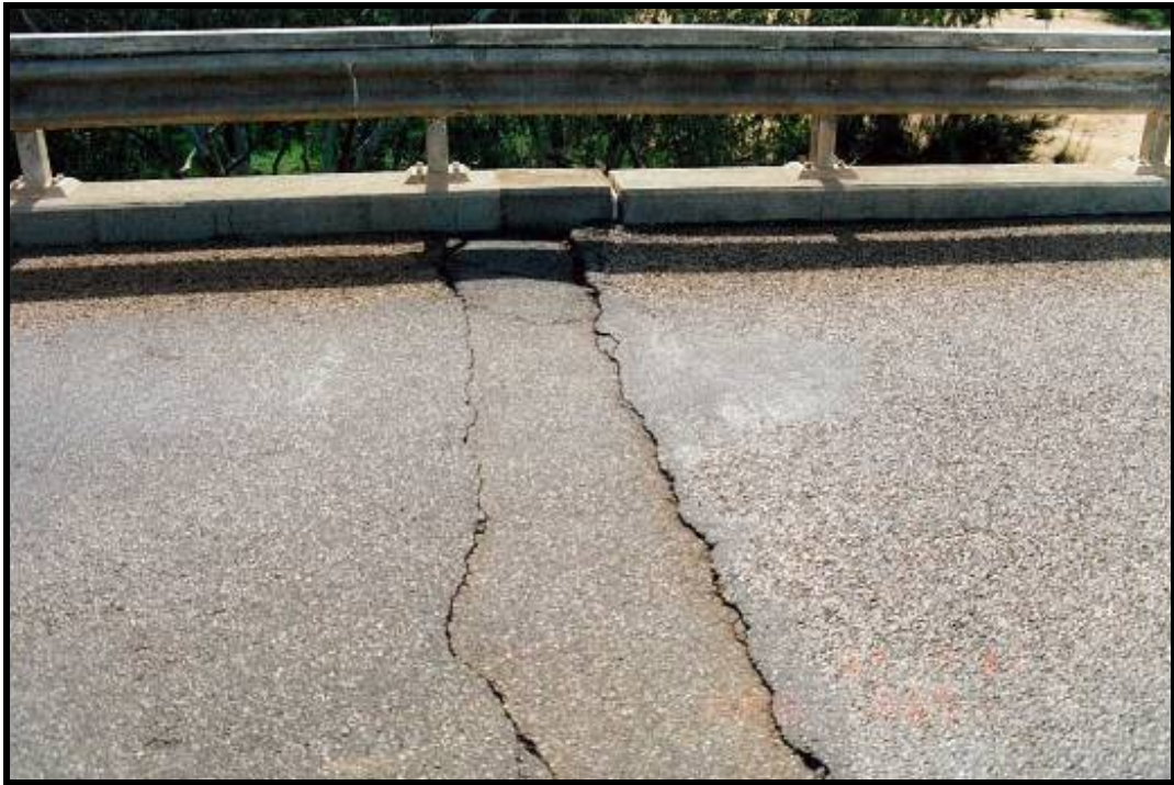
Photo 5 - CRACKS IN THE ROAD PAVEMENT AND SETTLEMENT AT THE ABUTMENT
