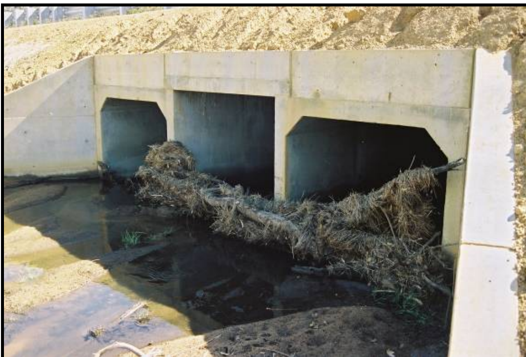
Photo 28 - PRECAST BOX UNITS HAVE A BUILD-UP OF BRANCHES AND WEEDS (This could cause future flow and/or scour problems)
