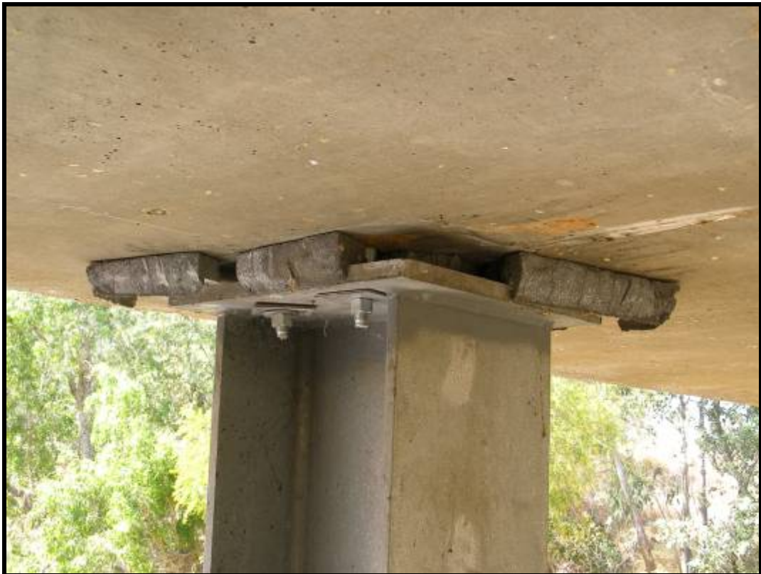
Photo 54 - PIER 3 COLUMN 1, DRY PACK BREAKING UP SUPERSTRUCTURE (TIMBER BRIDGES)
