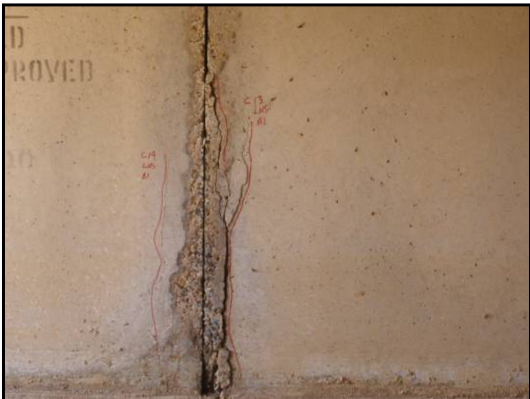
Photo 90 - HEAVY VERTICAL CRACKS IN BARREL 1, UNITS 13 AND 14
