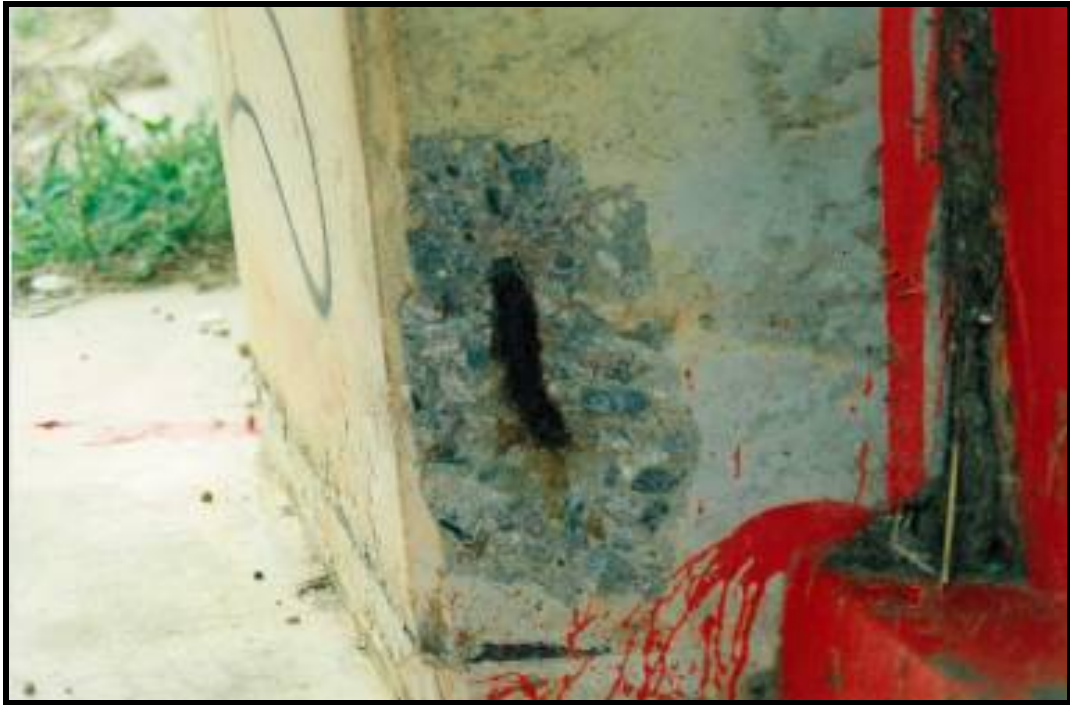
Photo 77 - SPALLED CONCRETE & EXPOSED REINFORCEMENT, PIER 2, COLUMN 1
