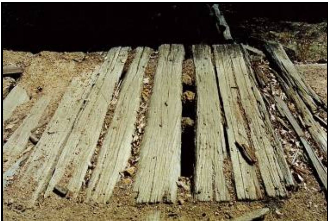
Photo 56 - DECK PLANKS IN VERY POOR CONDITION
