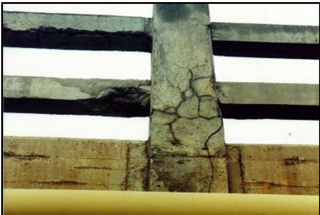
Photo 18 - ADVANCED ASR CRACKING IN POSTS AND RAILS
