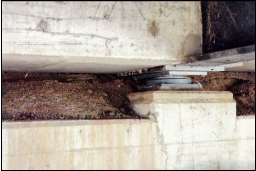
Photo 51 - BUILD-UP OF DEBRIS AROUND THE BEARING
