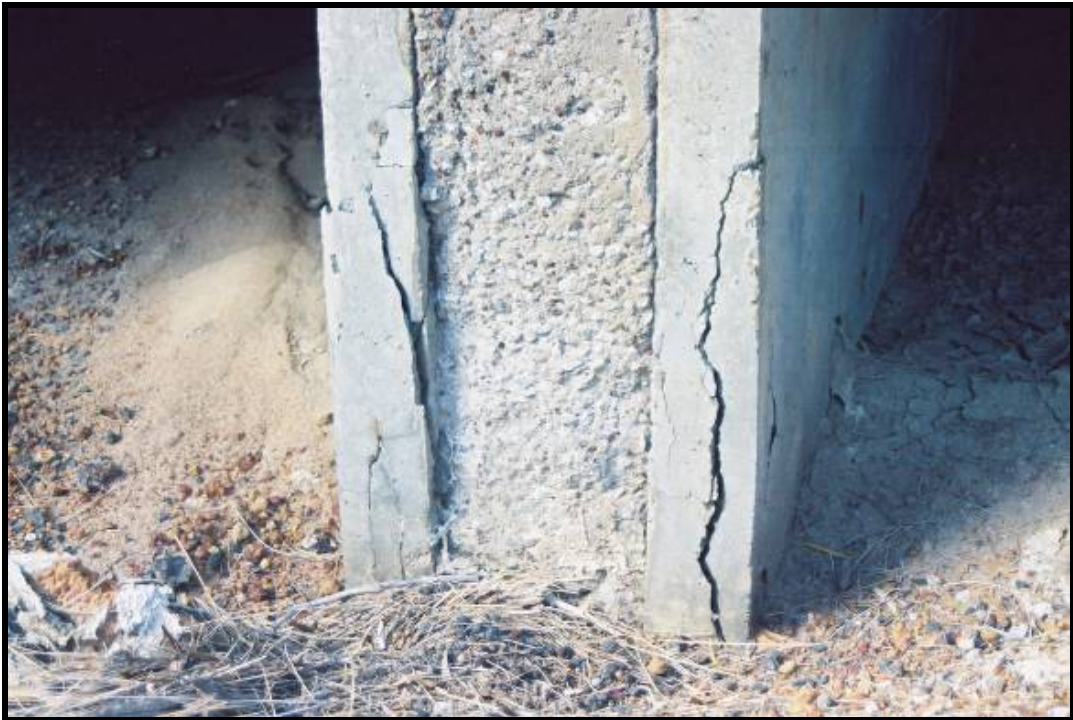
Photo 89 - PRECAST BOX UNIT OUTSIDE LEGS HAVE HEAVY CRACKING CAUSED BY CORRODED REINFORCEMENT
