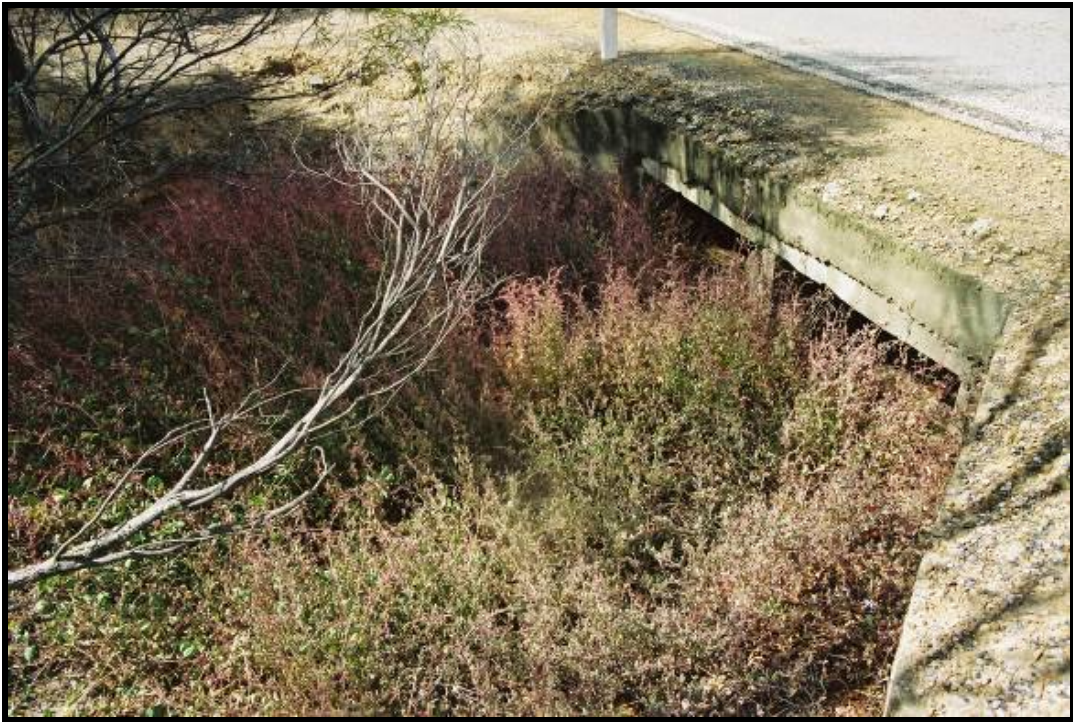
Photo 25 - BRIDGE OPENING IS BLOCKED BY HEAVY VEGETATION
