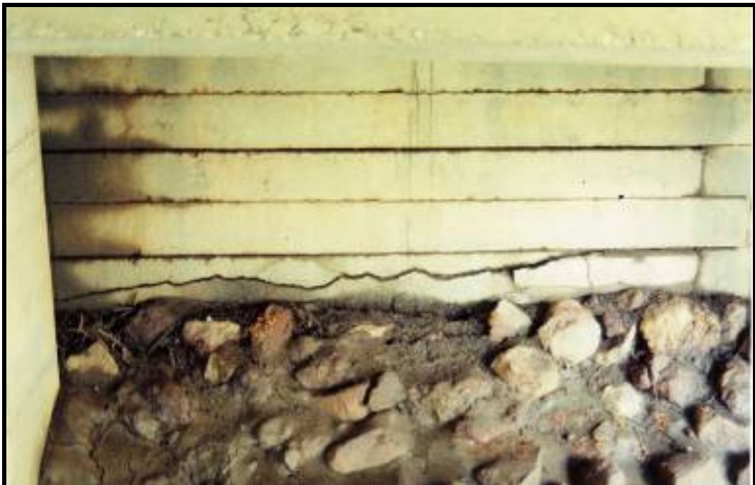
Photo 82 - HEAVILY CRACKED ABUTMENT CRIB WALL PANEL
