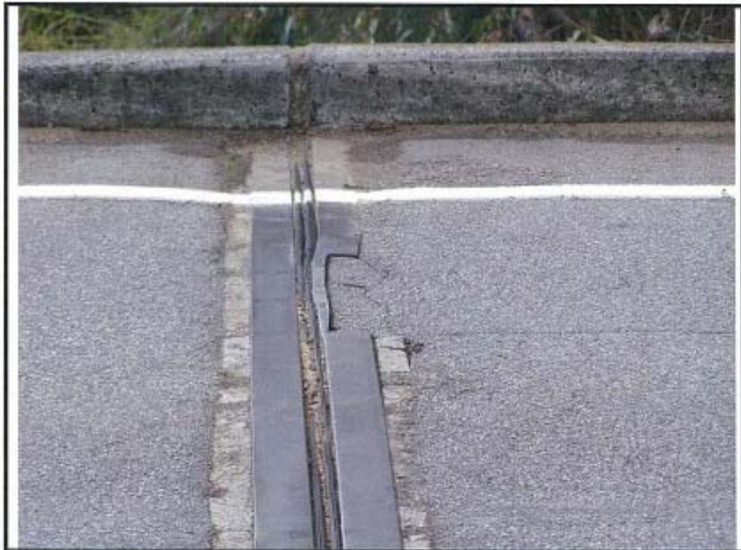
Photo No. 6: Damaged Section of Steel Angle near LHS
