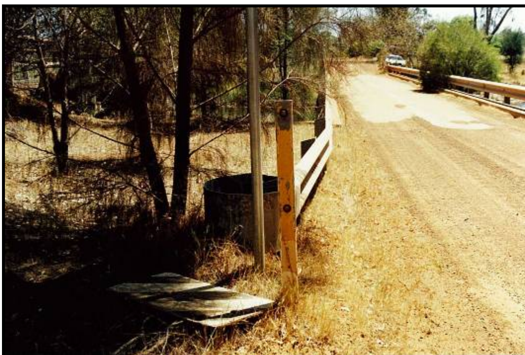
Photo 3 - WIDTH MARKER BROKEN OFF POST
