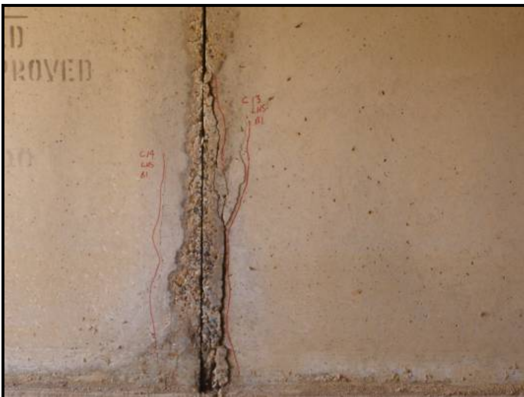
Photo No. 10: Heavy Vertical Cracks in Barrel 1, Units 13 and 14
