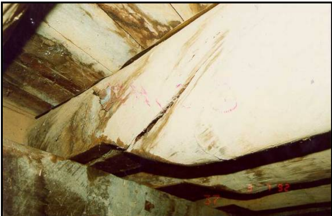
Photo 60 - TWISTING SPLIT IN STRINGER
