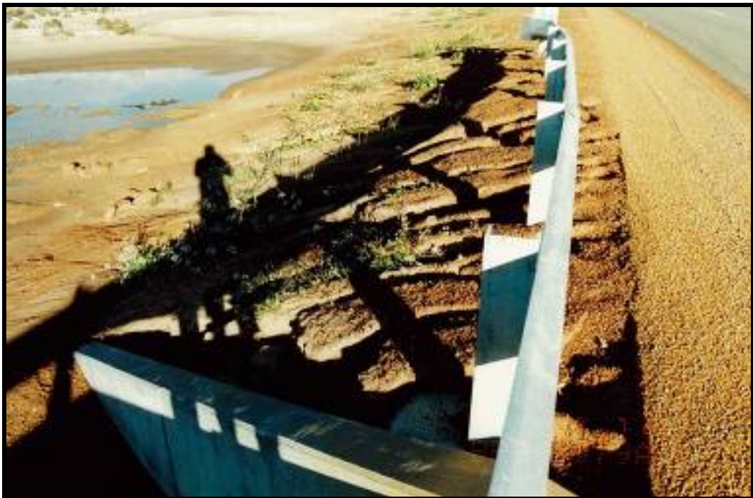
Photo 32 - EMBANKMENT EROSION
