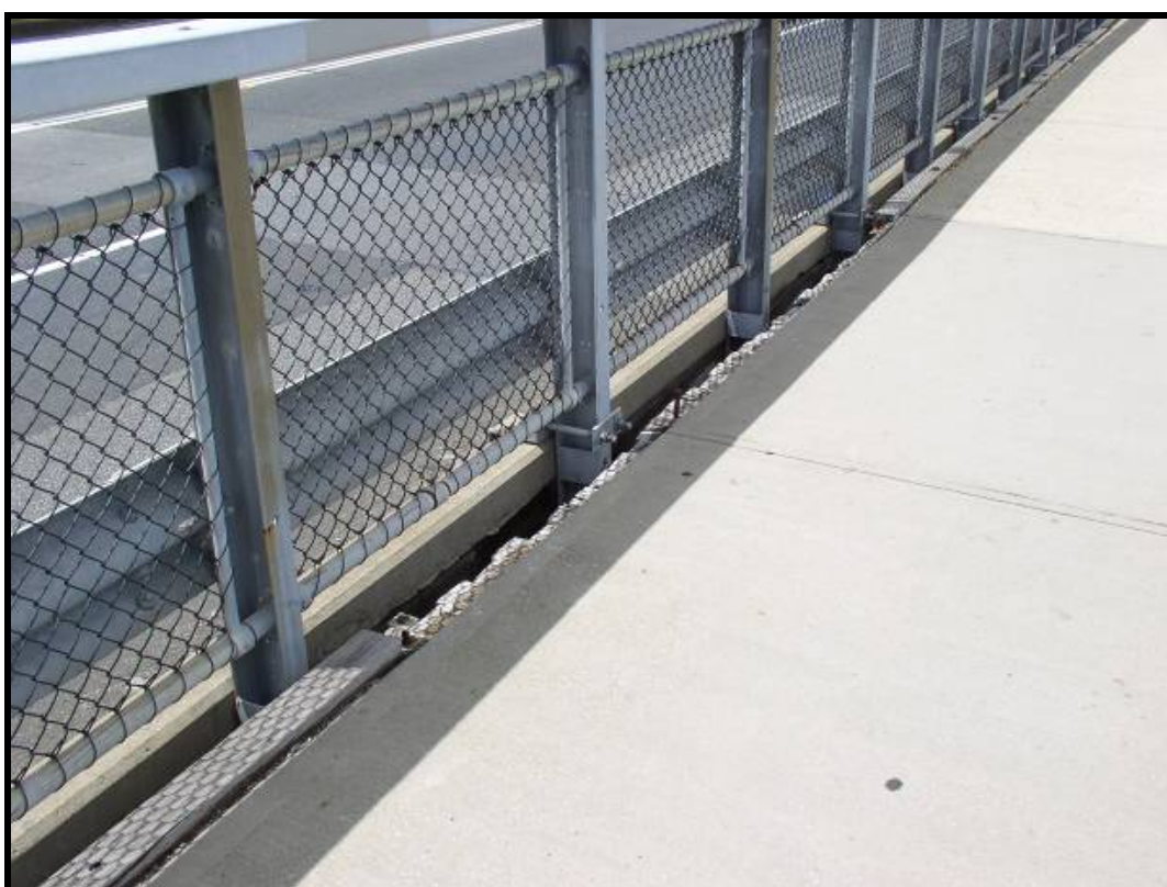
Photo 44 - LHS KERB OF FOOTPATH MISSING OVER SPAN 28 EXPANSION JOINTS AND DECK JOINTS (TIMBER AND NON-TIMBER BRIDGES)
