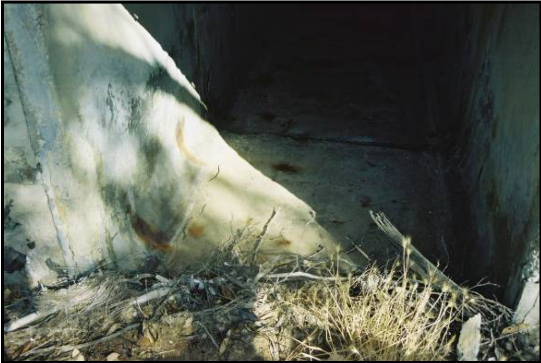
Photo 87 - PRECAST BOX UNIT MEDIUM CRACKING AND RUST STAINING IN THE BASE SLAB
