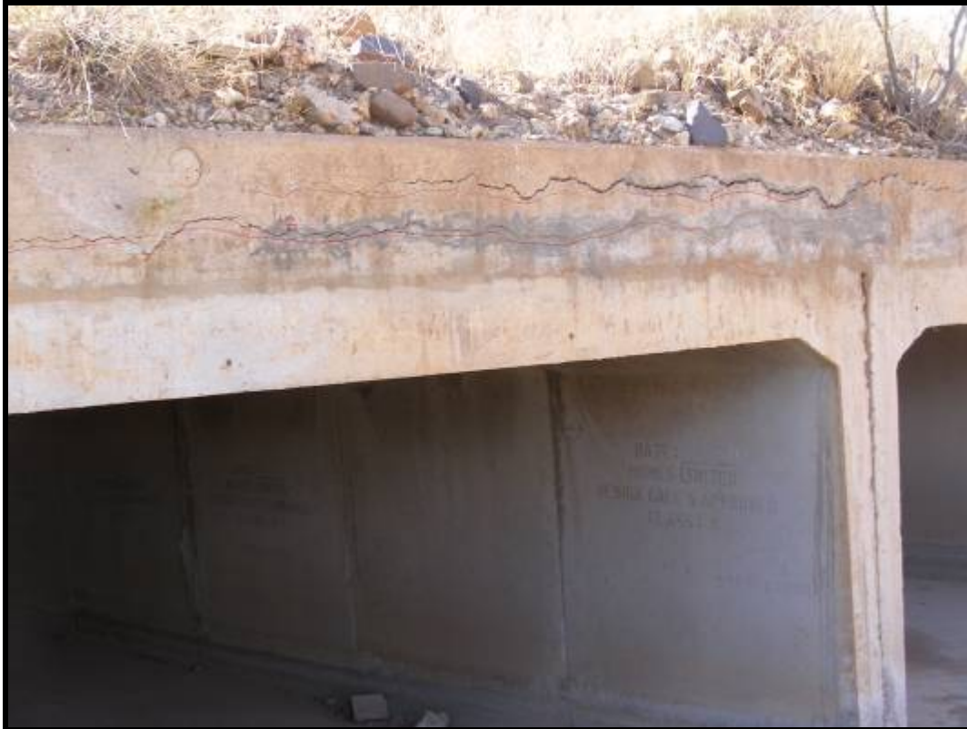
Photo No. 3: Headwall LHS, Heavy Cracks over Barrels 1 and 2
