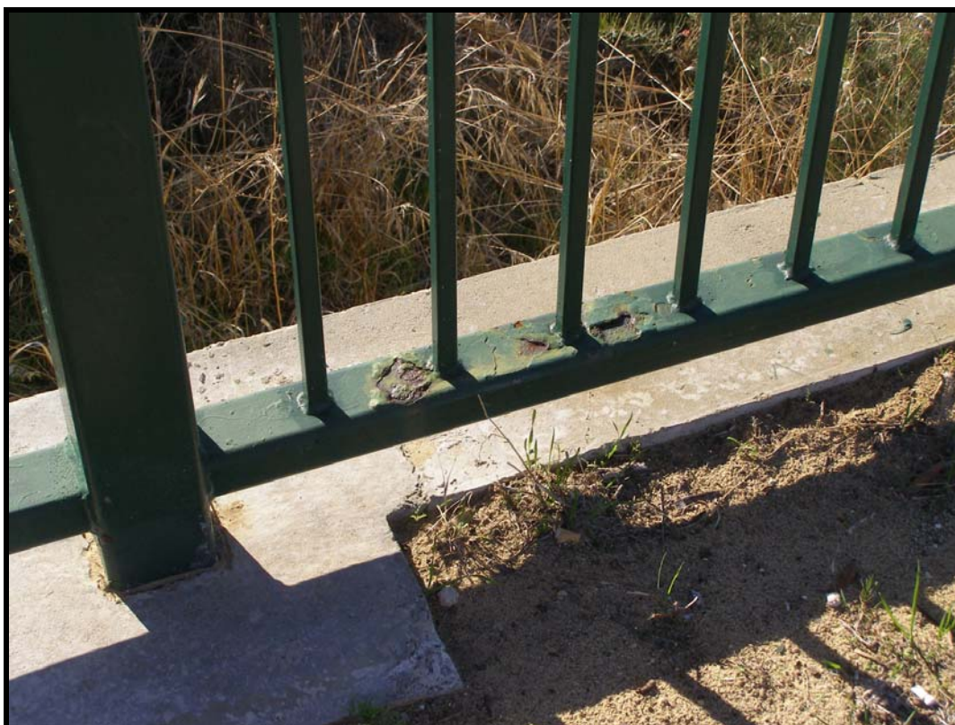
Photo 43 - CORROSION OF PEDESTRIAN BARRIER
