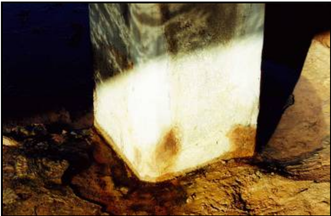
Photo 78 - MEDIUM CRACKS AND RUST STAINING TO BOTTOM OF PILE
