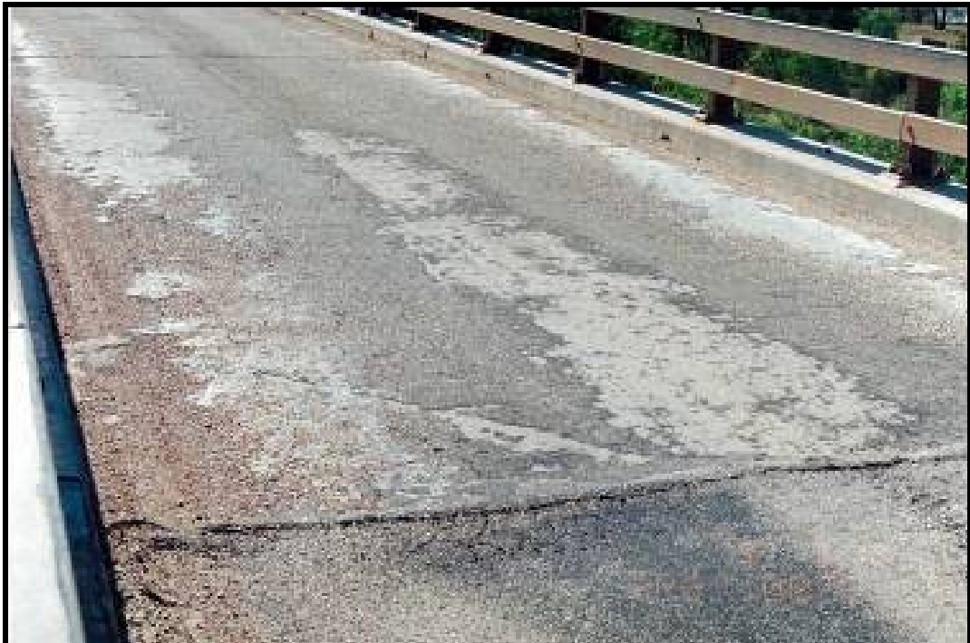
Photo 6 - STRIPPING OF SEAL SURFACE AND SETTLEMENT AT THE ABUTMENT
