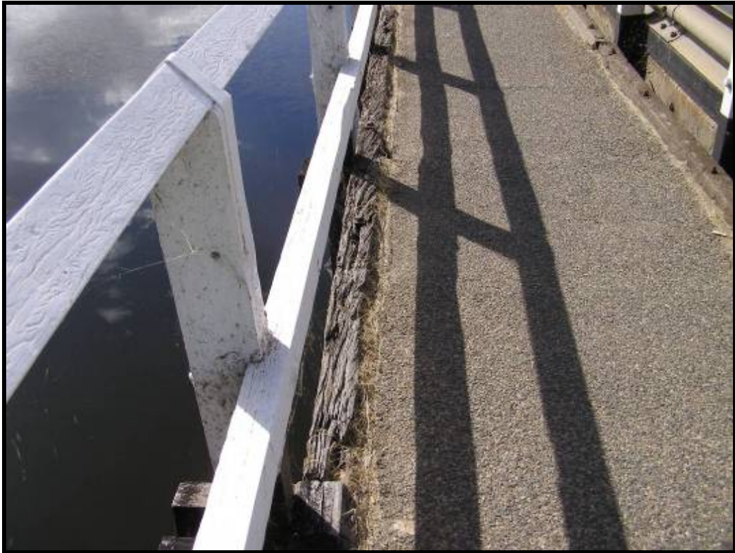
Photo 41 - TYPICAL POOR CONDITION OF TIMBER KERB, LHS OF FOOTPATH
