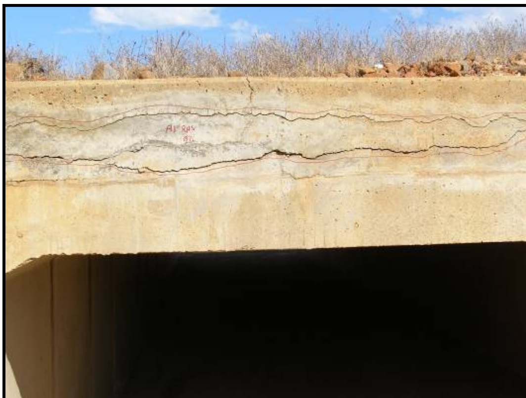
Photo No. 6: Headwall RHS, Heavy Cracks over Barrel 1
