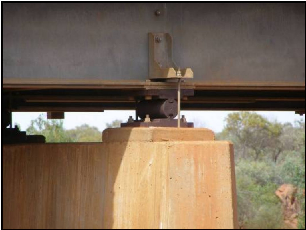
Photo 52 - CORRODED ROCKER BEARING
