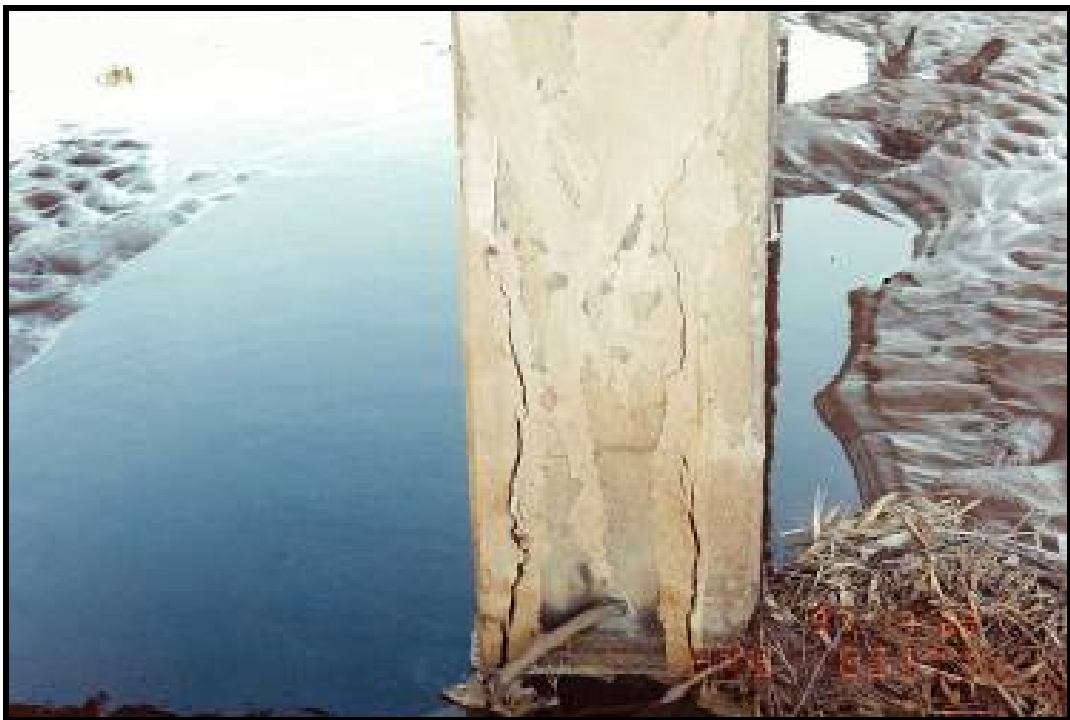
Photo 76 - HEAVY CRACKING FROM STEEL CORROSION, PIER 3, PILE 4
