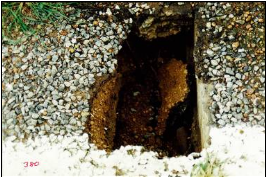
Photo 24 - LARGE HOLE IN ROAD APPROACH CAUSED BY POOR ROAD DRAINAGE
