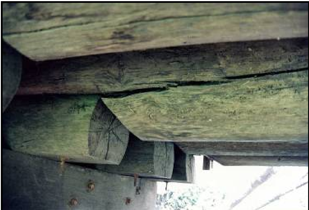
Photo 58 - LARGE HORIZONTAL SPLIT IN STRINGER
