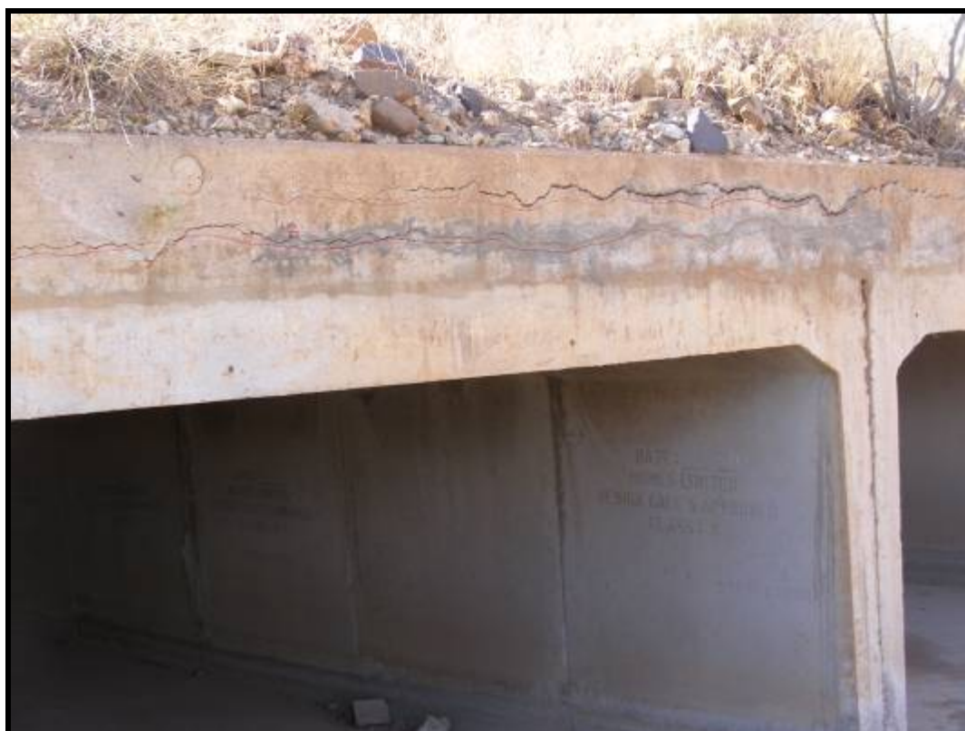
Photo 85 - HEADWALL LHS, HEAVY CRACKS OVER BARRELS 1 AND 2
