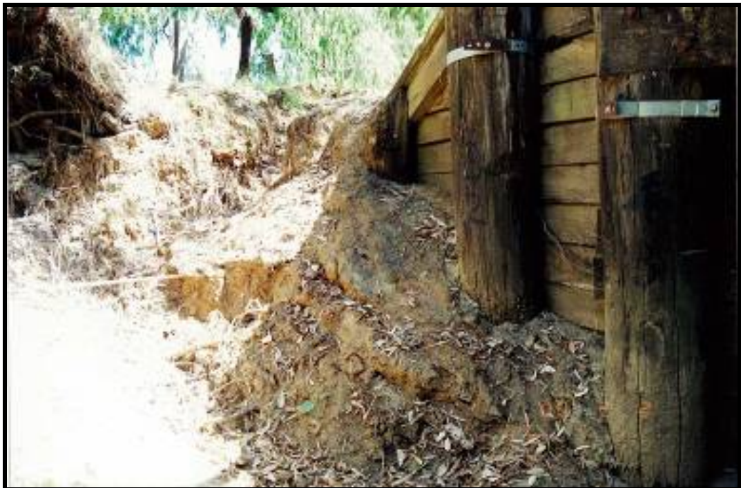
Photo 34 - SCOUR NEAR ABUTMENT WING WALL
