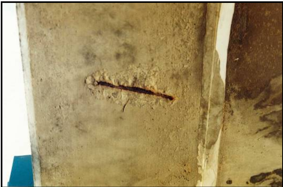
Photo 66 - EXPOSED REINFORCEMENT IN SOFFIT NEAR PIER, LHS (No change since previous inspection)
