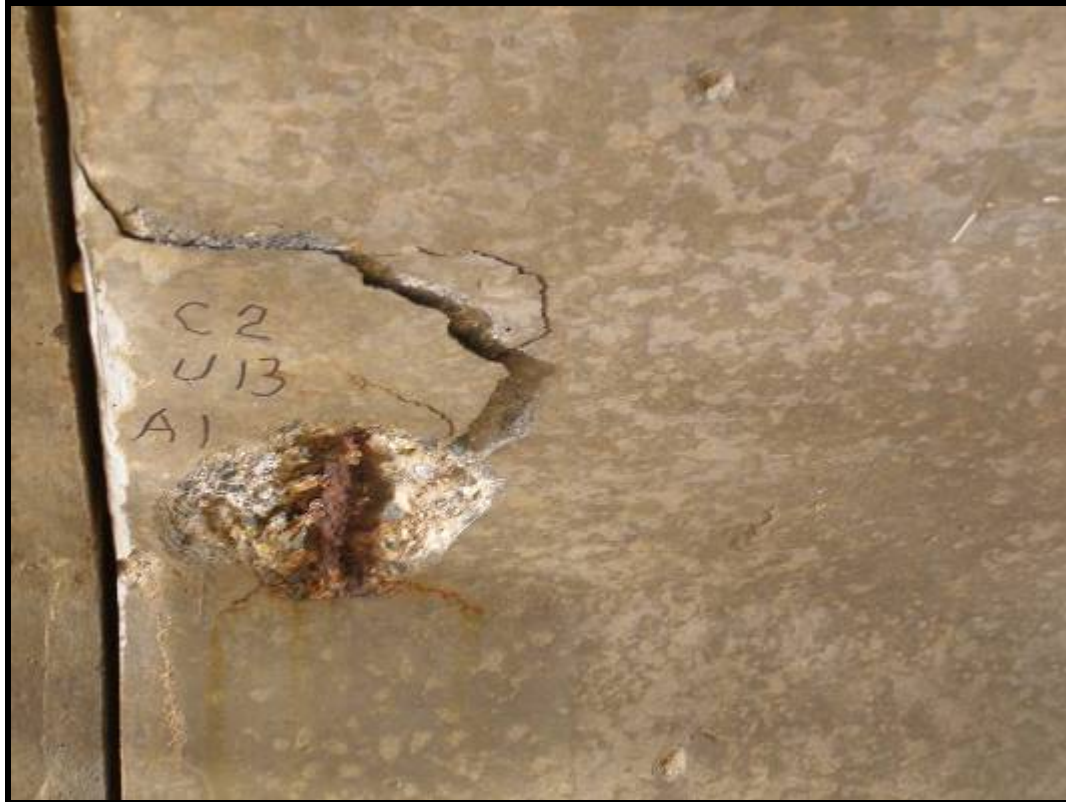
Photo No. 11: Spalled Concrete, Corroded Reinforcement, Barrel 3, Unit 2
