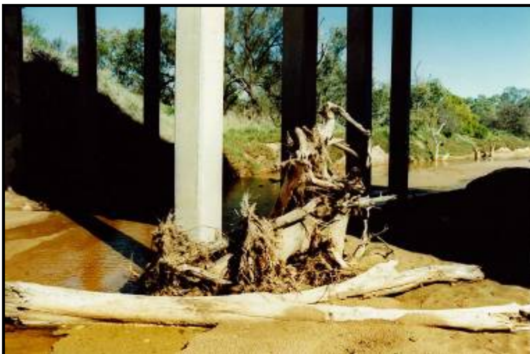
Photo 30 - DEBRIS BUILD-UP AROUND PIER 3
