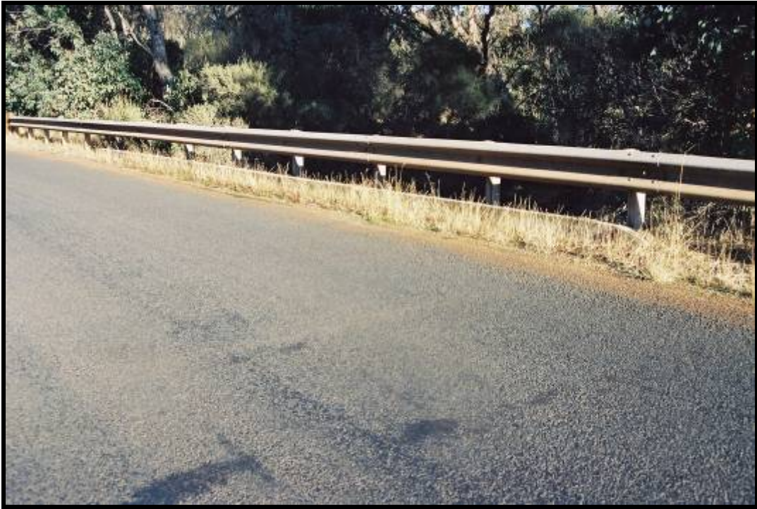
Photo 21 - VEGETATION REQUIRES CLEARING TO ENABLE SCUPPERS TO FUNCTION
