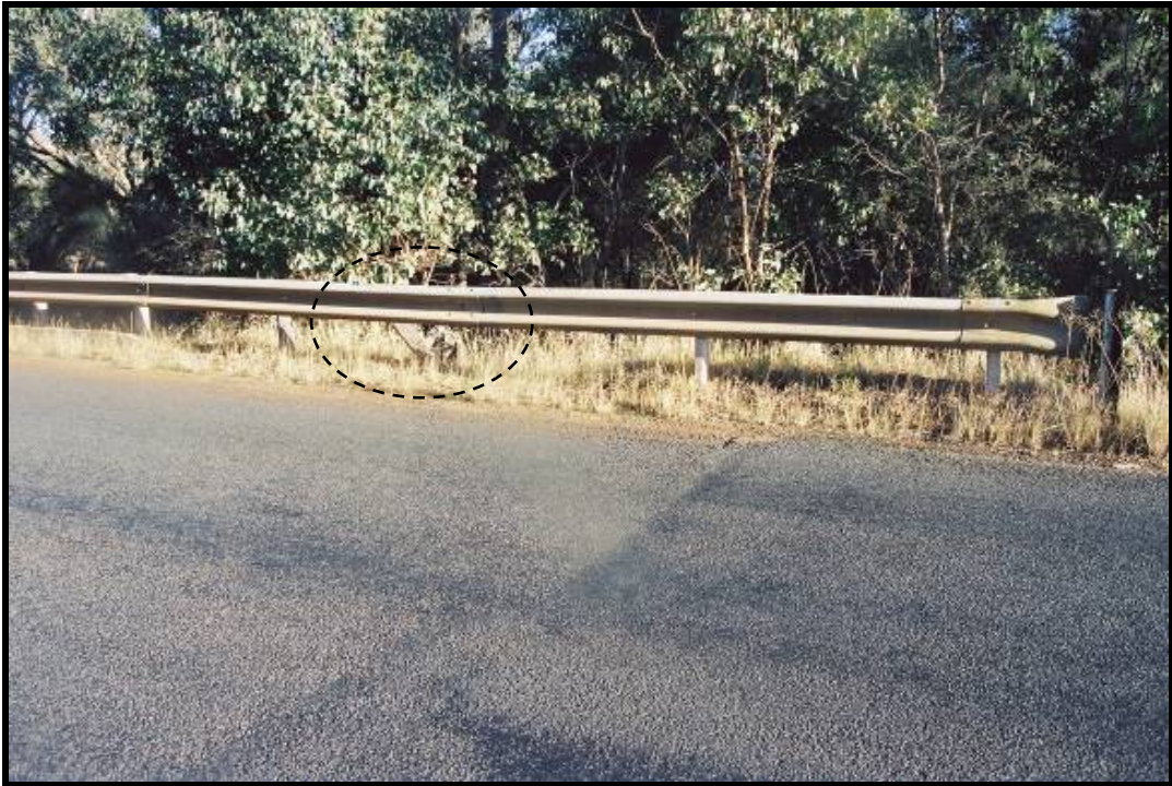
Photo 13 - DEPARTURE RAILING HAS BROKEN POSTS
