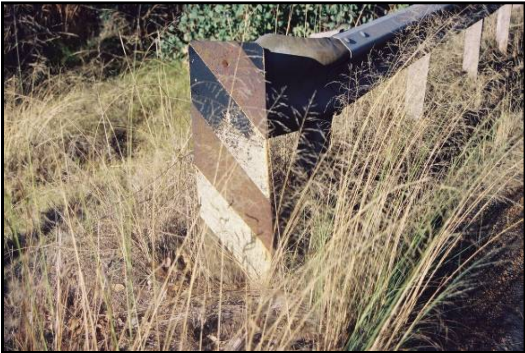
Photo 2 - WIDTH MARKER HAS LOST ITS REFLECTIVITY AND IS CONCEALED BY HIGH GRASS GROWTH
