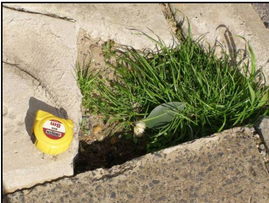
Photo 39 - HOLE IN FOOTPATH AT ABUTMENT 2
