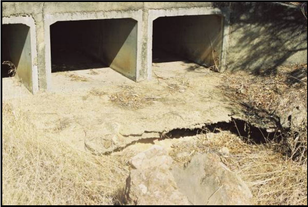
Photo 33 - SEVERE SCOURING UNDER THE INLET APRON
