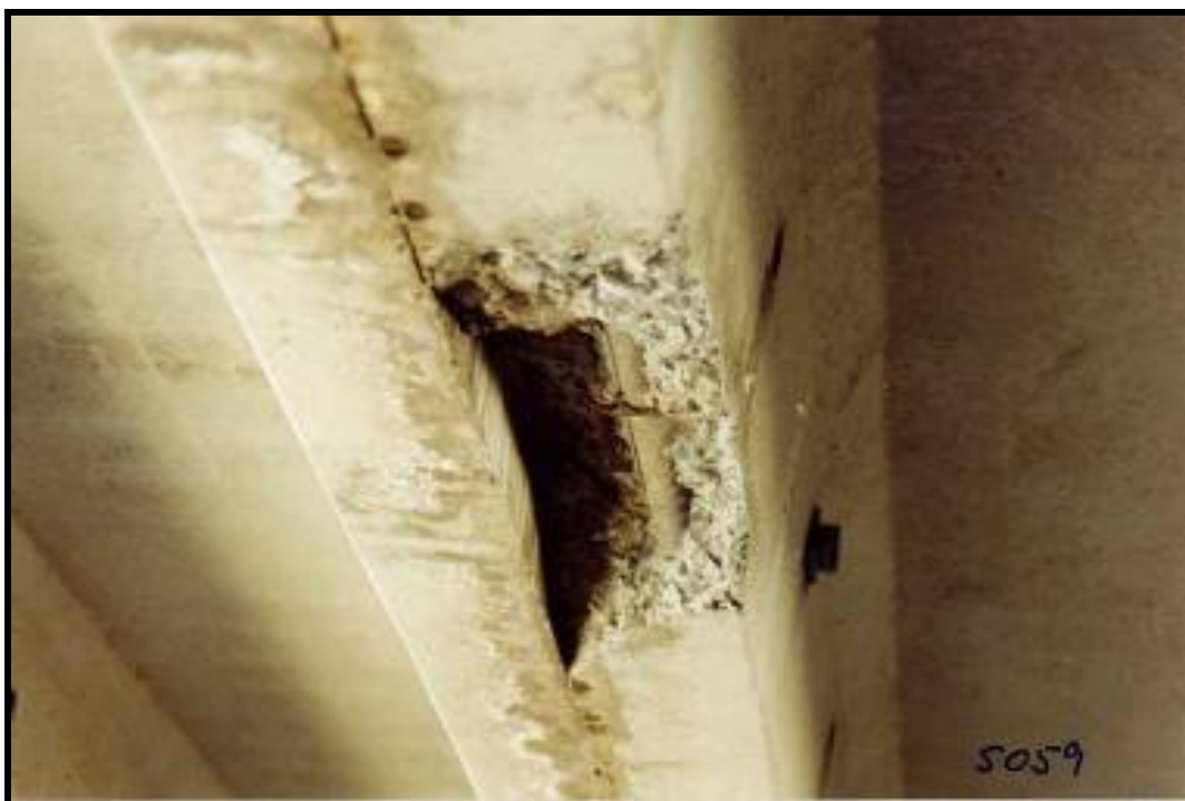
Photo 62 - DAMAGED U-BEAM LEG, EXPOSING REINFORCEMENT
