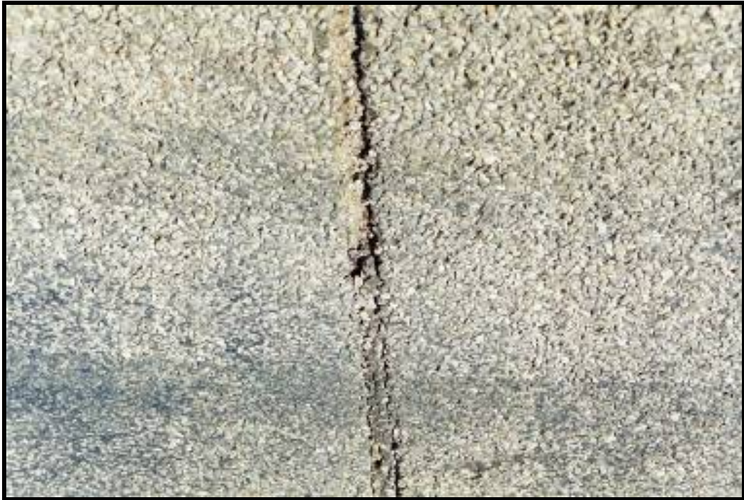
Photo 47 - WABO JOINT FILLED WITH ROAD SEAL
