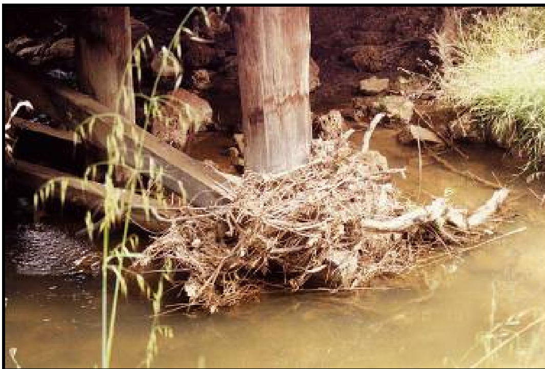
Photo 29 - DEBRIS BUILD-UP AROUND A TIMBER PIER PILE
