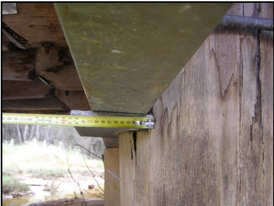
Photo 68 - HALFCAP SEATING STARTING TO SHOW SIGNS OF DISTRESS
