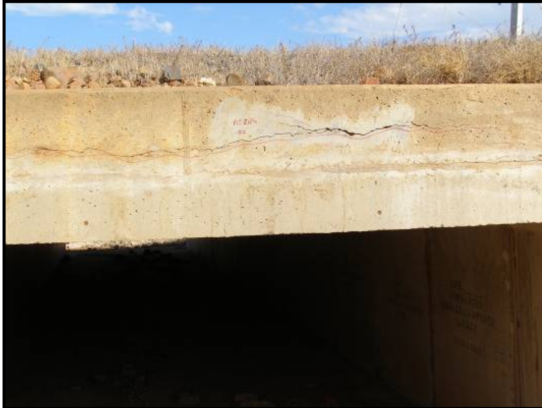
Photo No. 7: Headwall RHS, Heavy Cracks over Barrel 3
