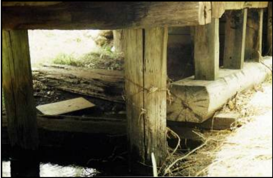
Photo 71 - LARGE VERTICAL SPLIT IN PILE
