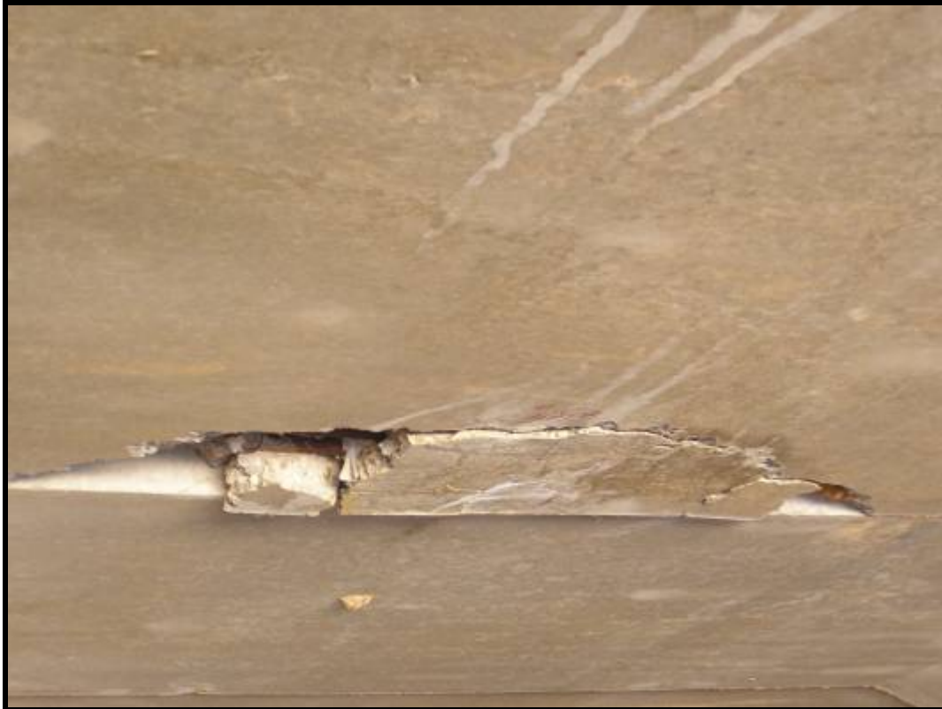
Photo No. 9: Concrete Spall and Exposed Reinforcement, Barrel 1, Unit 4
