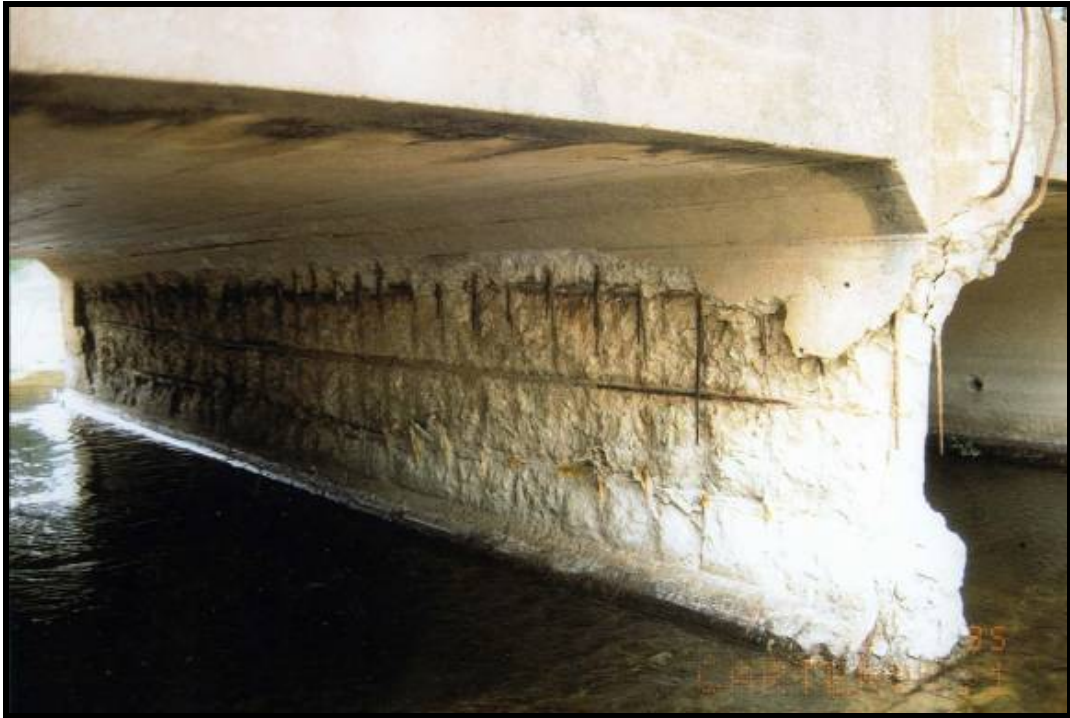
Photo 81 - BADLY ERODED CONCRETE WALL PIER
