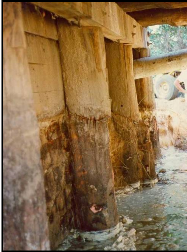
Photo 35 - SCOUR OF ABUTMENT PILES
