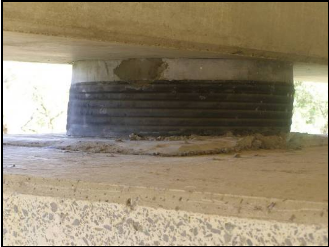
Photo 53 - SLIGHT BULGING OF ELASTOMERIC BEARING
