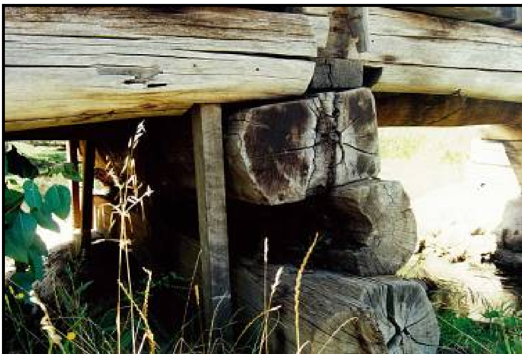
Photo 73 - FAILURE OF BEDLOG 2
