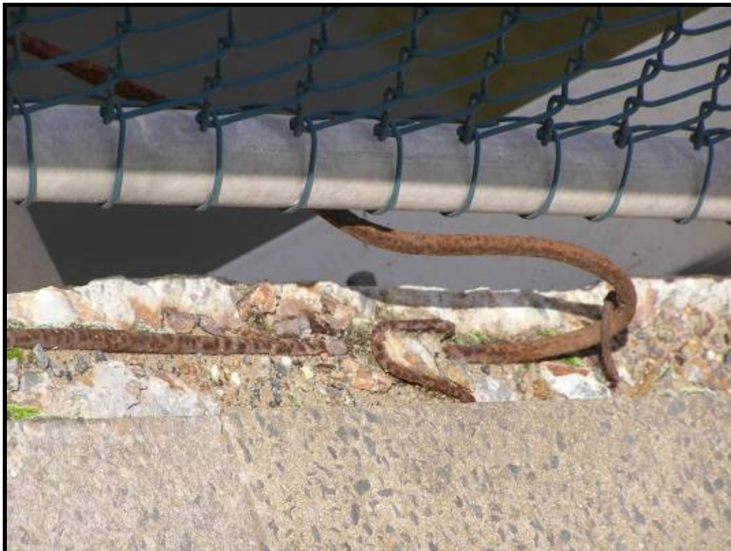
Photo 40 - TYPICAL POOR CONDITION OF CONCRETE KERB, LHS OF FOOTPATH
