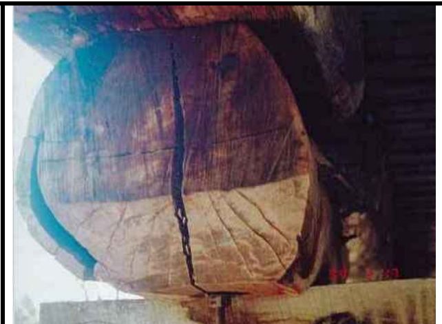
Photo 112 - Shows large vertical split and sap layer separating at corbel end
