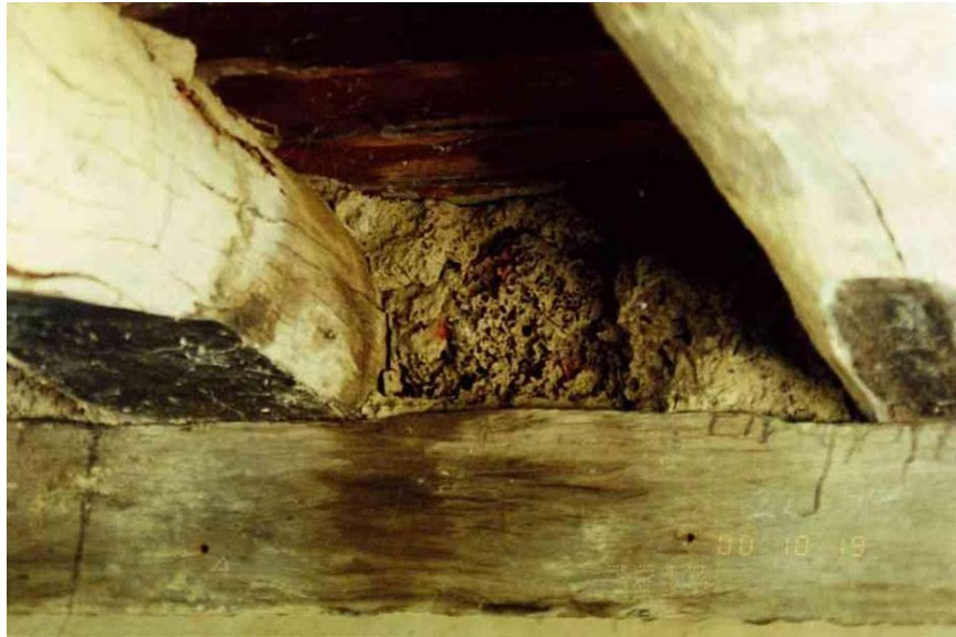
Figure 10.1 - EXAMPLE OF INSECT INFESTATION IN A TIMBER BRIDGE
