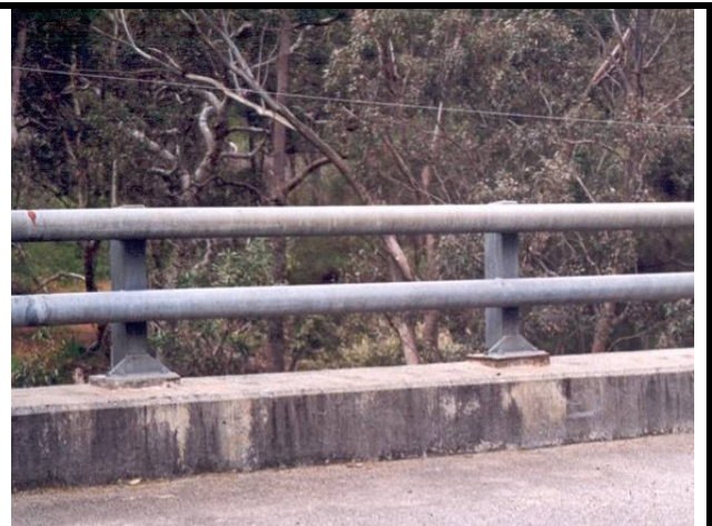
Photo 22 - Steel posts with 2 steel pipe visibility barrier
