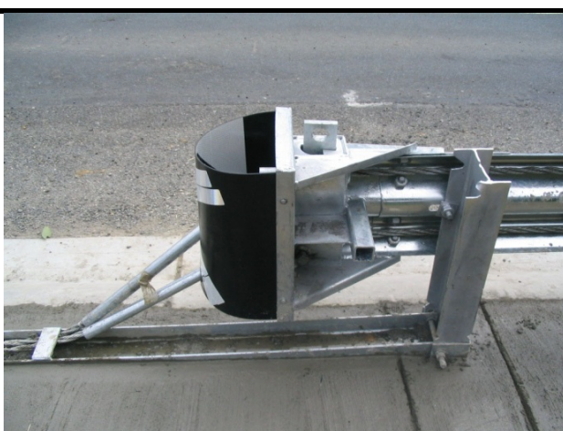
Photo 41 - X Tension (X-350) end terminal
