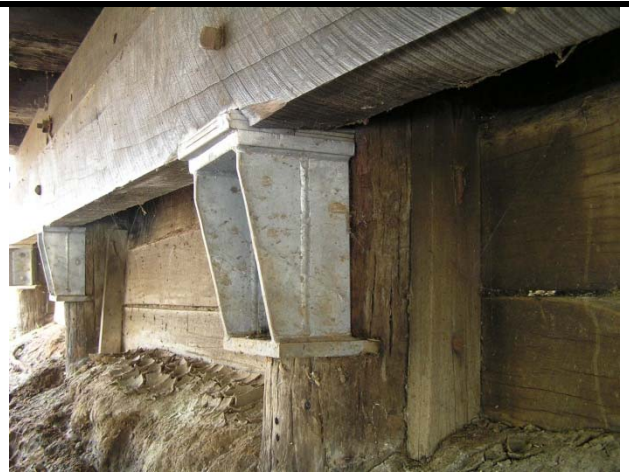
Photo 80 - Steel support bracket for halfcap
