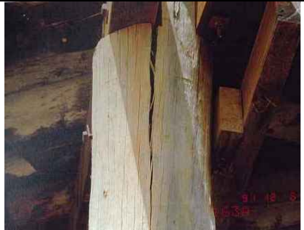
Photo 98 - Shows large vertical (LV) split which requires urgent action for banding
