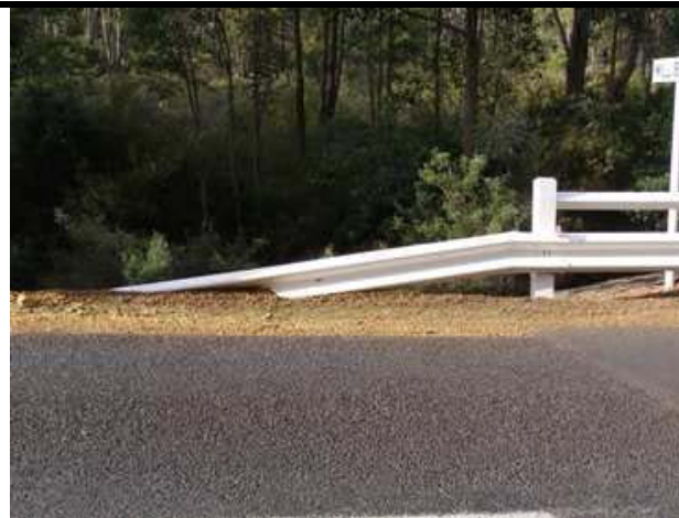
Photo 38 - Turn-down buried end terminal
