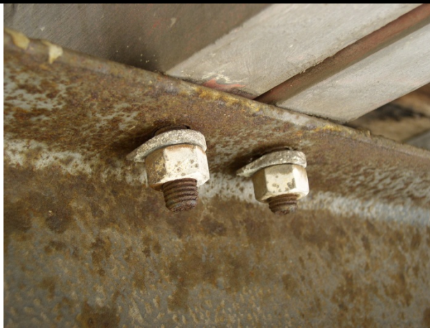
Photo 55 - Bolt tightening required
