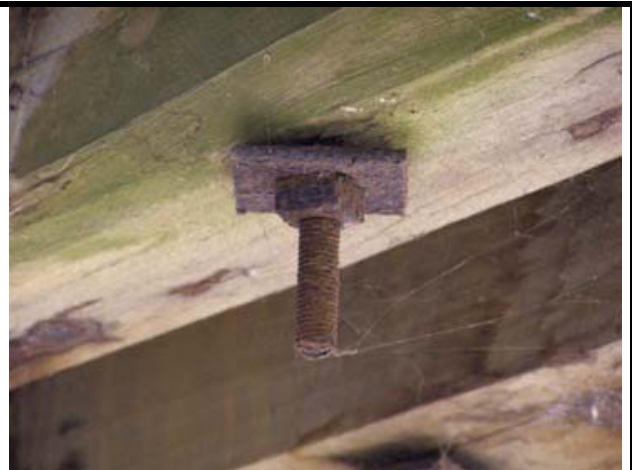
Photo 54 - Bolt tightening required
