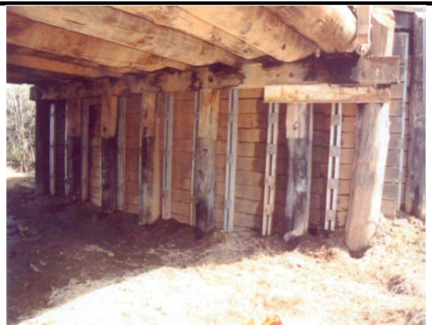
Photo 82 - Tie back bolts in abutment
