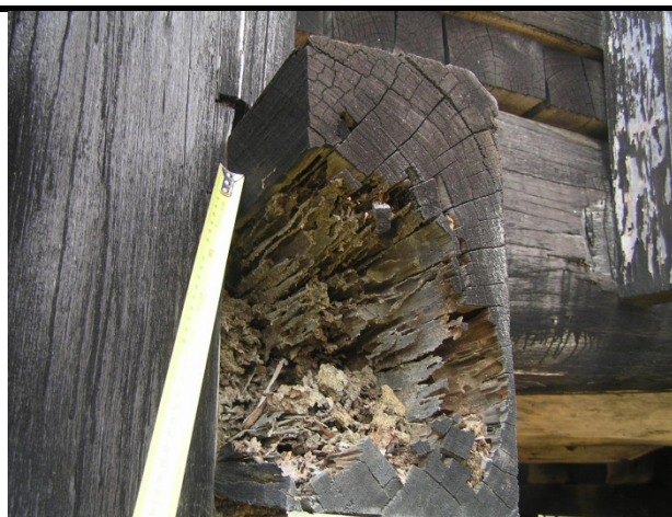
Photo 89 - Rotten halfcap end
