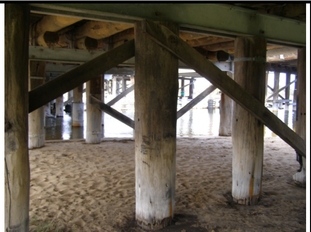
Photo 92 - Typical pier piles
