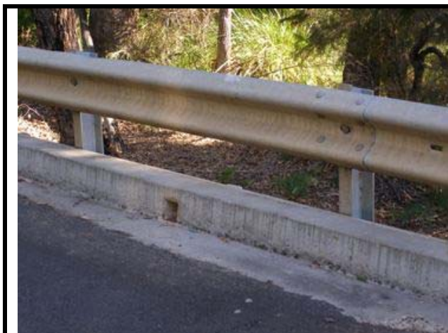
Photo 17 - Steel posts with W Beam barrier
