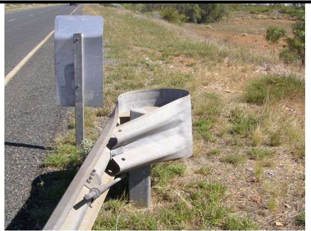
Photo 32 - Bullnose end terminal: w-end bolted (no diaphragm plates)
