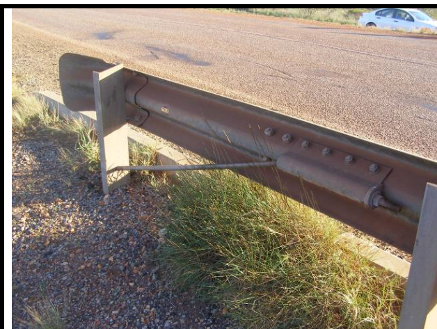
Photo 29 - Fishtail end terminal with tie rod
