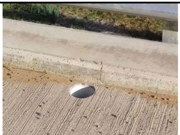
Photo 48 - PVC pipe scupper through deck
