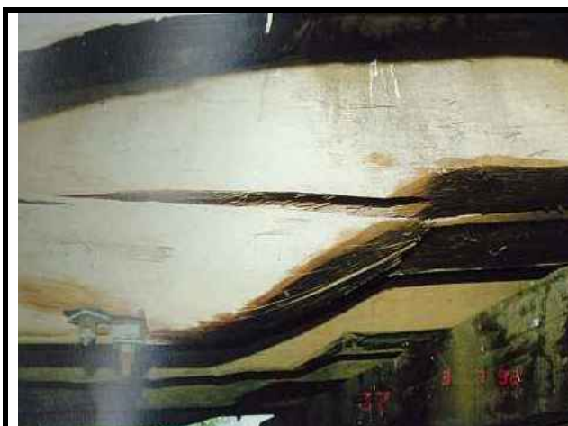
Photo 107 - Shows large horizontal (LH) split. Existing bolt requires tightening.
