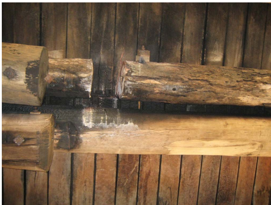
Figure 10.3 - CUT STRINGER TO OBTAIN ACCESS TO THE SEAT OF THE FIRE
