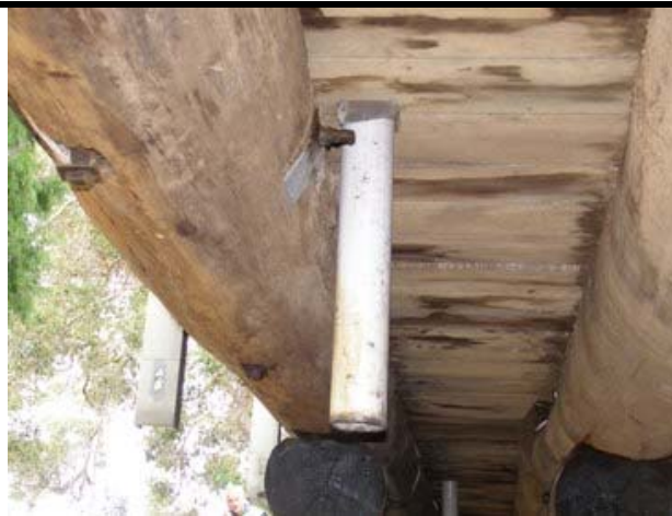
Photo 49 - PVC pipe scupper through deck, extending below stringer
