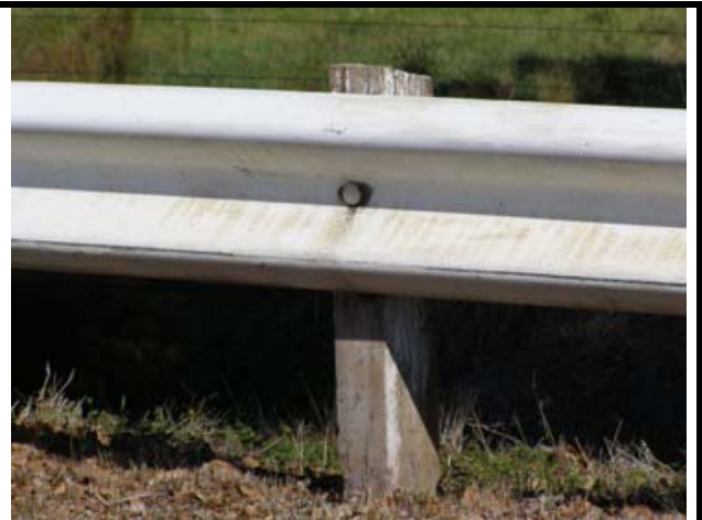
Photo 14 - Timber posts with W Beam barrier
