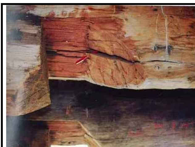
Photo 105 - Shows large (LV) vertical split in stringer. These are common. Bolting required.
