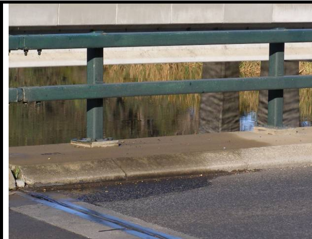
Photo 25 - Steel posts with 2 RHS rails
