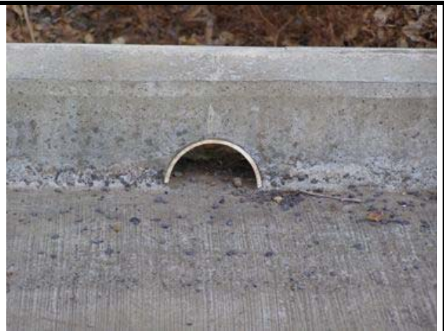
Photo 50 - Half PVC pipe scupper through kerb
