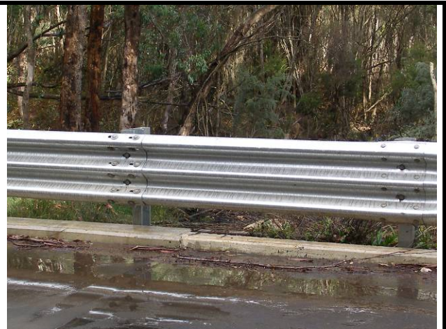
Photo 20 - Steel posts with Thriebeam barrier
