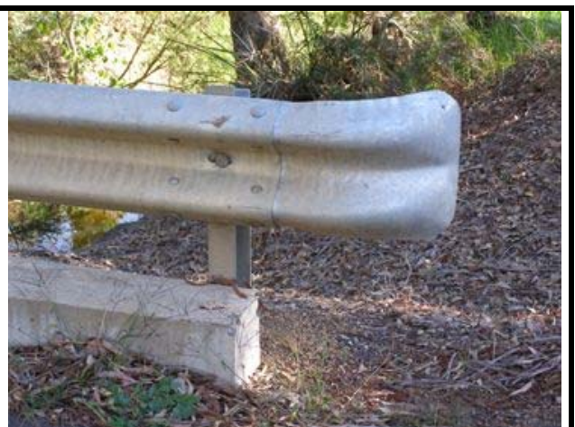
Photo 30 - Fishtail end terminal without tie rod
