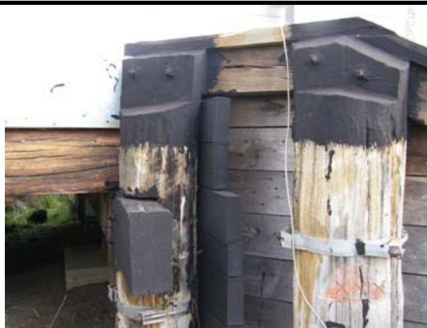
Photo 61 - Preventative end treatment to top of piles
