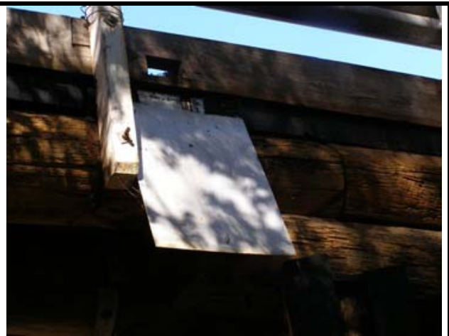
Photo 52 - Typical pressed galvanised iron flashing
