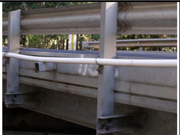
Photo 74 - Telecom pipe attached to the LHS side of the bridge
