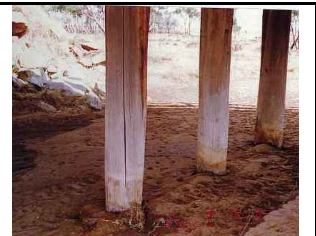
Photo 96 - Shows one long split, multiple banding is required
