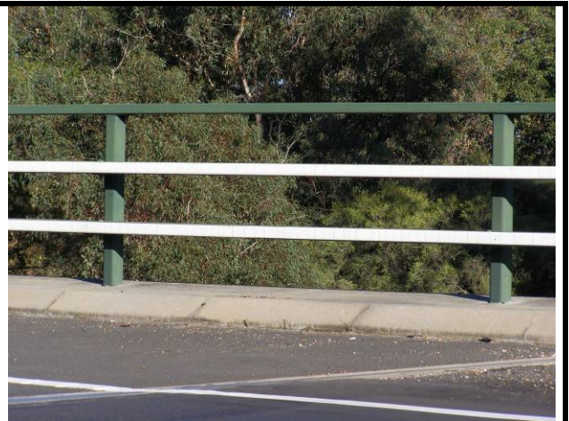
Photo 26 - Steel posts with 2 RHS rails and steel channel top rail
