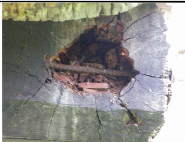
Photo 111 - Example of a damaged corbel
