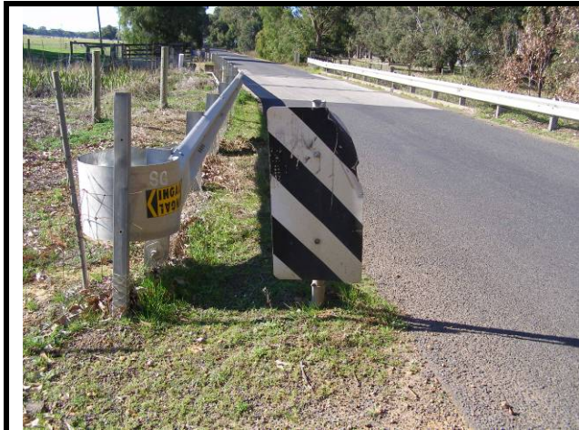
Photo 7 - Width marker in poor condition
