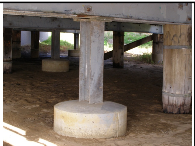
Photo 94 - Pier pile pot type 2
