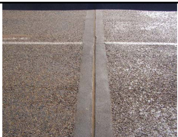
Photo 47 - Pourable joint with nosing
