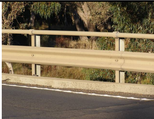
Photo 19 - Steel posts with W Beam barrier and steel pipe top rail
