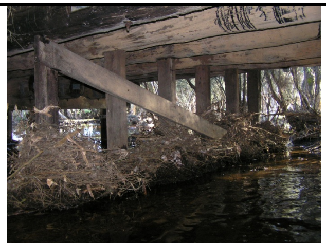
Photo 66 - Build-up of vegetation debris against piles
