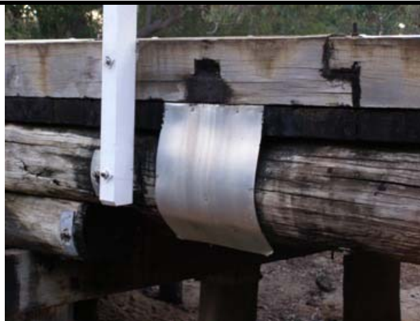
Photo 53 - Typical pressed galvanised iron flashing
