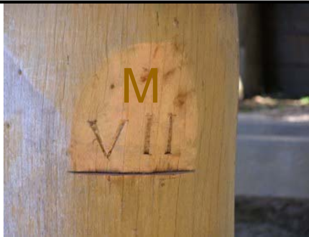
Photo 79 - Blaze marking with "M" above is measured in metres
