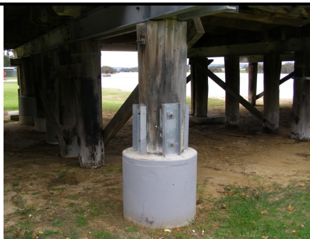
Photo 93 - Pier pile pot type 1
