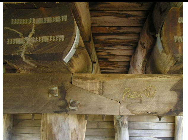
Photo 86 - Typical halfcap joint
