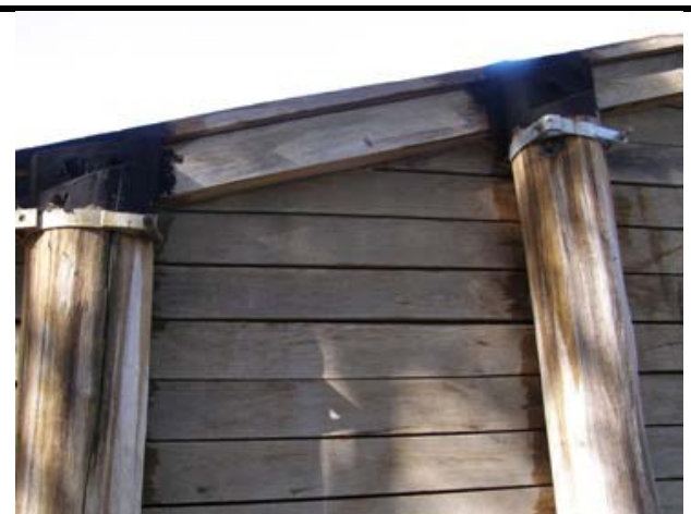
Photo 90 - Typical wing wall timber sheeting
