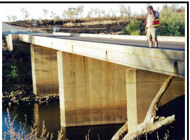
Photo 10 - Bridge with no railing
