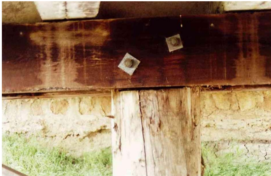
Figure 8.4 - EXAMPLE OF HALFCAP NOT SEATED ON PILE
