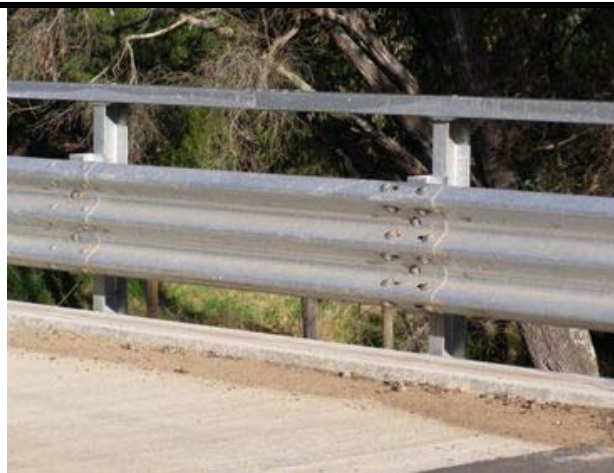
Photo 21 - Steel posts with Thriebeam barrier and steel channel top rail
