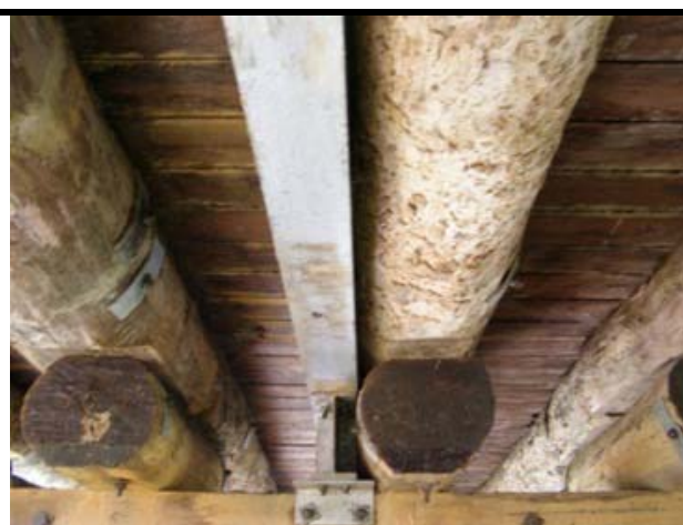
Photo 108 - Timber stringer with steel stringer alongside
