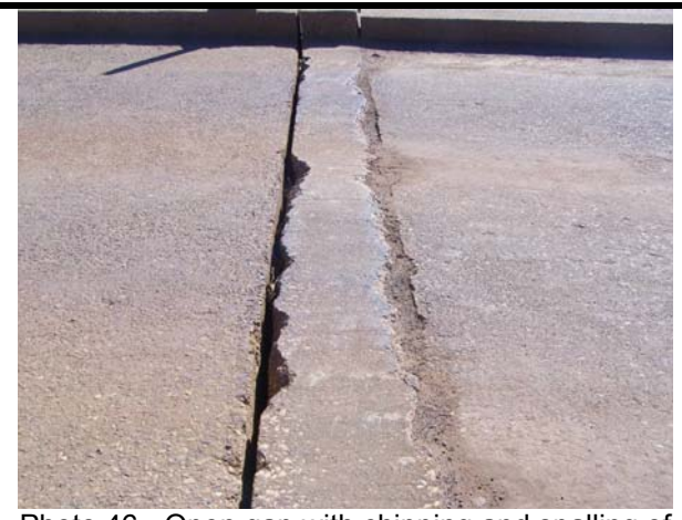
Photo 46 - Open gap with chipping and spalling of the joint
