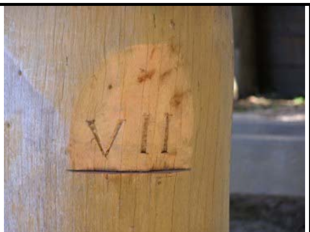
Photo 78 - Driven depth mark (blaze)
