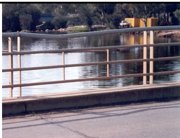
Photo 23 - Steel posts with 4 steel pipe visibility barrier
