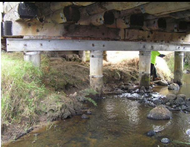
Photo 99 - Steel halfcap under an existing timber halfcap
