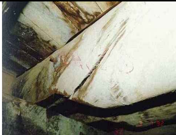
Photo 109 - Shows LV twisting type of split. This split can spiral around the entire stringer.
