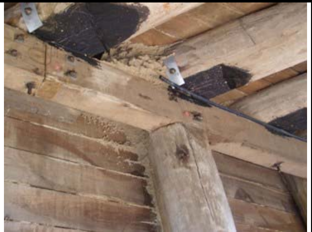
Photo 56 - Termite nest on top of halfcap and behind pile
