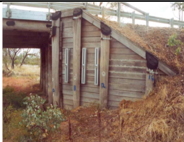
Photo 83 - Tie back bolts in wing wall
