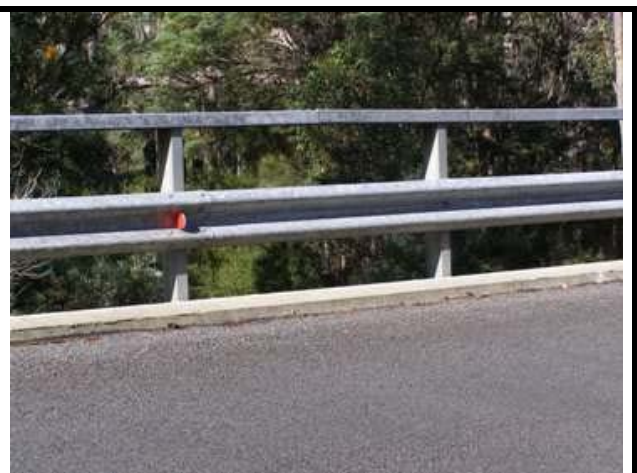
Photo 18 - Steel posts with W beam barrier and steel channel top rail
