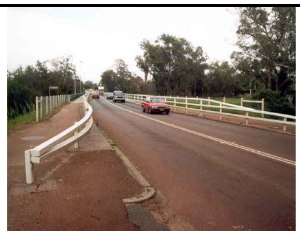
Photo 39 - Abrupt termination, no end terminal
