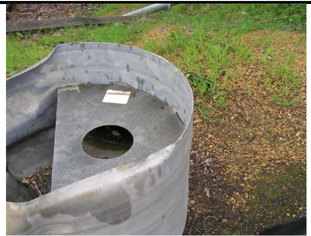
Photo 34 - Bullnose end terminal with 1 and 2 diaphragm plates
