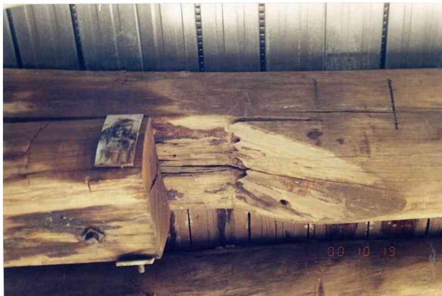
Figure 8.2 - EXAMPLE OF STRINGER SPLITTING AT HAUNCH
