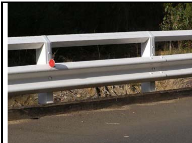
Photo 15 - Timber posts with W Beam barrier and timber top rail
