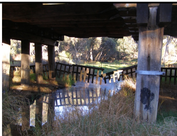
Photo 65 - Fence attached to bridge across waterway
