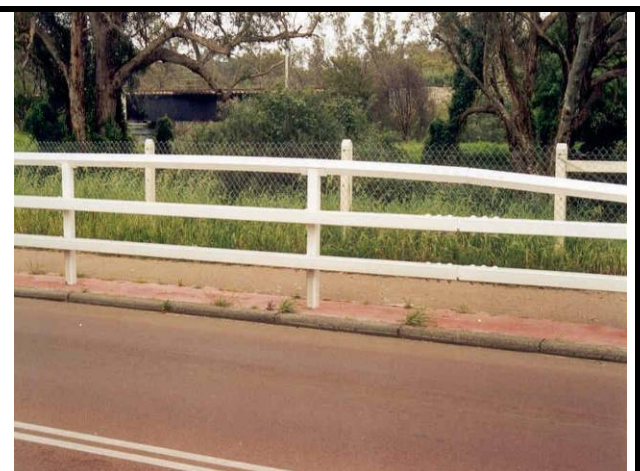
Photo 24 - Steel posts with 2 RHS rails and RHS "Diamond" top rail
