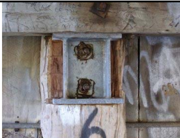
Photo 81 - Steel support bracket for halfcap
