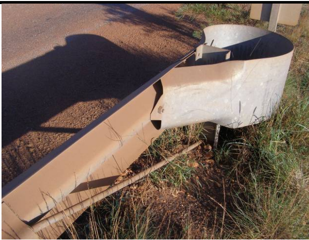
Photo 33 - Bullnose end terminal: flat end bolted (no diaphragm plates)
