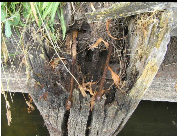
Photo 101 - Photo of end of pile with splits
