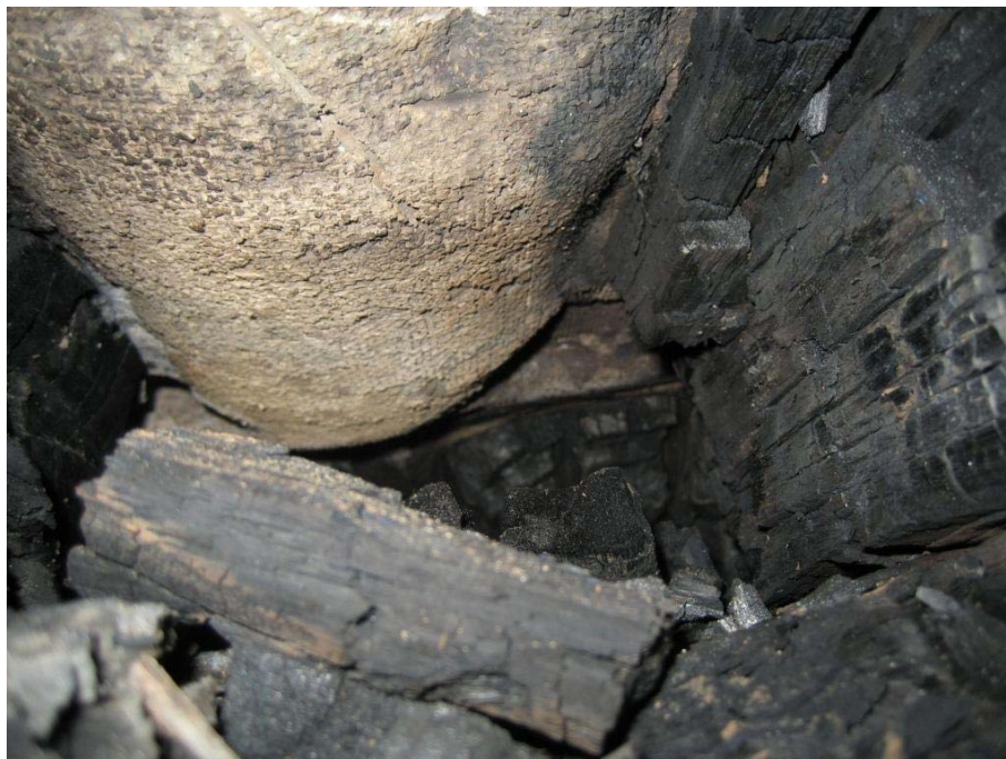
Figure 10.2 - FIRE DAMAGE IN A TIMBER BRIDGE
