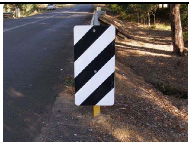
Photo 6 - Width marker in good condition
