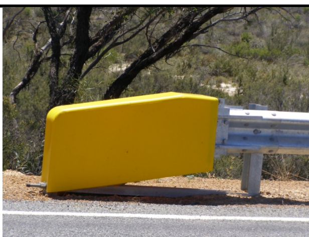
Photo 42 - X Tension (350) end terminal
