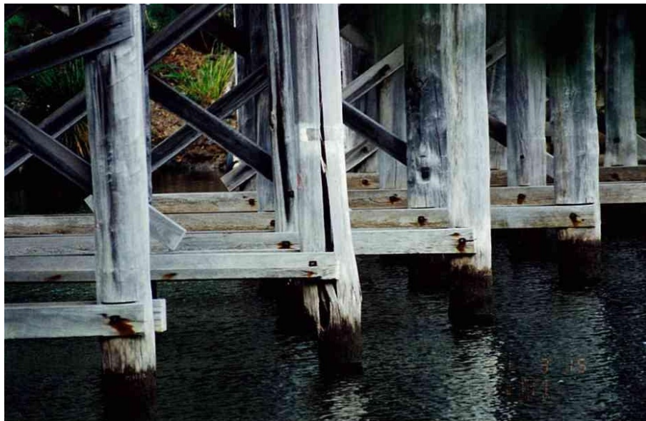
Figure 8.3 - EXAMPLE OF SPLIT TIMBER PILE
