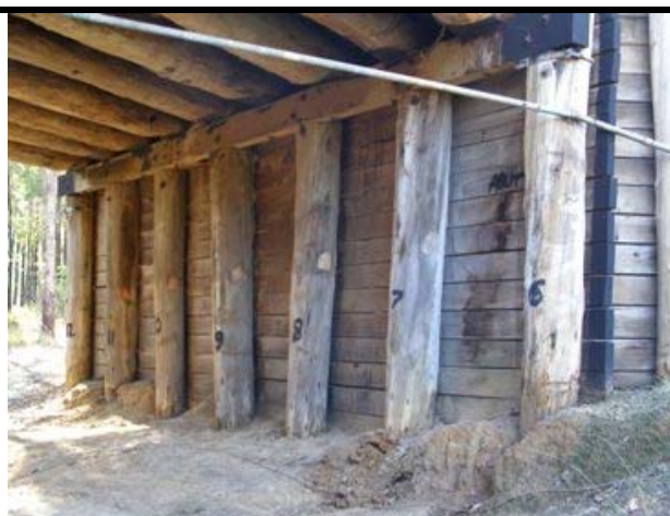
Photo 77 - Typical abutment piles, Abutment 1
