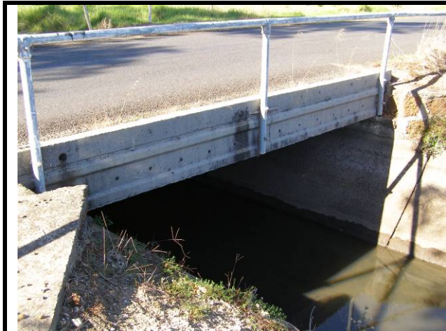
Photo 13 - Steel pipe visibility barrier
