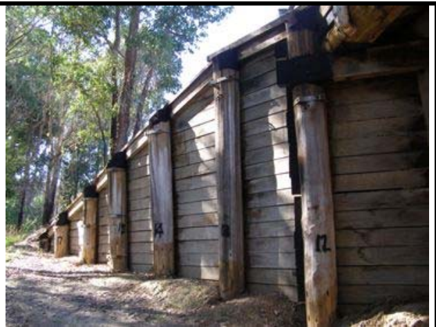
Photo 76 - Typical wing wall piles, Abutment 1, RHS
