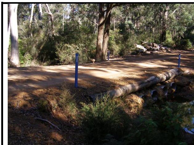
Photo 11 - Bridge with no railing
