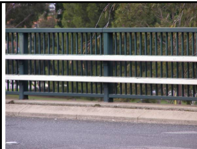
Photo 27 - Steel balustrade with RHS rails
