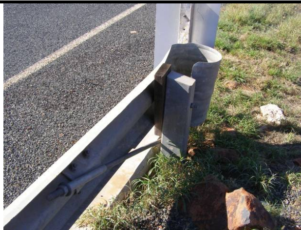
Photo 31 - Non-standard bullnose end terminal
