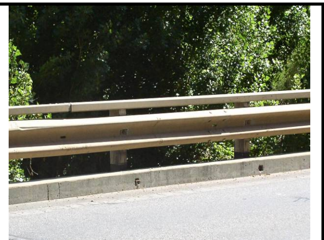
Photo 16 - Timber posts with W Beam barrier and steel top rail
