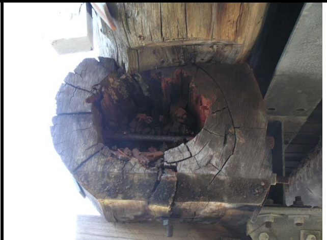
Photo 110 - Splits and rot hole in end of corbel. It is crushing and failing.
