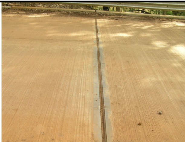
Photo 45 - Compression seal in good condition
