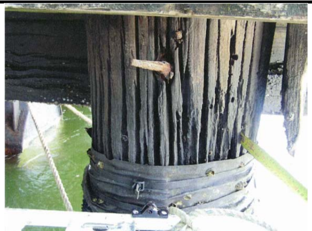
Photo 102 - Example of a damaged pile
