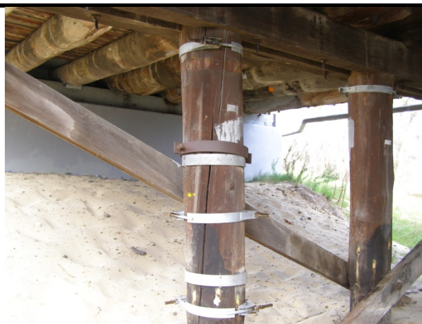
Photo 95 - Pile with multiple bands
