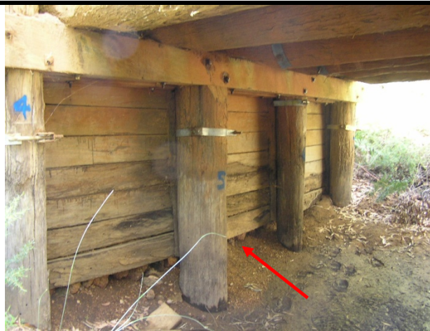
Photo 73 - Scour at Abutment 2
