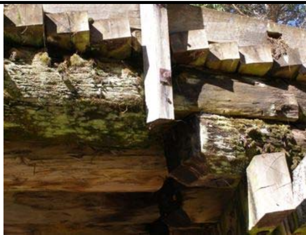
Photo 63 - Preventative treatment required Note: moss on side of stringer and corbel
