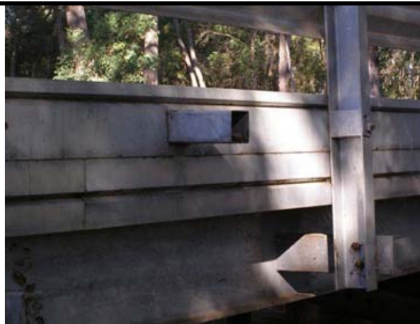
Photo 51 - Box scupper through kerb
