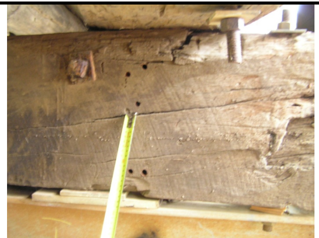
Photo 88 - Horizontal and vertical splits in a halfcap
