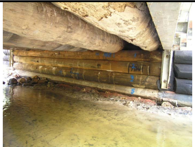
Photo 84 - Typical bedlog abutment
