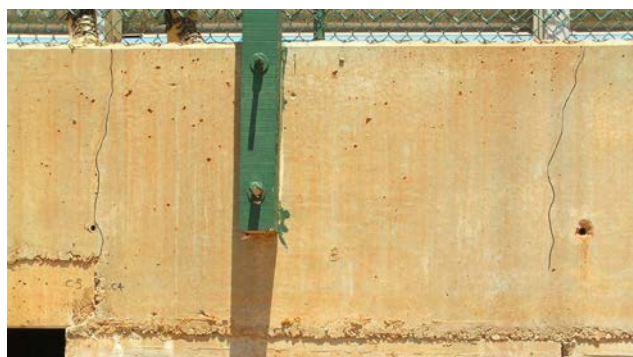
Widely spaced medium cracks in the structural head wall.
