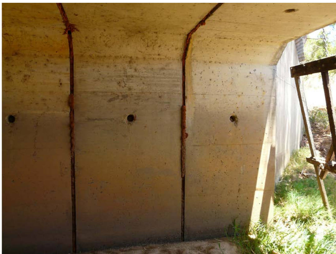
Photo No. 6: Barrel No.1 – typical gaps between units (Taken: 14-Mar-2010)
