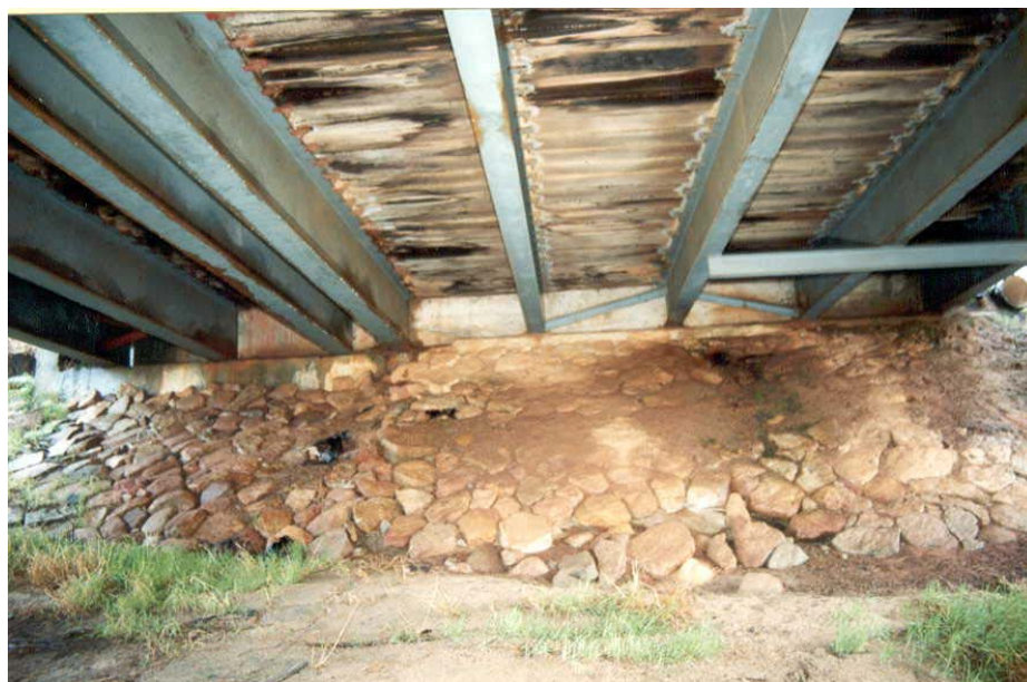
FIGURE E.2.6B(2) - TIMBER DECKING ON STEEL BEAMS – VIEW FROM UNDERSIDE OF BRIDGE
