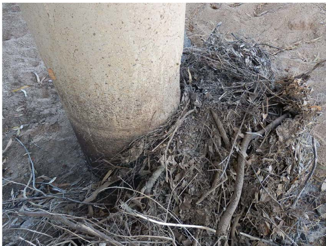
Photo No. 30: Flood debris up against previous fire damaged column. Unable to remove by hand but no obvious signs of deterioration to upper section that could be seen. (Taken: 31-Jul-2013)
