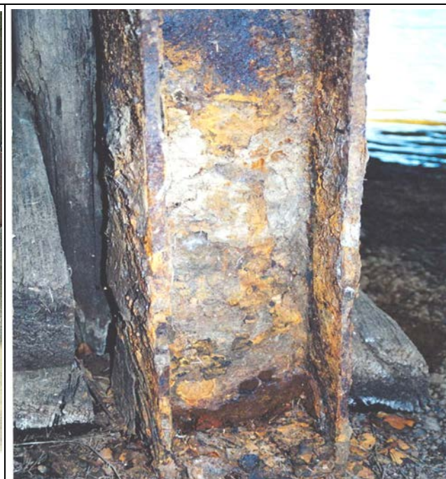
Severely corroded steel section.
