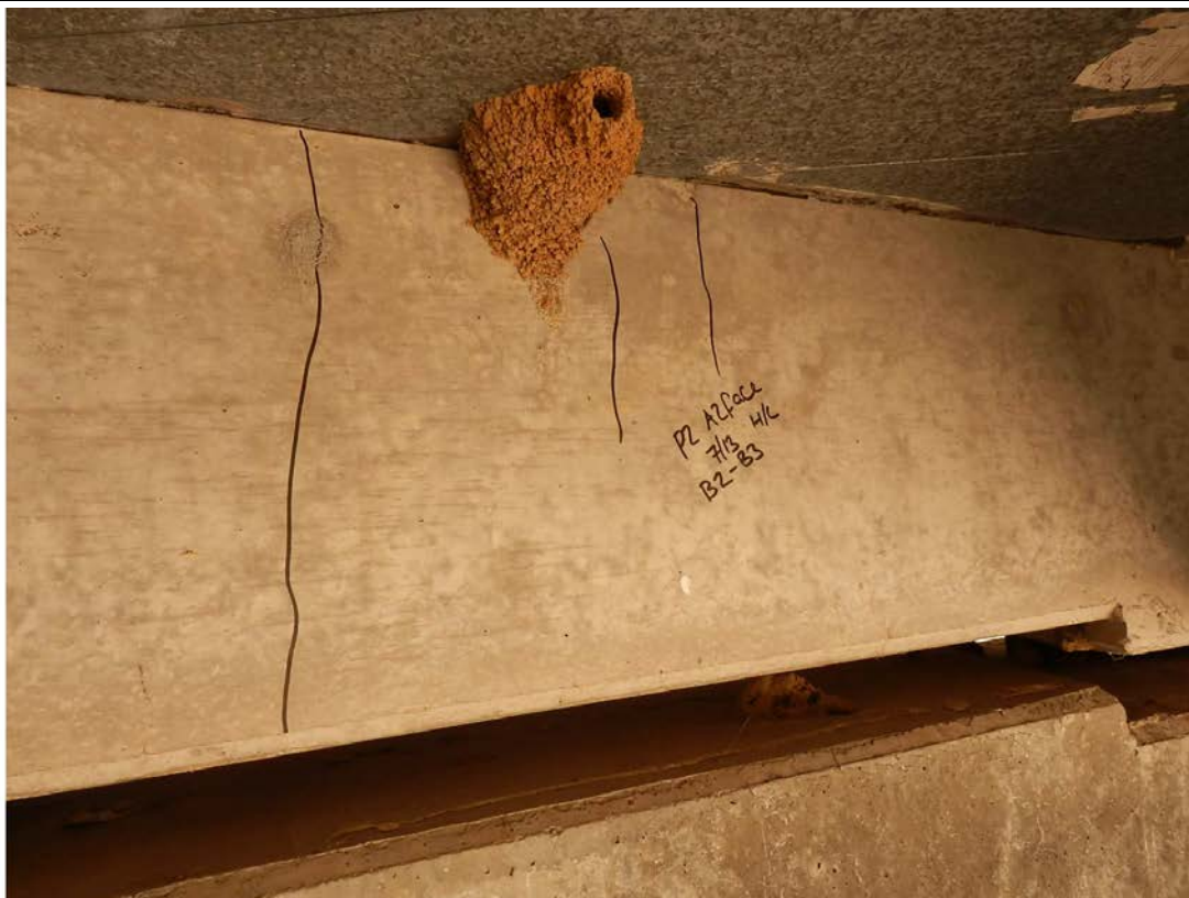
Photo No. 41: Pier 2 abutment 2 face. Hairline cracks in diaphragm between beams 2 and 3. (Taken: 31-Jul-2013)
