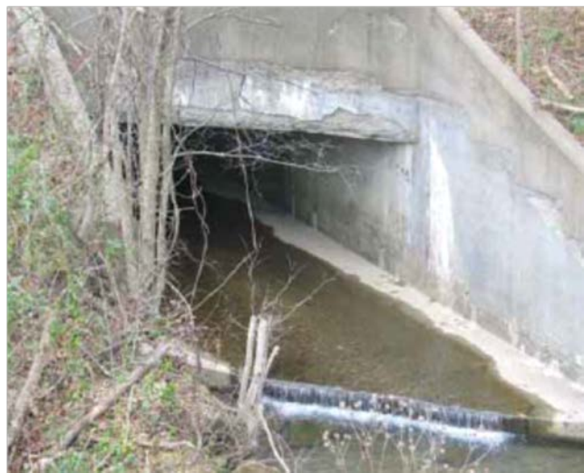
Heavy cracking and spalling in the headwall and wing wall with efflorescence.
