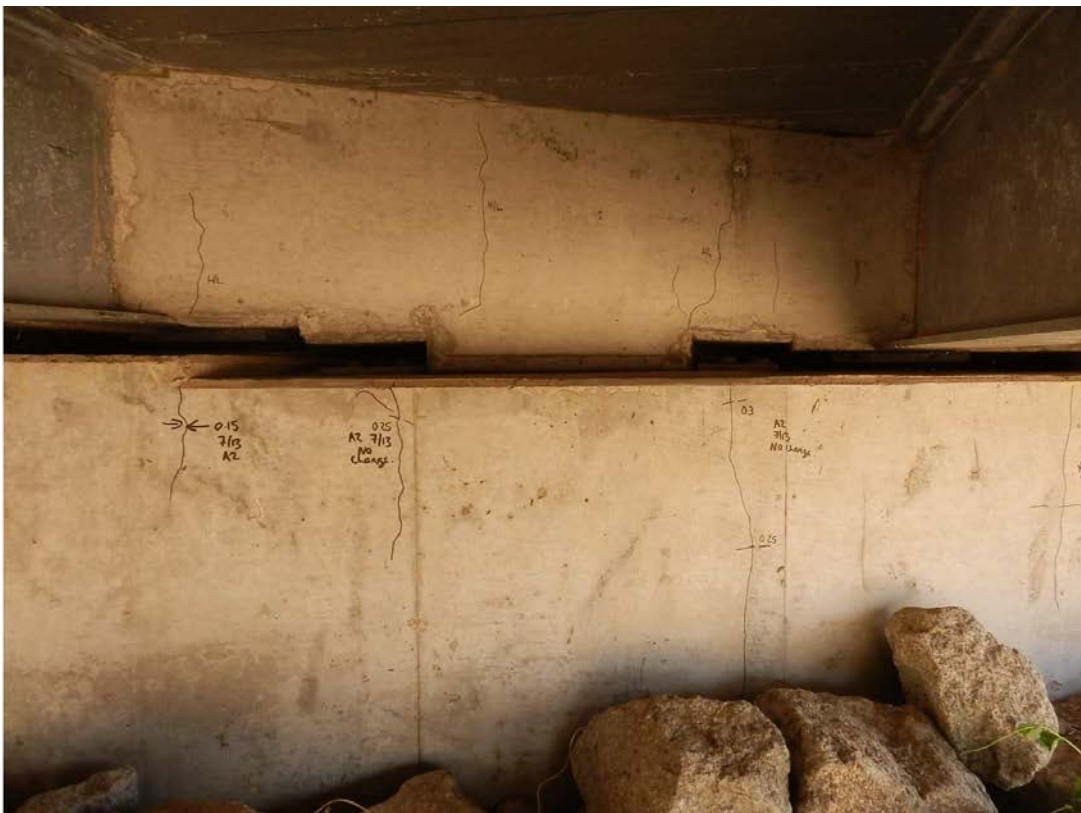
Photo No. 60: Abutment 2. Cracking to capbeam and diaphragm at shear key. (Taken: 30-Jul-2013)
