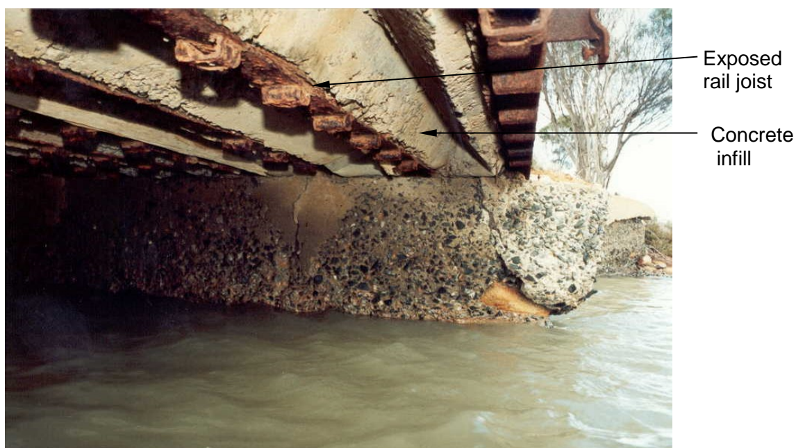
FIGURE E.2.1F(2) - FILLER JOIST BRIDGE WITH EXPOSED JOISTS
