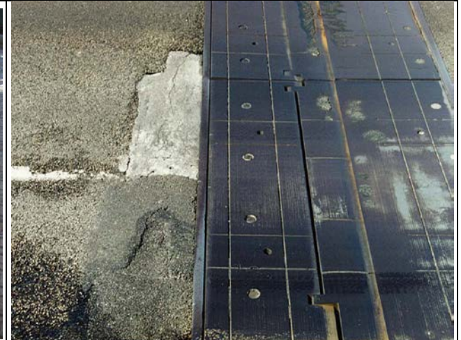
Road surface repaired, plate appears warped, and worn. Insufficient gap for movement.
