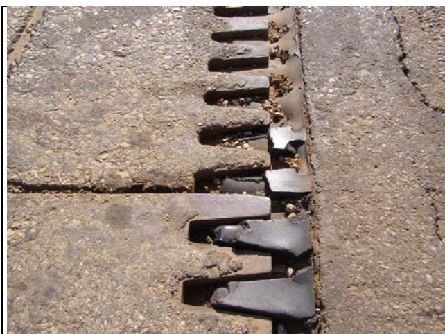
The debris build-up would indicate a significant blockage to movement.
