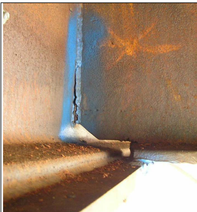
Significant cracking of weld. Section could potentially fail.
