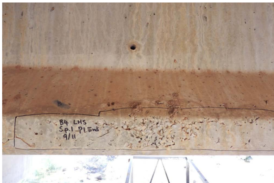
FIGURE 9.3 - HONEYCOMBING (AREA DEFECT) MARK-UP
