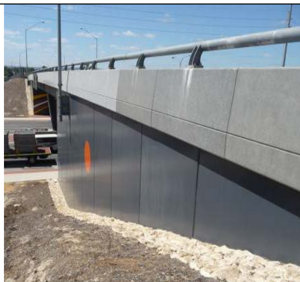
MSE wing wall in excellent condition.
