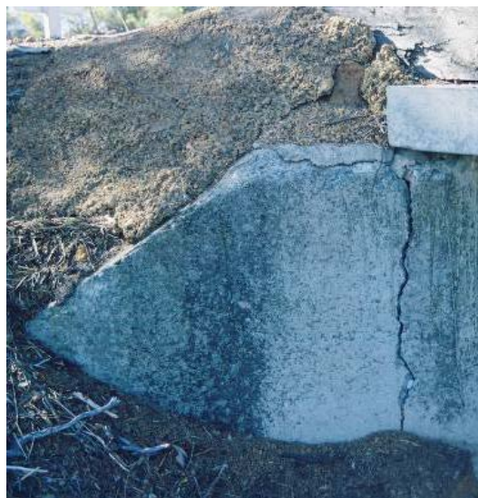
Heavy vertical crack in the wing wall but appears stable.
