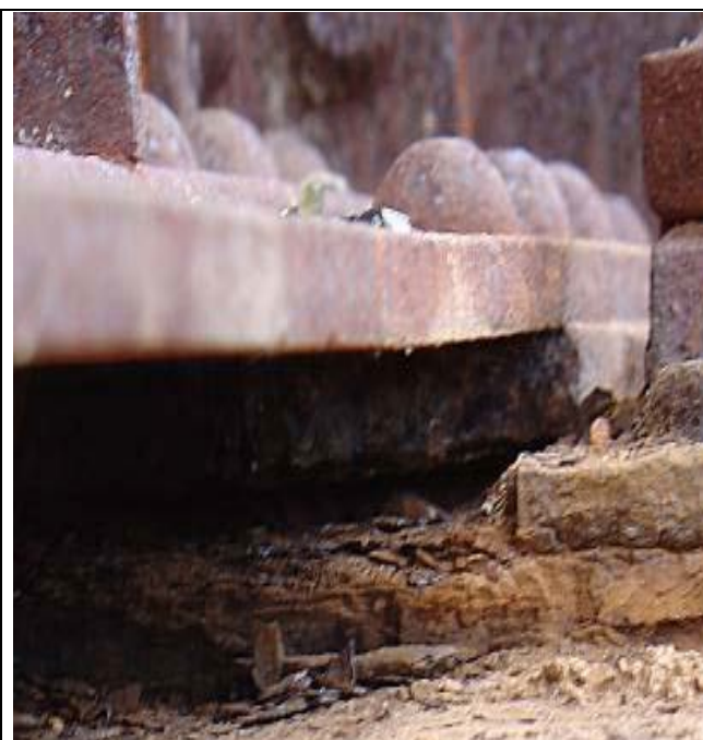
Steel components and holding down connections with advanced corrosion and heavy pitting.
