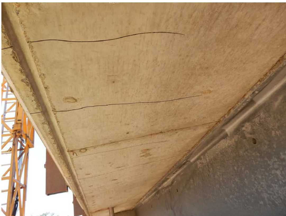
Photo No. 52: Span 4, left hand side cantilever. Hairline cracking at approximately 400mm centres. (Taken: 31-Jul-2013)
