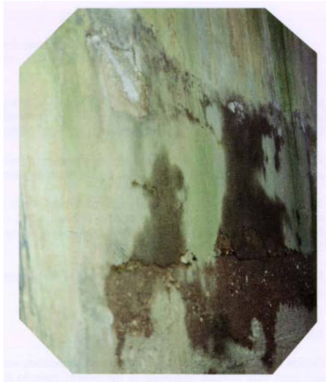
FIGURE 11.2A - SCALING OF CONCRETE
