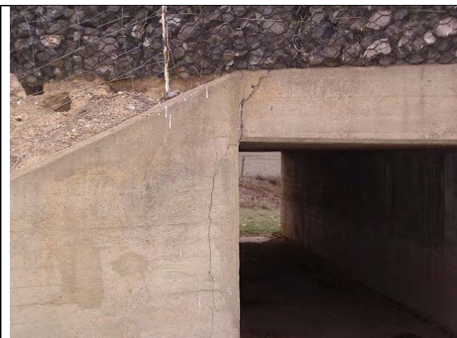
Vertical medium cracking on the wing wall.
