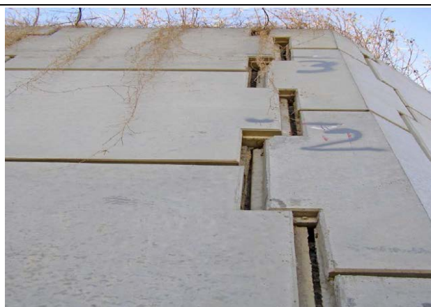
MSE wall panels have separated up to 50 mm.
