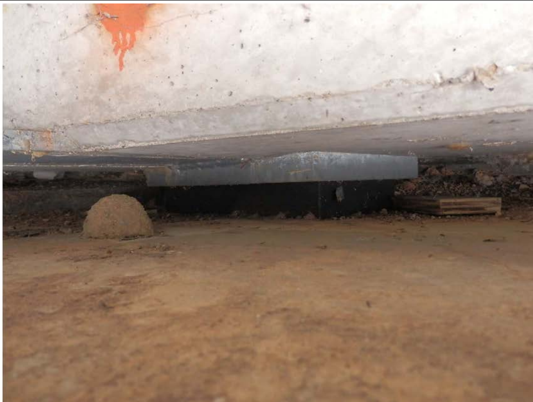
Photo No. 21: Abutment 1, bearing pad 2 of 5. (Taken: 30-Jul-2013)
