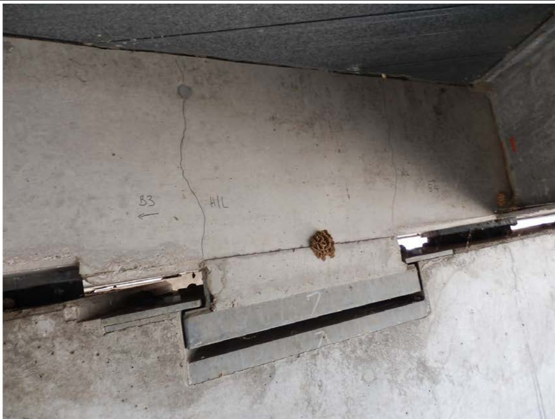
Photo No. 31: Pier 1 shear key/ diaphragm. Hairline cracks from internal corner up to shutter bolt hole. Abutment 1 face. (Taken: 31-Jul-2013)
