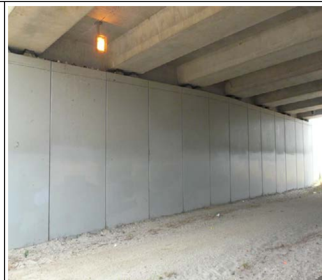
Only minor coating defects, structurally 'as new'.
