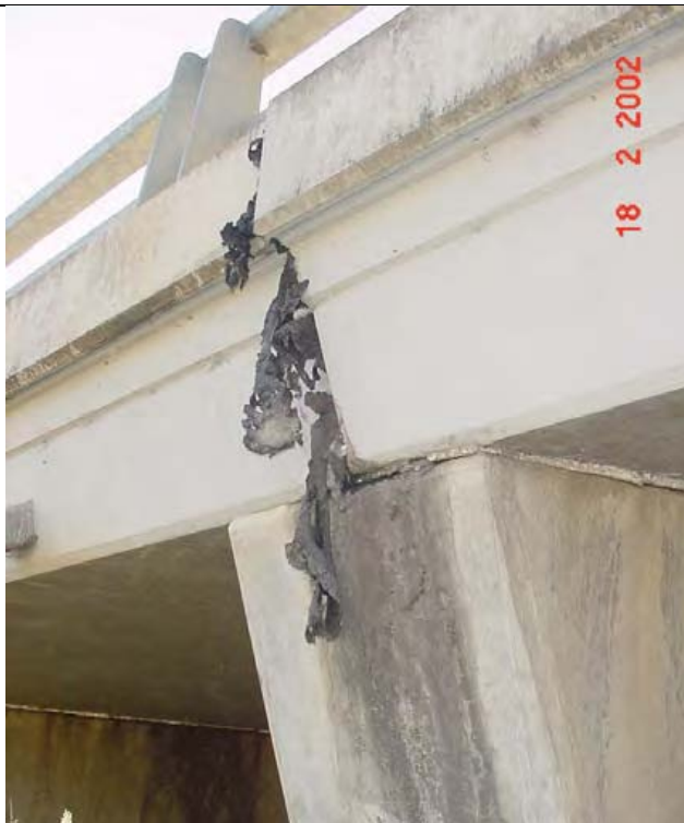
Significant loss of sealant.
