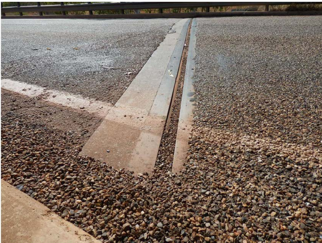
Photo No. 10: Abutment 1 expansion joint. Compressive seal gap full of road debris. (Taken: 30-Jul-2013)
