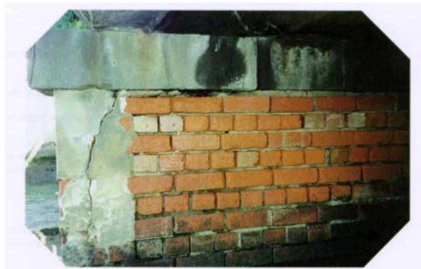
FIGURE 13.3 - MASONRY WALL WITH LOSS OF MORTAR
