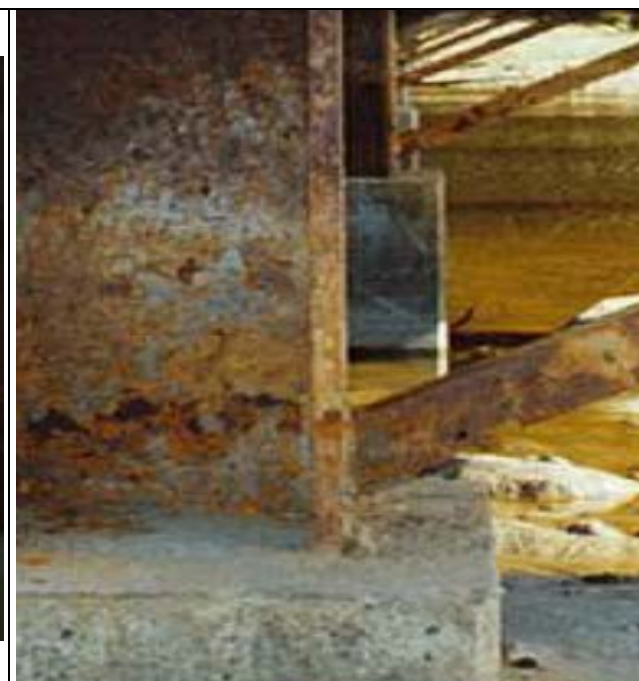
The flanges have only minor section loss, the flaking on the web indicates a greater loss of section.
