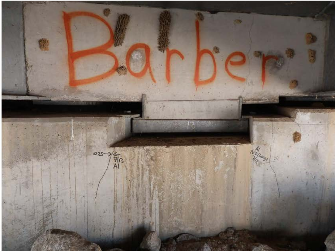
Photo No. 23: Abutment 1 diaphragm and capbeam. 0.25mm cracks as previously recorded. (Taken: 30-Jul-2013)
