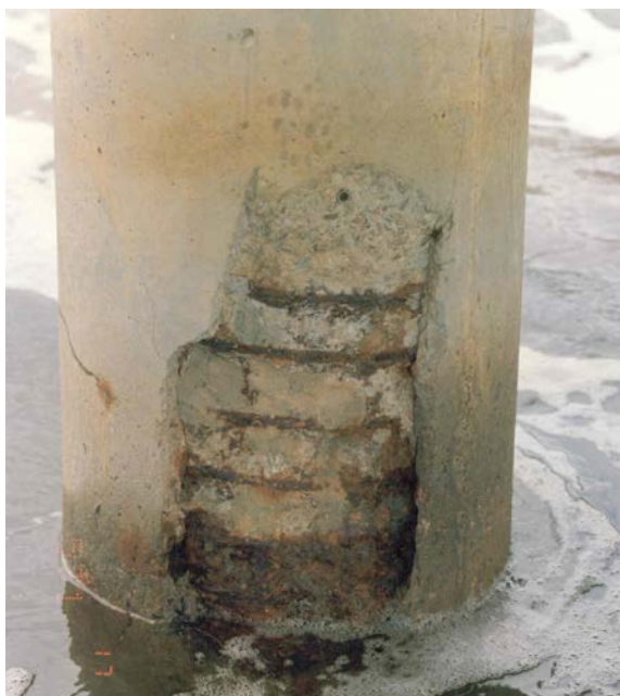
FIGURE 11.4B - CORROSION OF REINFORCEMENT ACCOMPANIED BY SPALLING
