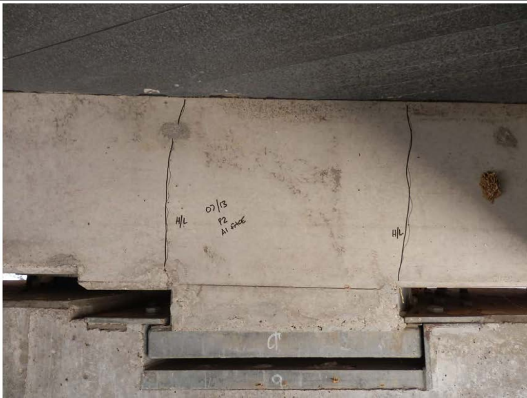
Photo No. 39: Pier 2 abutment 1 face. Hairline cracking at shear key. (Taken: 31-Jul-2013)
