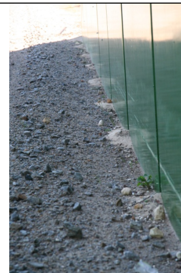
Minor loss of embankment fill between the MSE wall panels.
