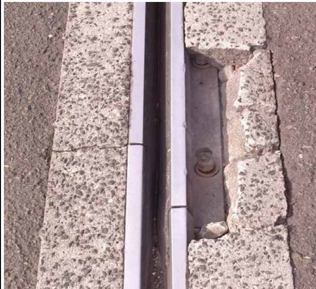
Significant spall and loose nut with loss of connectivity between the deck and joint.
