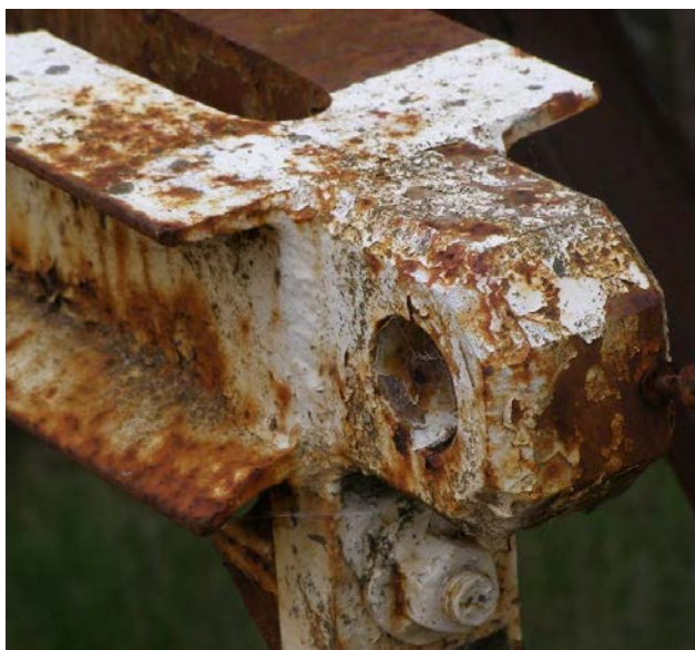
Moderate pitting with some section loss although still serviceable.
