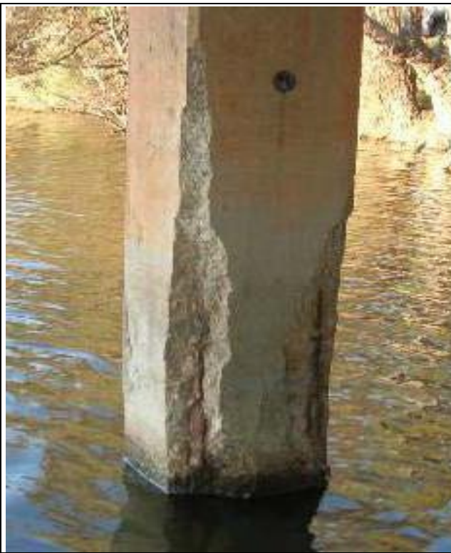
Reduced section capacity based on loss of section area from spalling, in tidal zone so assume deterioration will proceed rapidly.
