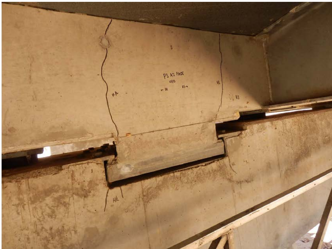
Photo No. 48: Pier 3 abutment 2 face. Minor hairline cracking. (Taken: 31-Jul-2013)
