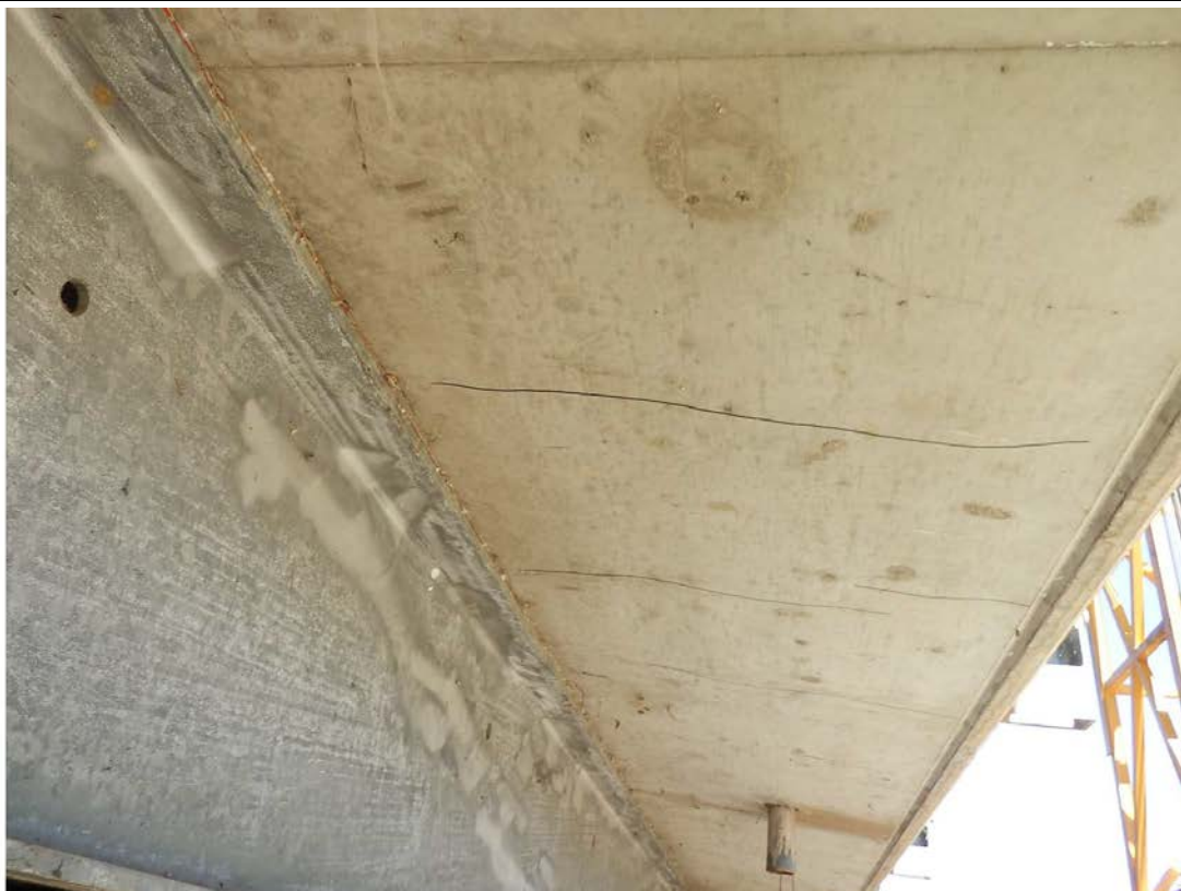
Photo No. 27: Hairline cracking to left hand side cantilever of span 1. (Taken: 31-Jul-2013)
