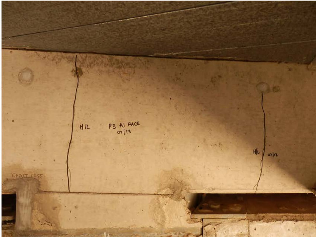
Photo No. 47: Pier 3 abutment 1 face. Hairline cracking. (Taken: 31-Jul-2013)
