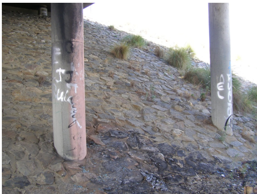
FIGURE 11.12 - FIRE DAMAGE TO CONCRETE COLUMN
