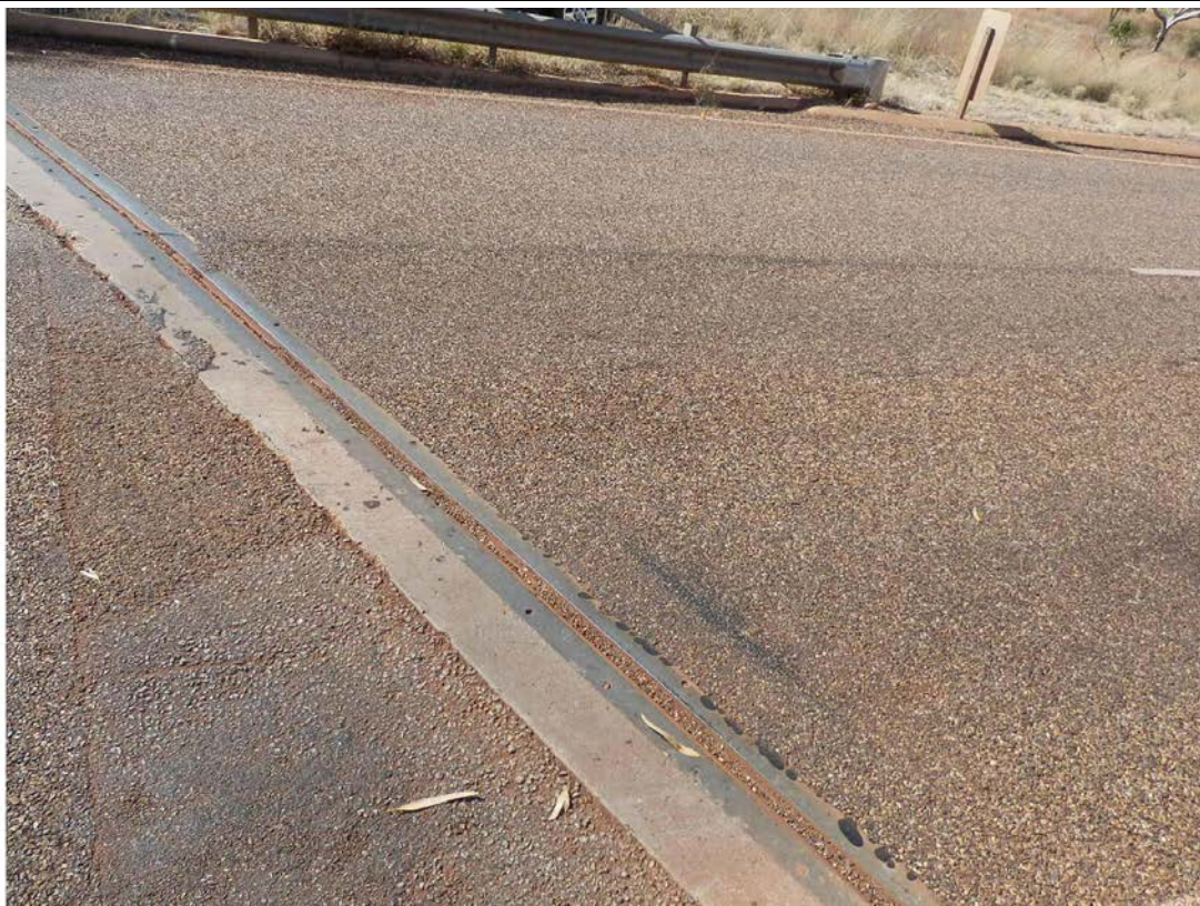
Photo No. 11: Abutment 1 end. Surfacing over buried approach slab. (Taken: 30-Jul-2013)
