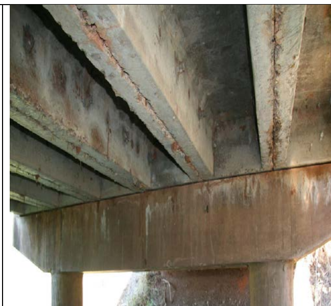
Staining indicates hidden issues and some minor deterioration. Warrants a CS2 even though there is no obvious cracking.
