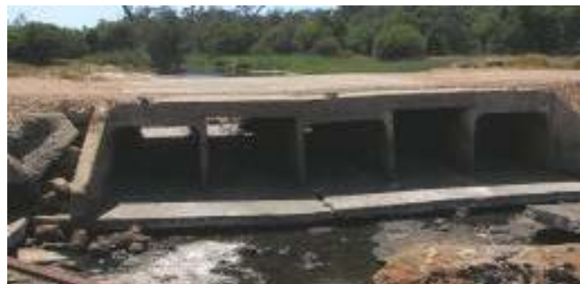
Apron failure with potential loss of entire box unit bridge.
