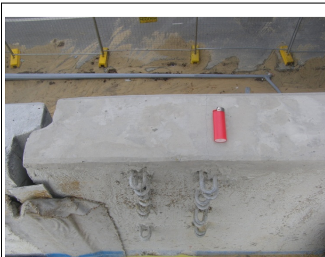
Minor movement of MSE wall panels. No significant loss of fill.
