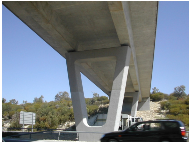
FIGURE E.2.2G(1) - PRESTRESSED CONCRETE DOUBLE T-BEAM SUPERSTRUCTURE CAST IN SITU
