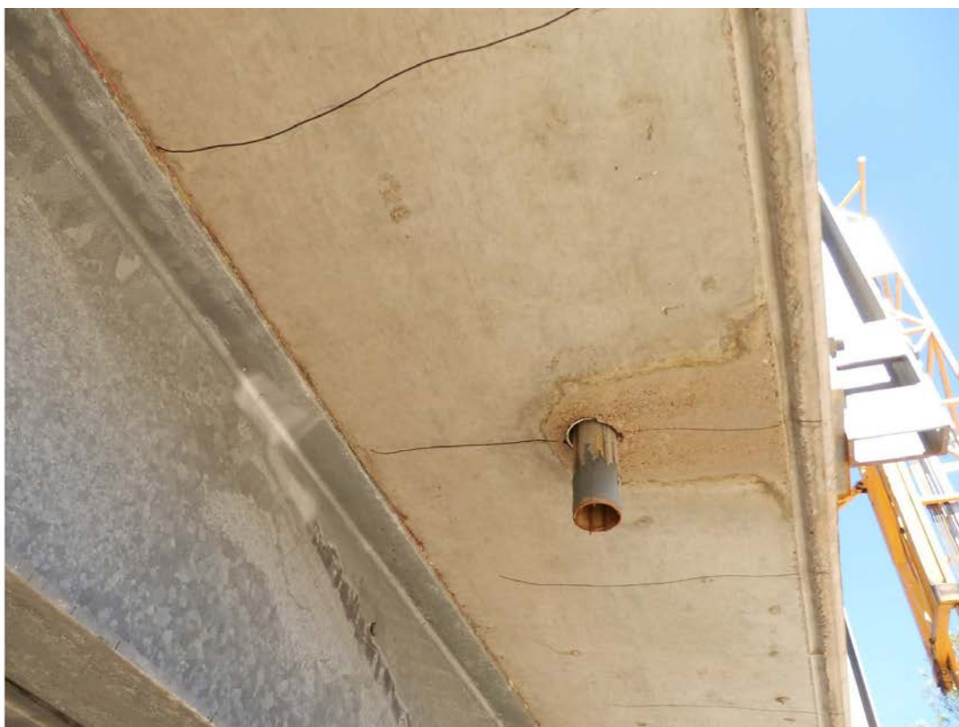
Photo No. 44: Span 3 left hand side cantilever. Transverse hairline cracks. (Taken: 31-Jul-2013)
