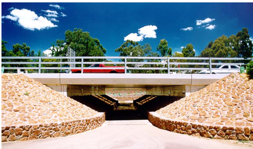
FIGURE E.2.1C - REINFORCED CONCRETE PRECAST PLANK WITH IN SITU TOPPING
