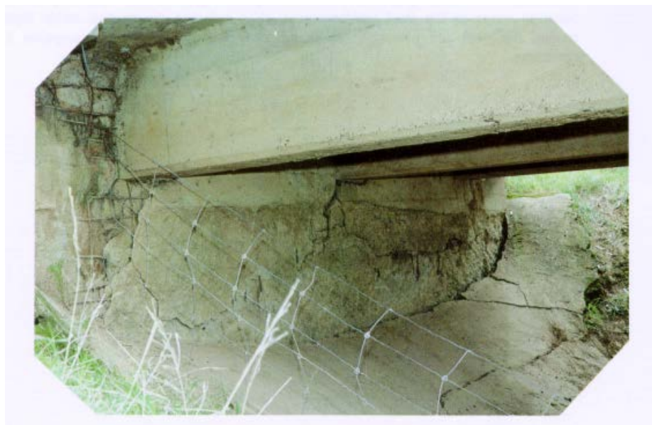
FIGURE 11.2B - DISINTEGRATION OF CONCRETE
