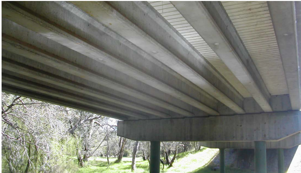
FIGURE E.2.1G - REINFORCED CONCRETE PRECAST BEAM WITH IN SITU SLAB
