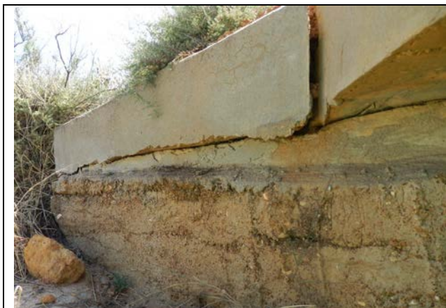
Wing wall has moved away from the abutment wall.
