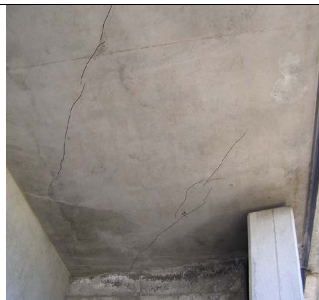
Widely spaced fine cracking. Water staining prevalent in more sheltered areas.
