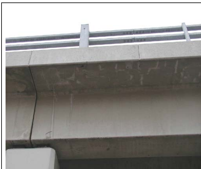
Closely spaced hairline cracks as indicated by the efflorescence.
