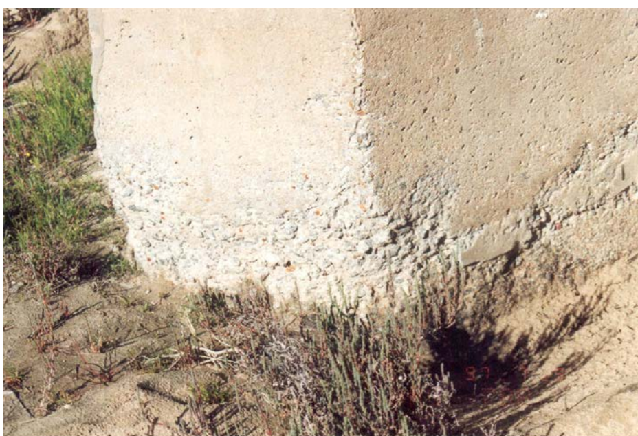
FIGURE 11.11 - EROSION OF CONCRETE DUE TO WATER WASH
