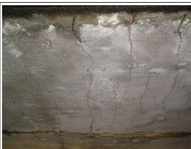
Frequent cracking greater than 0.3 mm.
