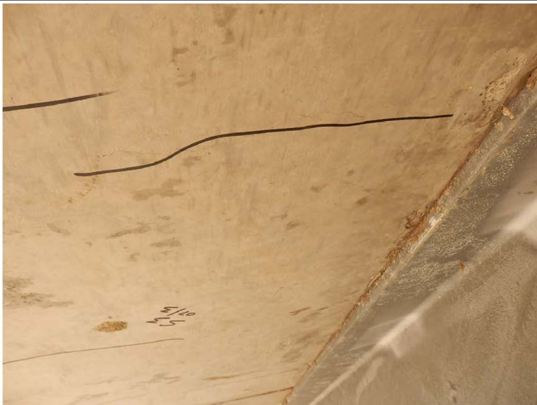
Photo No. 43: Span 3 left hand side cantilever. Transverse hairline cracks. (Taken: 31-Jul-2013)
