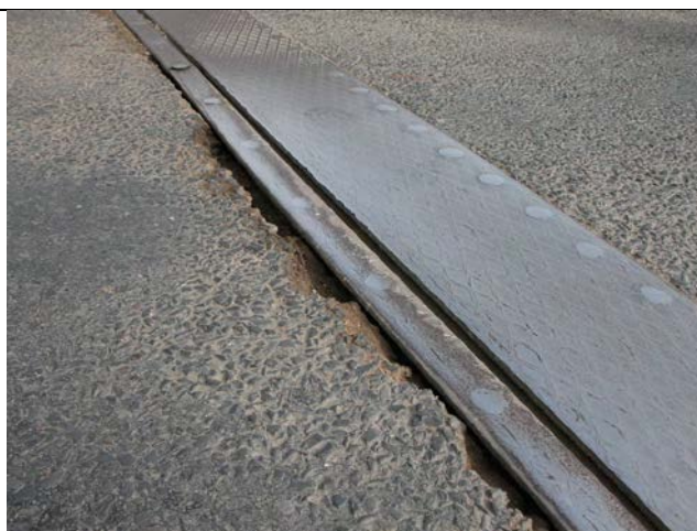
Significant spalling of concrete adjacent to the joint.
