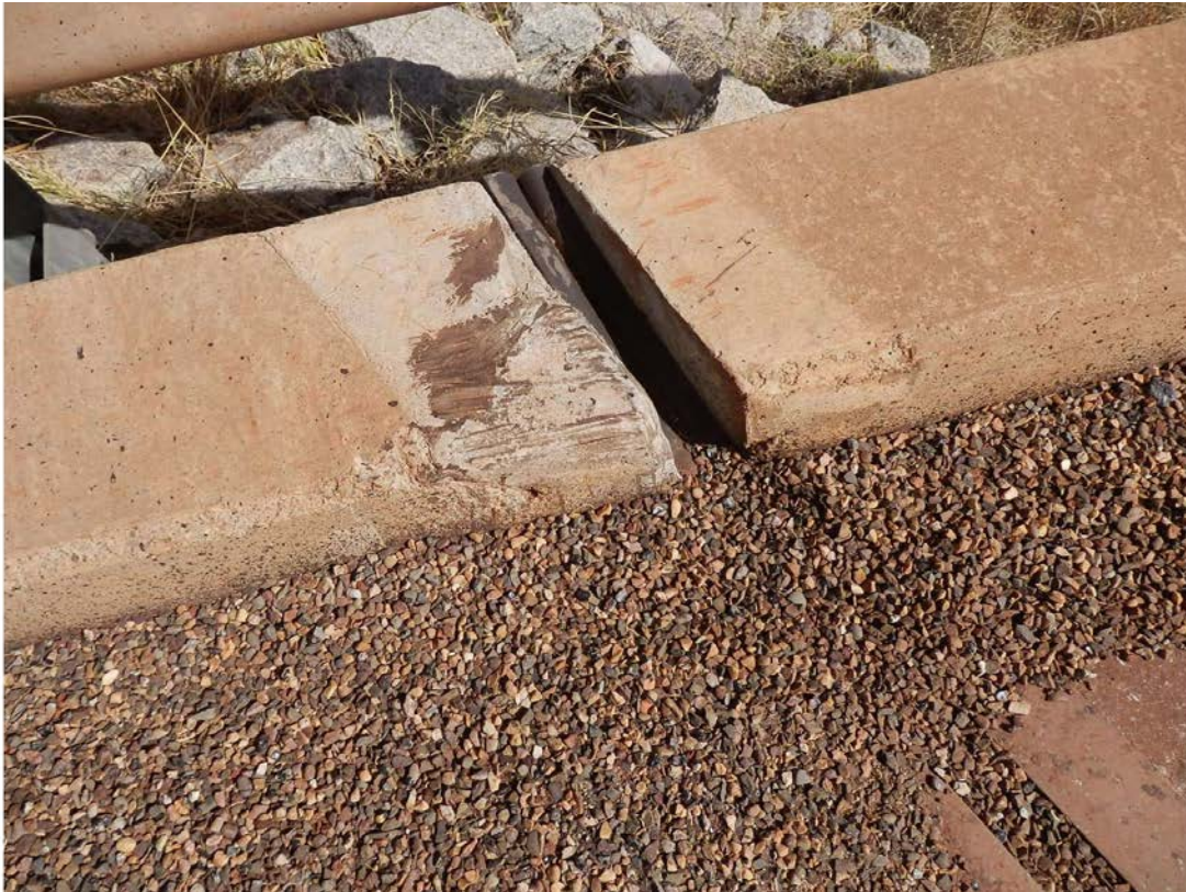
Photo No. 9: Abutment 1 expansion joint cover plate to kerb missing. Road debris filling joint gap. (Taken: 30-Jul-2013)
