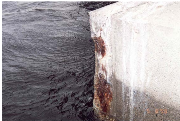
FIGURE 11.4A - SPALLING OF CONCRETE IN PILE CAP
