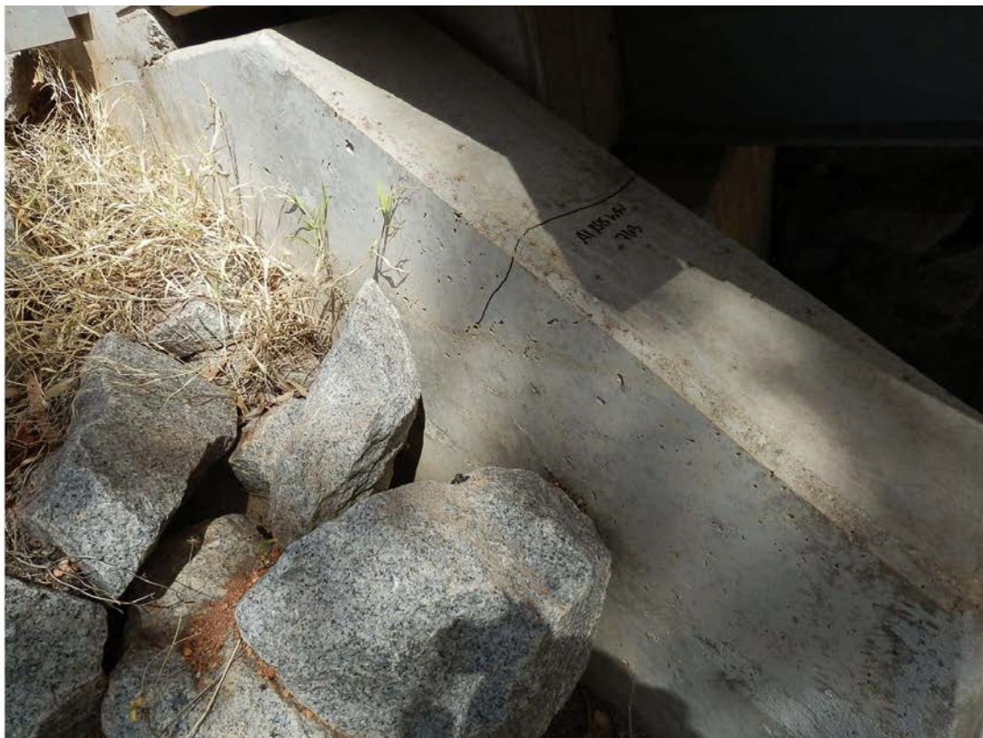
Photo No. 24: Abutment 1 right hand side wing wall. 0.15mm crack to top face of wall (Taken: 30-Jul-2013)
