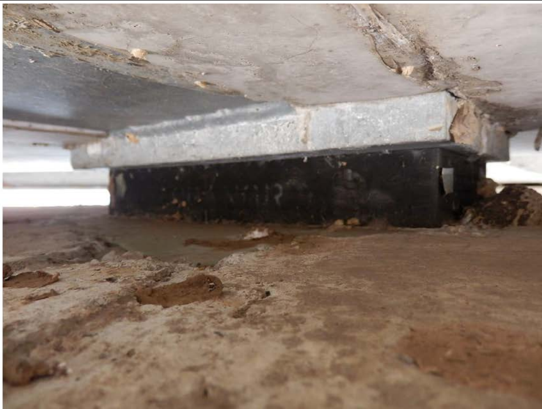
Photo No. 33: Pier 1 typical bearing pad in good condition. (Taken: 31-Jul-2013)
