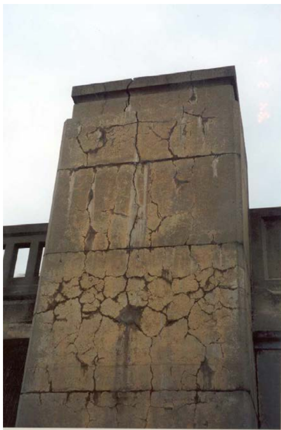
FIGURE 11.1B - CRACKING CAUSED BY ALKALI AGGREGATE REACTION
