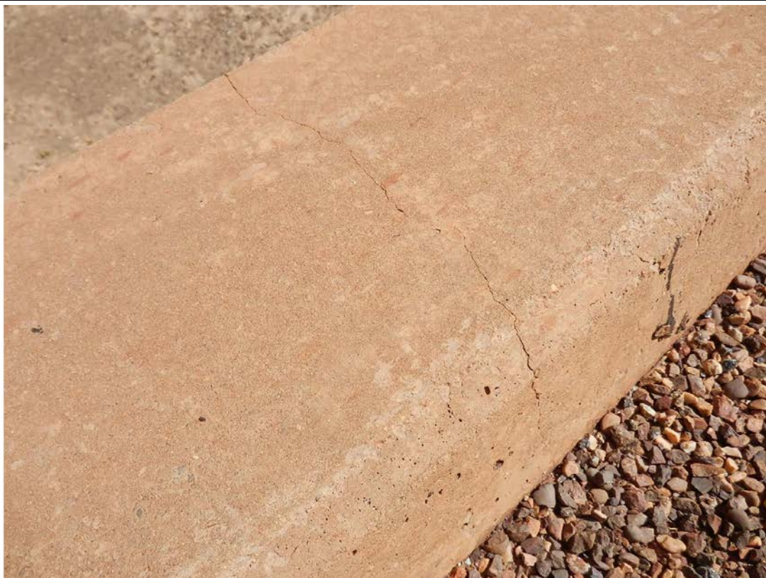
Photo No. 13: Typical cracking to kerbs on bridge deck. Left hand side shown here. (Taken: 30-Jul-2013)
