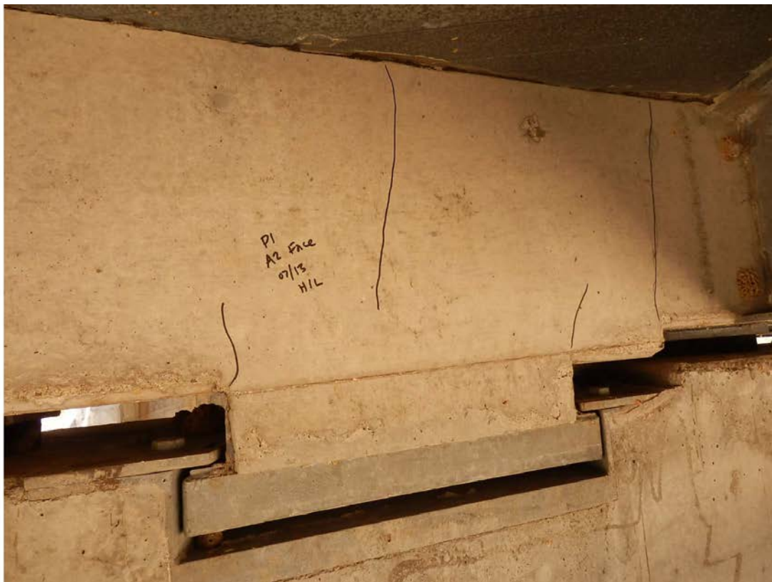
Photo No. 32: Pier 1 shear key/ diaphragm. Abutment 2 face. (Taken: 31-Jul-2013)
