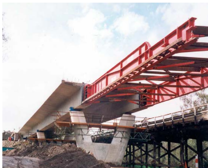
FIGURE E.2.2G(3) - INCREMENTALLY LAUNCHED DOUBLE T-BEAM
