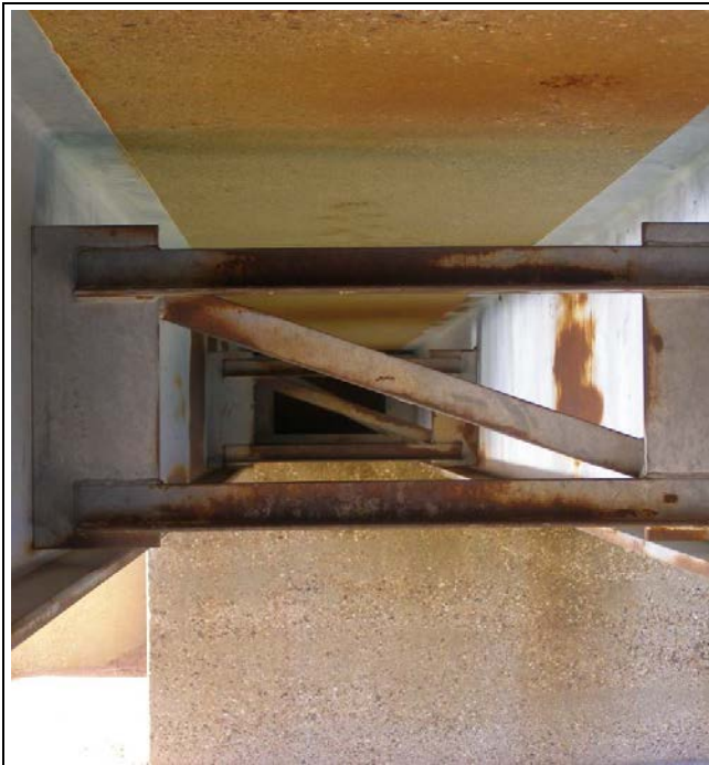
Localised surface corrosion, more prevalent in areas of greater exposure, no section loss.
