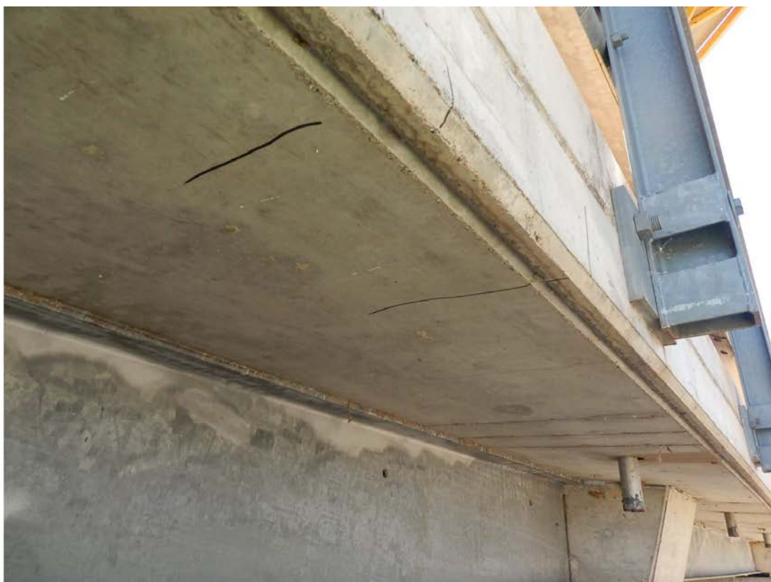
Photo No. 28: Hairline cracking to right hand side cantilever of span 1. (Taken: 31-Jul-2013)
