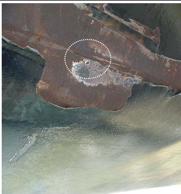
Example of impact damage. This warrants a CS4 as the box section has been torn.
