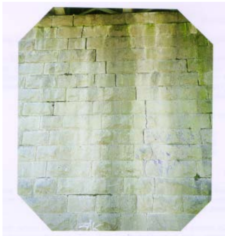
FIGURE 13.1 - CRACK IN MASONRY WALL
