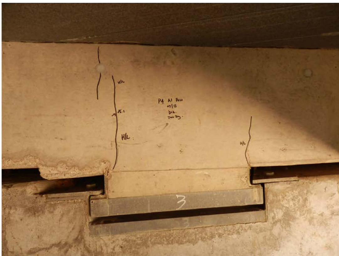
Photo No. 54: Pier 4 abutment 1 face. Hairline cracking from internal corners of shear key up to plastic bolt hole form for the formwork during construction. (Taken: 31-Jul-2013)
