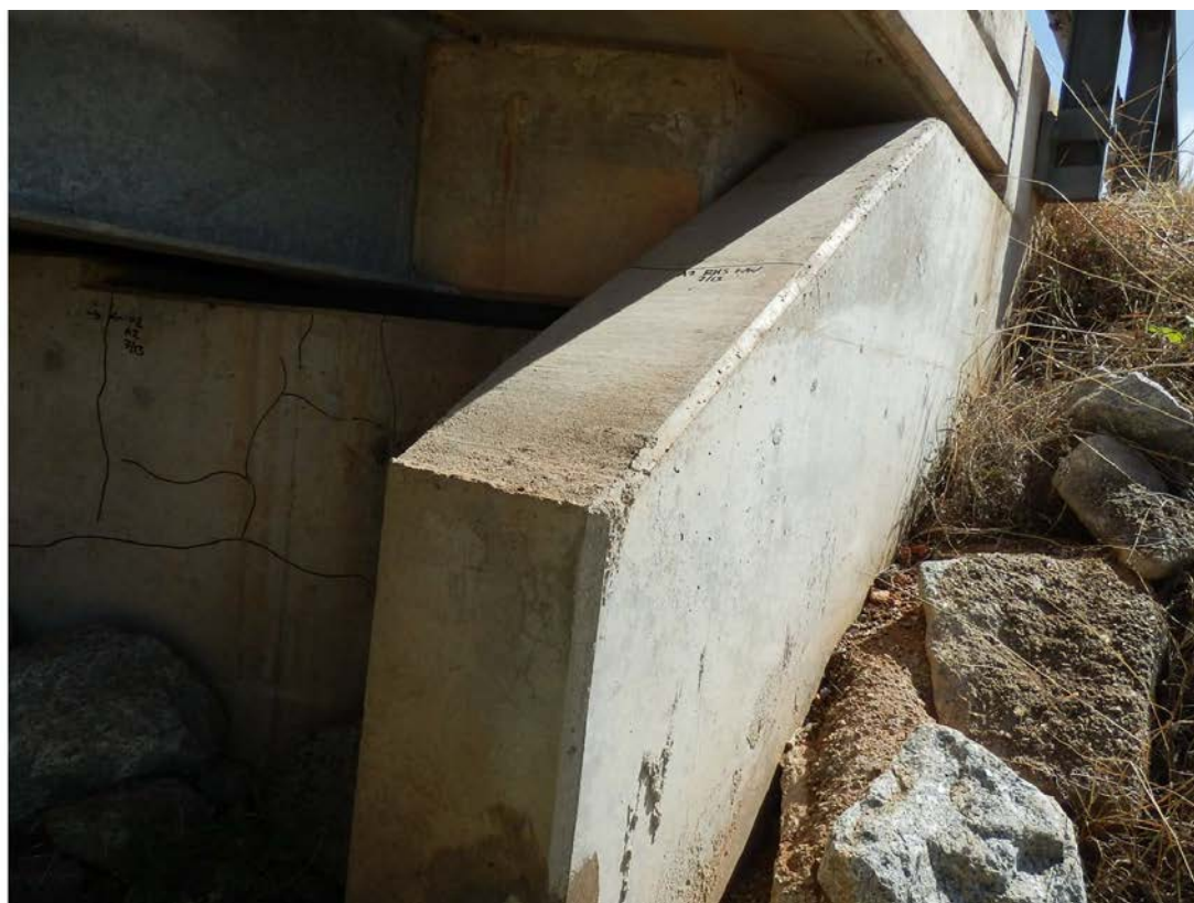
Photo No. 62: Abutment 2 right hand side wing wall. 0.15mm crack to top face of wall. (Taken: 30-Jul-2013)
