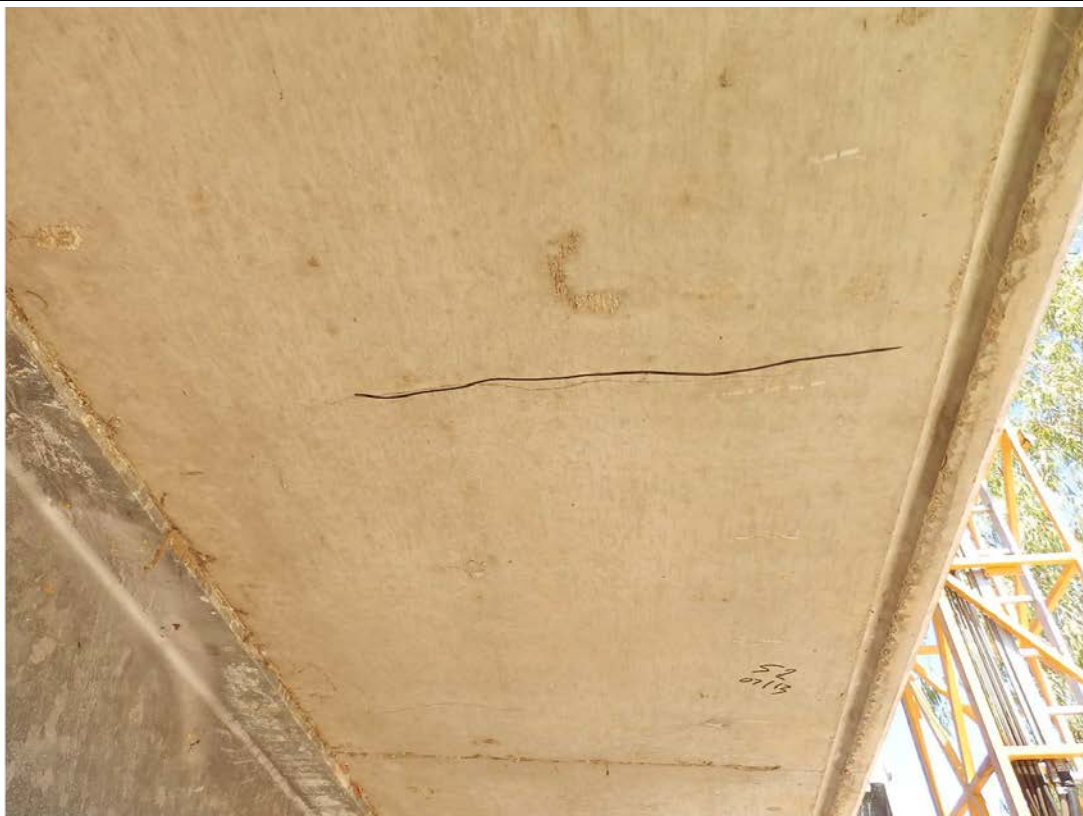
Photo No. 35: Span 2 left hand side cantilever. Hairline cracks. (Taken: 31-Jul-2013)
