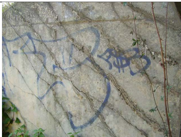
Heavy diagonal cracking of inlet wing wall.
