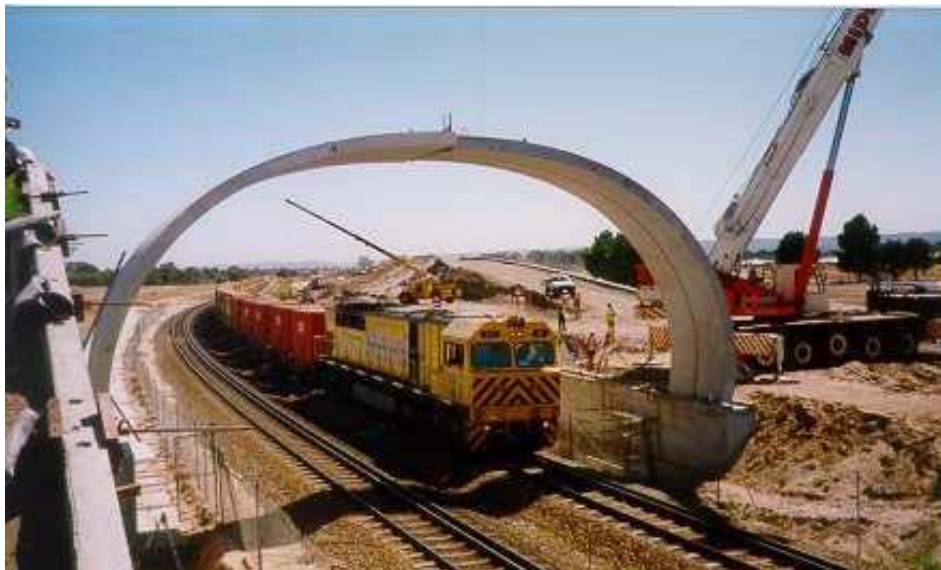
FIGURE E.2.1H(1) - REINFORCED CONCRETE PRECAST ARCH UNDER CONSTRUCTION
