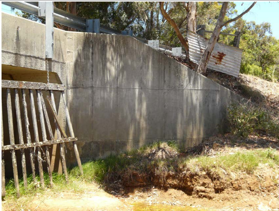
Photo No. 5: Wing Wall, Abutment 1 LHS – minor scour and tree close to wing wall (Taken: 14-Mar-2010)
