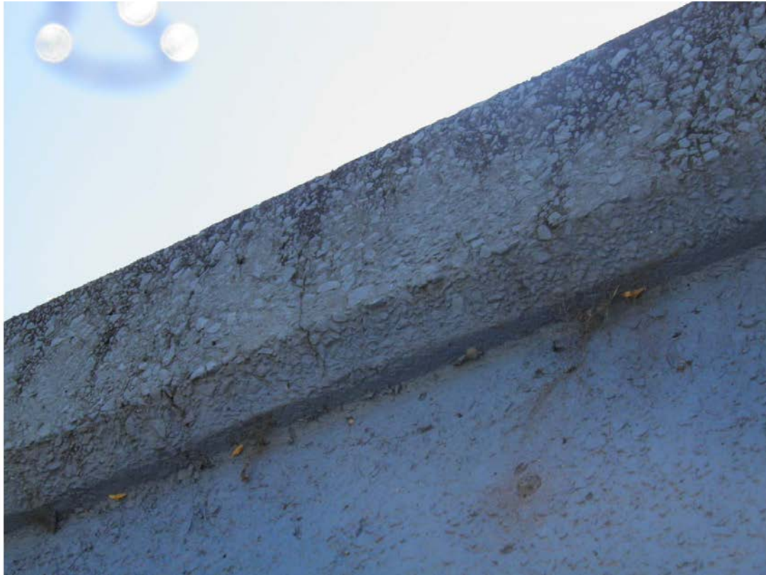
Photo No. 19: Cracks to abutment 2 left hand side head wall cap (Taken: 02-Nov-2016)
