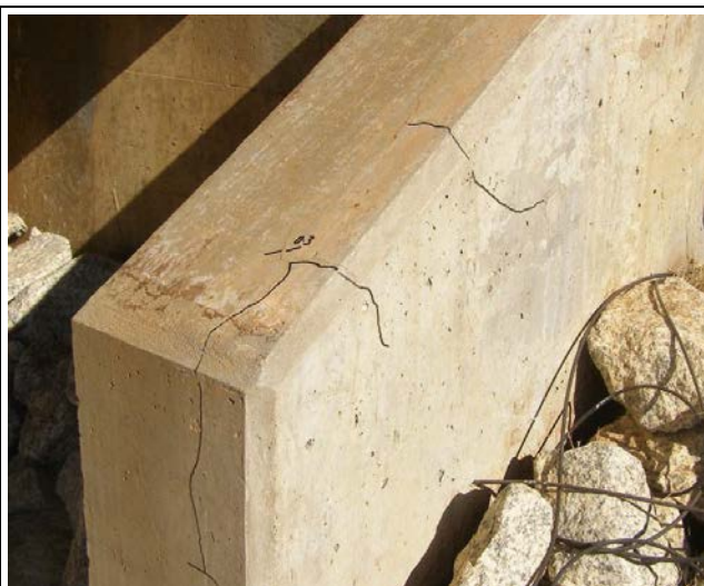
Medium cracks in the abutment wing wall, up to 0.4 mm.
