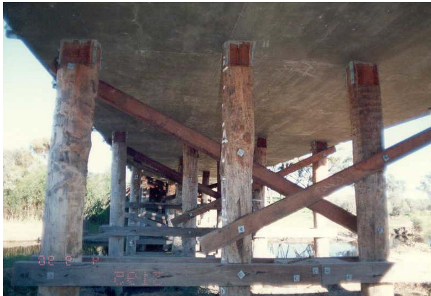
FIGURE E.2.6A - REINFORCED CONCRETE SLAB ON TIMBER SUBSTRUCTURE
