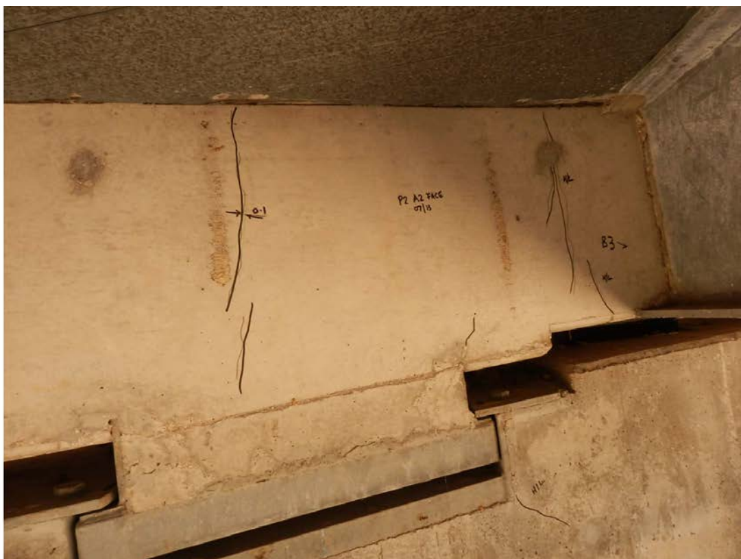
Photo No. 40: Pier 2 abutment 2 face. Hairline cracking (up to 0.1mm) at shear key. (Taken: 31-Jul-2013)
