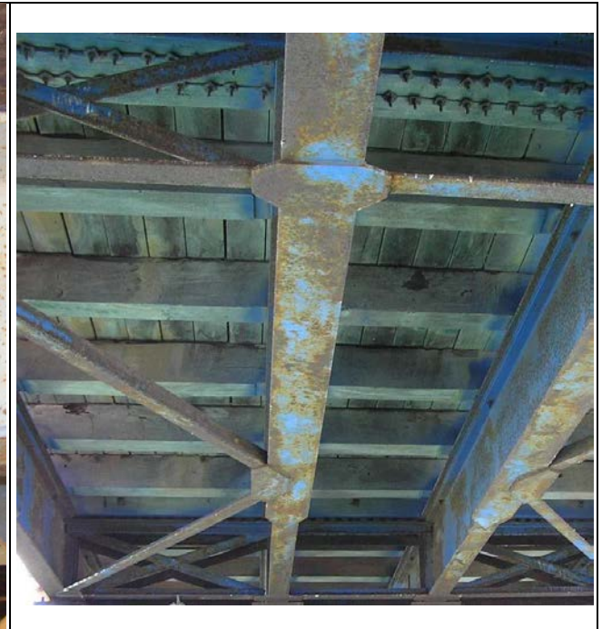
Quite widespread but superficial surface corrosion.
