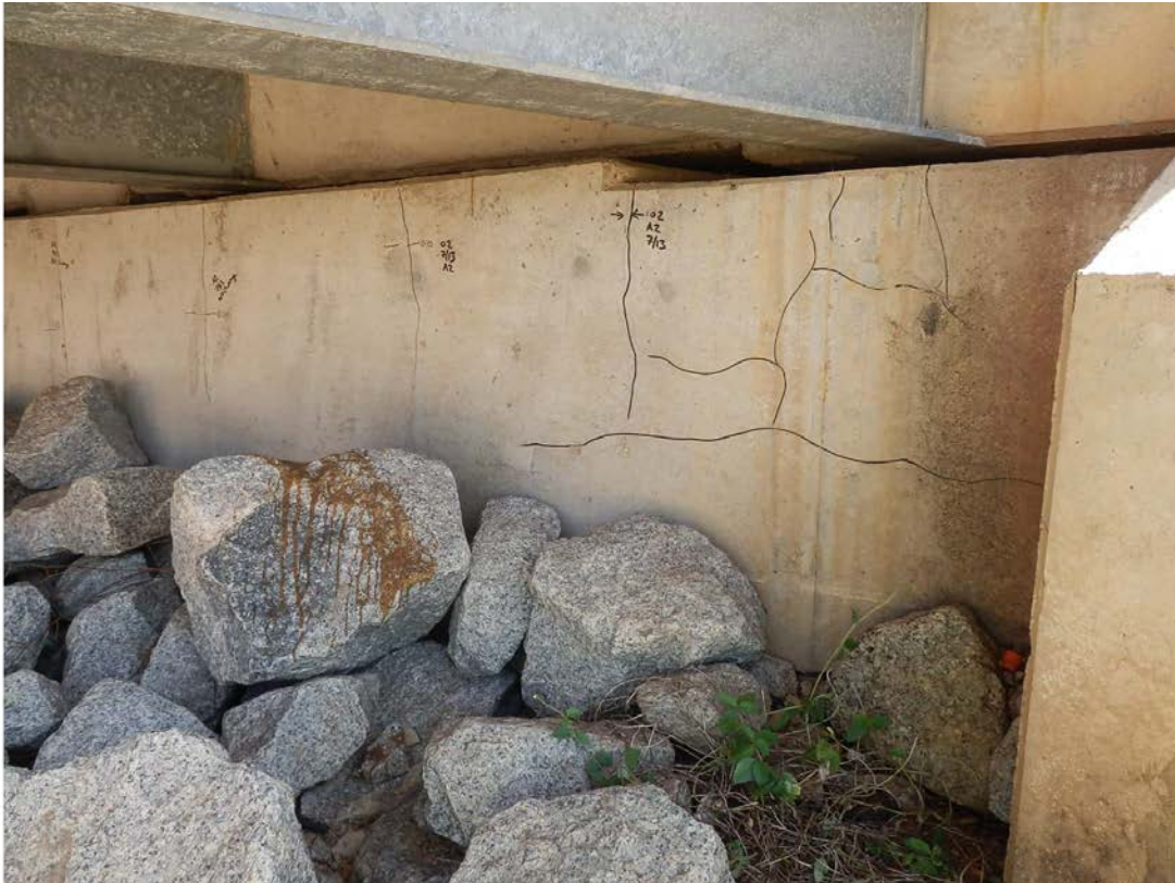
Photo No. 59: Abutment 2 capbeam. Various cracking, hairline, 0.2mm and 0.3mm. (Taken: 30-Jul-2013)
