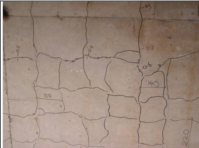
Deck slab block cracking, with cracks up to 0.6 mm.
