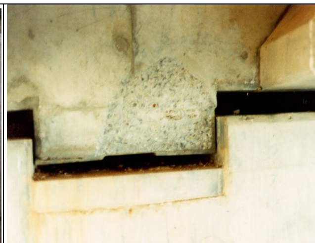
Single quite large spall. The spall is likely to have been caused by obstruction of movement and hence warrants CS3.
