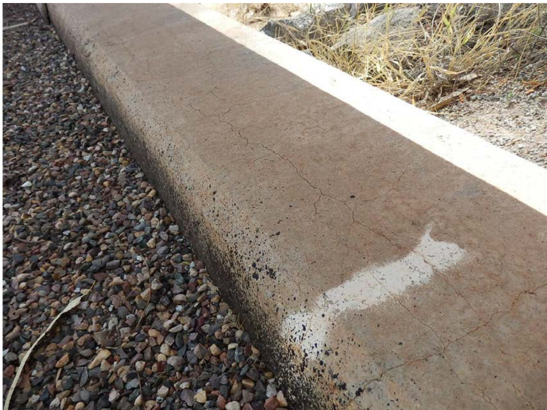
Photo No. 8: Various cracking to abutment 1 right hand side kerb. Concrete is solid. (Taken: 30-Jul-2013)
