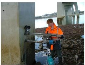
Figure 2 – Example of taking a core
