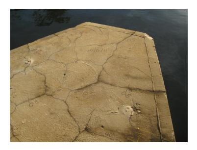
Figure 4 - Cracking due to AAR and related dampness
