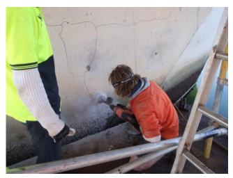
Figure 7 - Carrying out a breakout with a percussion core bit, with covermeter results lightly marked in red crayon
