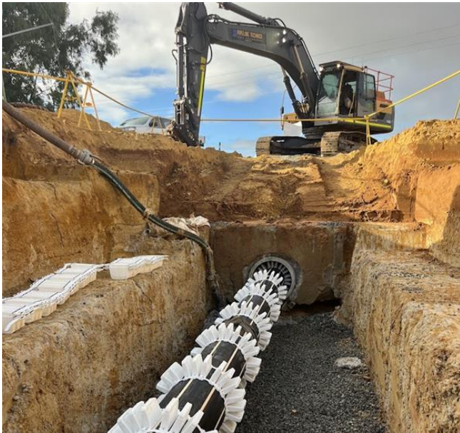
Sewerage pipe installation below Thomas Road.
