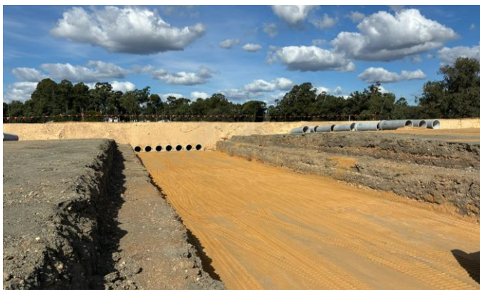
Drainage installation below Tonkin Highway.
