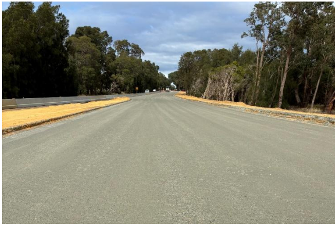
Basecourse along South Western Highway northbound.
