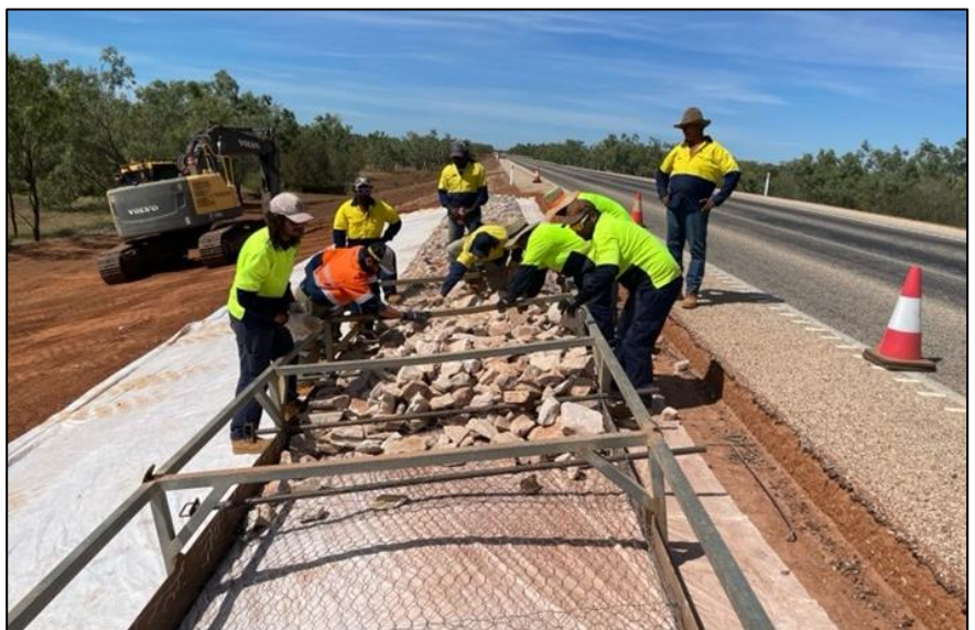
The three Aboriginal businesses and their employees working together to install gabion mattresses along Great Northern Highway
