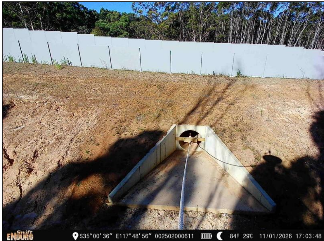
Photo 4a. Fauna underpass installed along George Street, between Fredrick Street and Cuming Road (looking east, camera 10).
