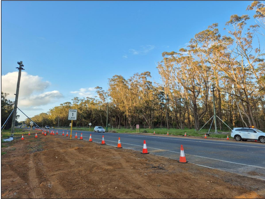
Photo 1. Installation of fauna bridge poles at Hanrahan Road (looking north east).
