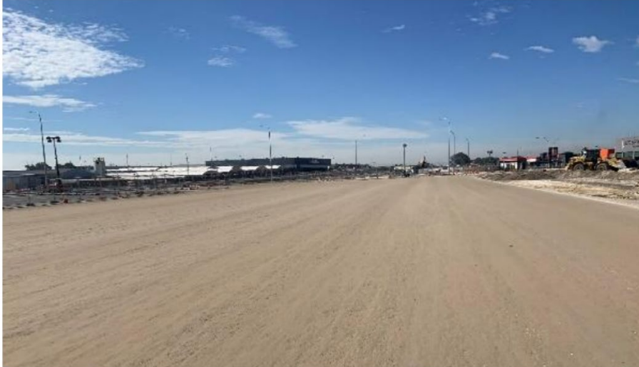
Figure 7 Trimmed and compacted CRC - Armadale Road North Lake Road Bridge Project
