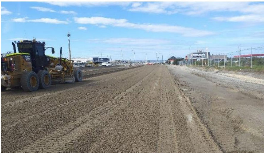
Figure 6 CRC - Armadale Road North Lake Road Bridge Project
