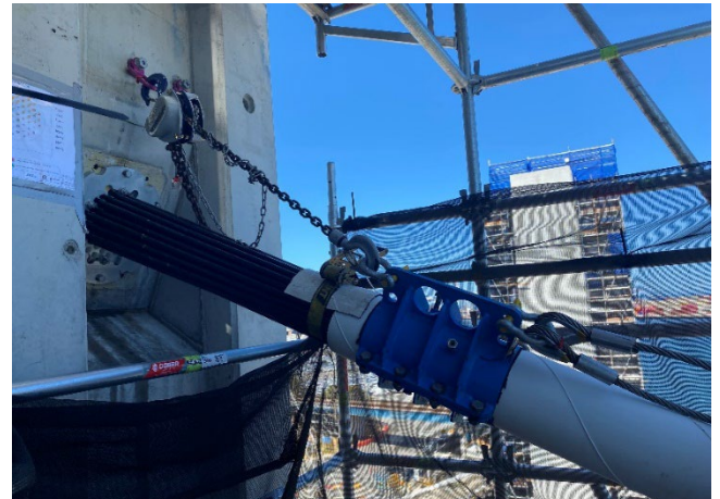
Figure 2: Cable stay concrete saddle at the top of the tower.
