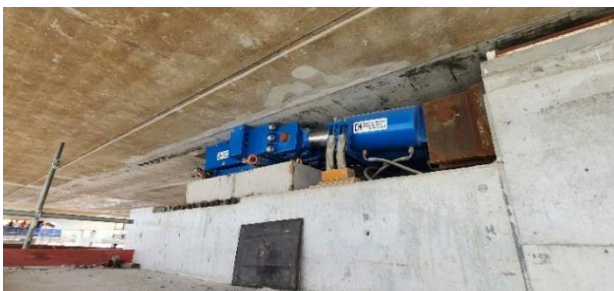
Image: The launching pad used to push the bridge segment 2.5cm per lift
