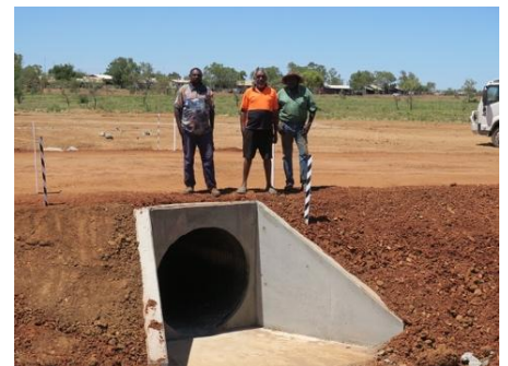
Proud Yiyili residents with community in background, L-R: Jason Cox, worker; Paul Cox business owner, and Terrence Dawson Snr, father of worker
