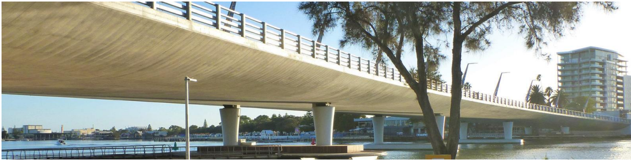
Mandurah Traffic Bridge
