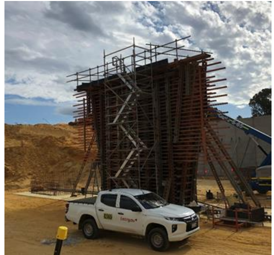
Example pier column and formwork before concrete is poured
