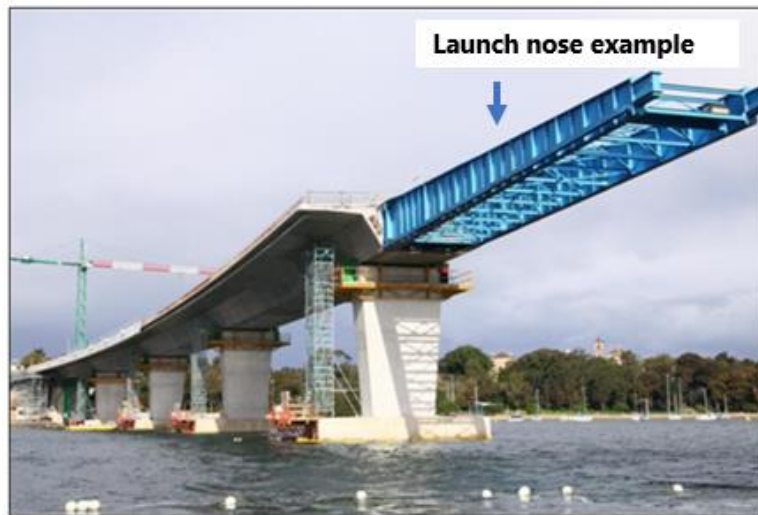
Incremental launch bridge example
