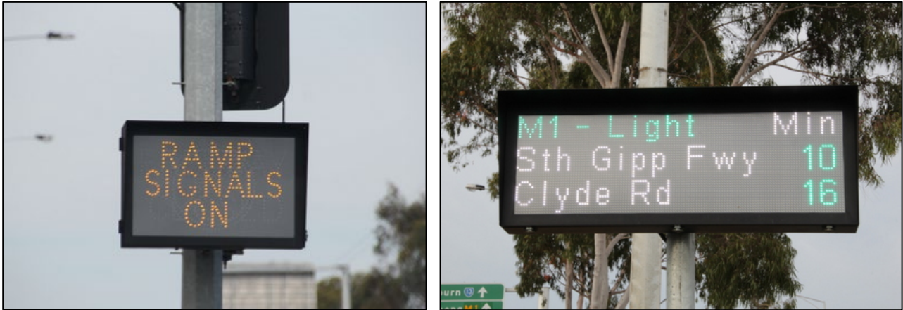
Figure 7-1 Example of an RC1 sign (left) and arterial road VMS (RC3) (right) in operation
