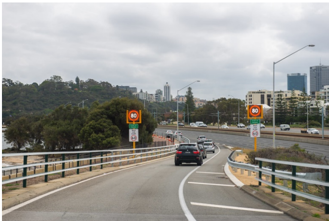
Figure 13-1 Example of side-mounted VSL sign
