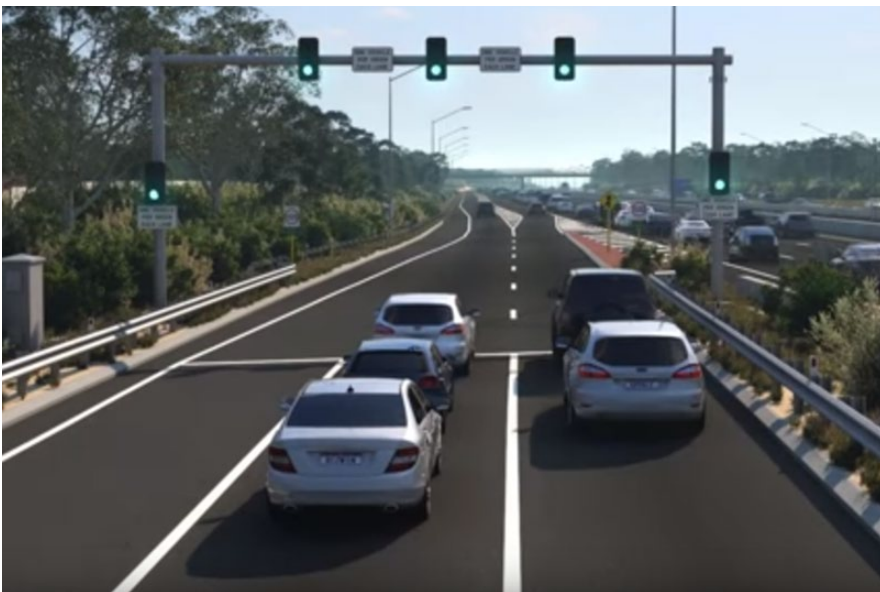
Figure 2-1 Coordinated ramp signals on the entry ramps of the freeway
