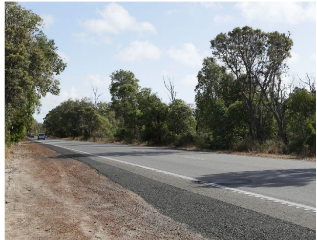
Photo 18 Dense vegetation within median, Bussell Highway near Woods Road.
