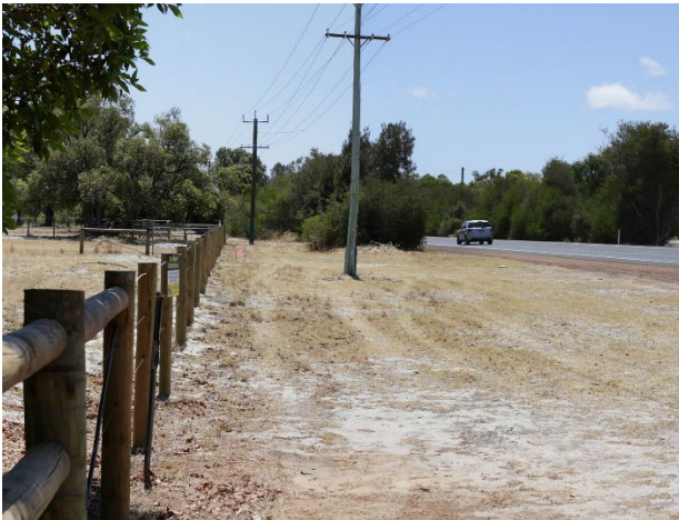
Photo 17 Residential property interface, Bussell Highway near Jaymon Road.
