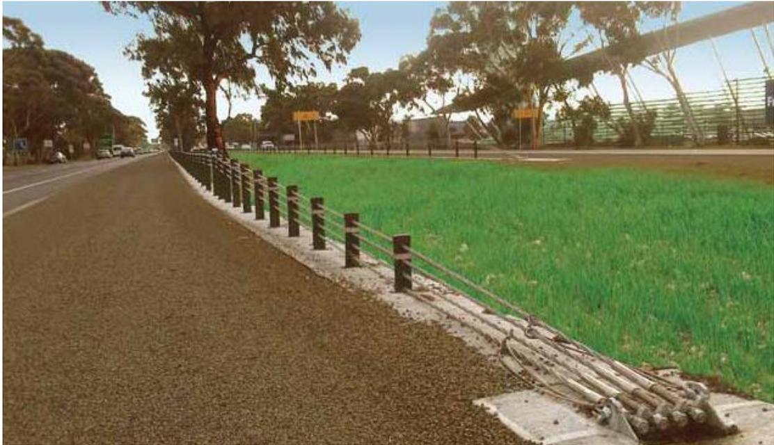
**Photograph of installed Flexfence TL3 Terminal
