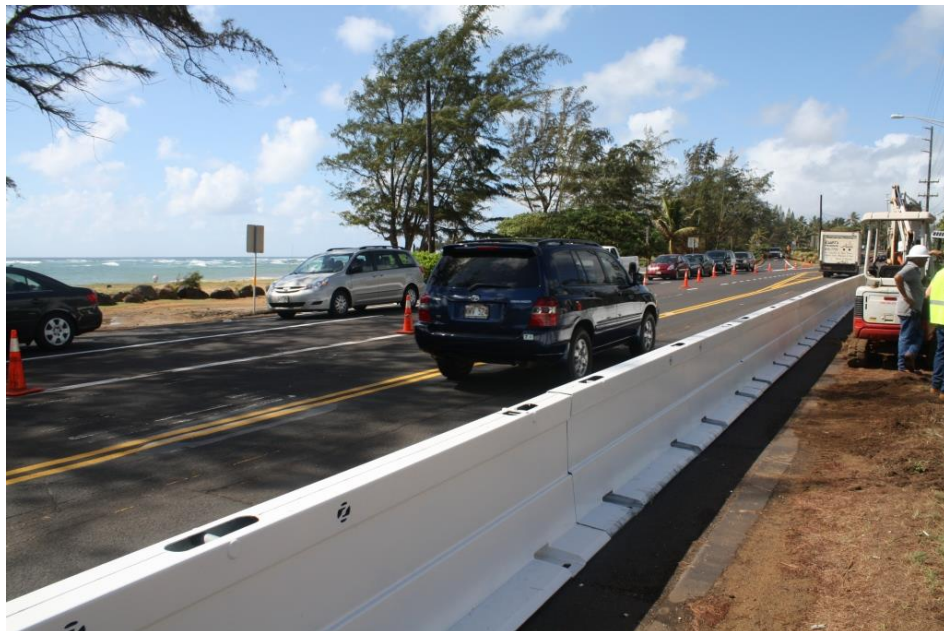
Photograph of ZoneGuard installation
