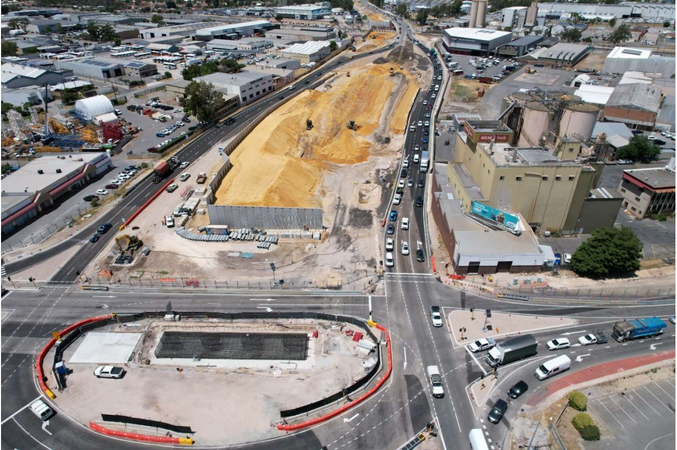
The temporary alignment of Leach Highway and the Welshpool Road intersection.
