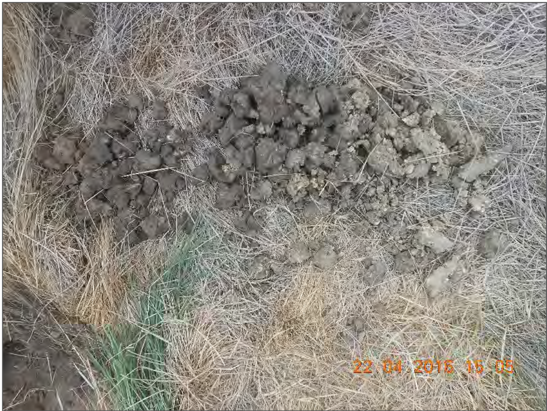
Photo 9: CH41900 limestone gravel entering near base of borehole
