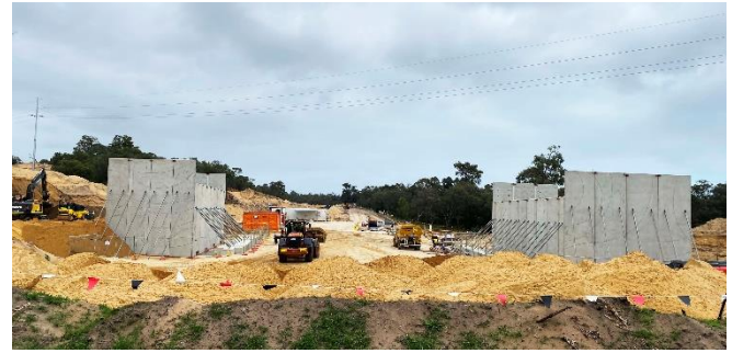
Erected wall panels with the recessed fauna design
