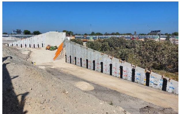
Malaga footbridge construction
