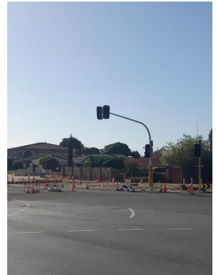
Broun/Embleton intersection works
