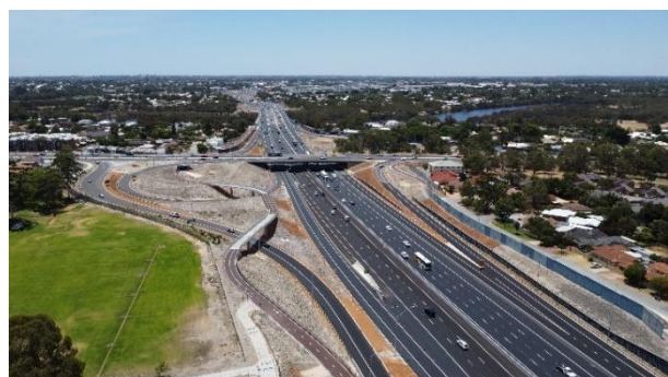
All lanes running on Tonkin Highway
