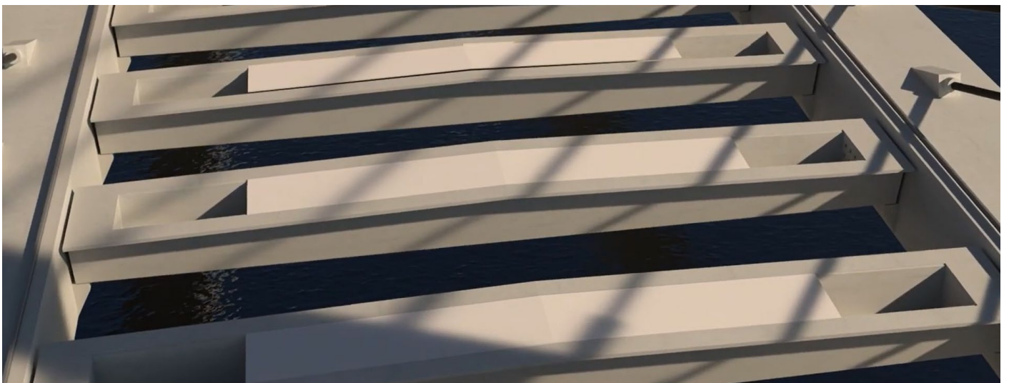
Figure 14: New bridge deck T-Roff beams.
