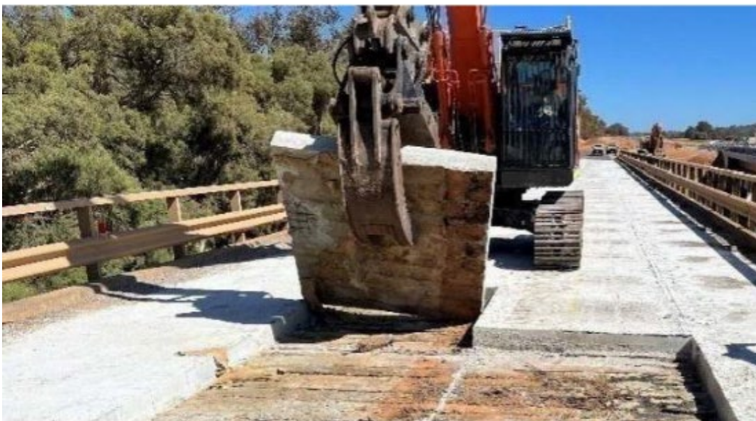
Figure 2: Example image of concrete deck removal.
