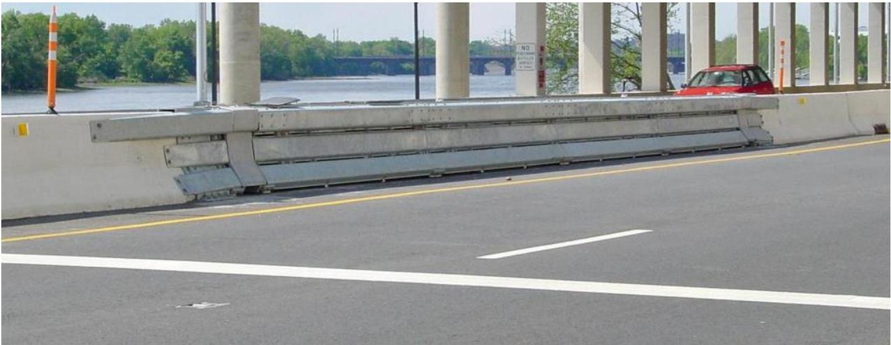
Photograph of ArmorGuard Gate installation
