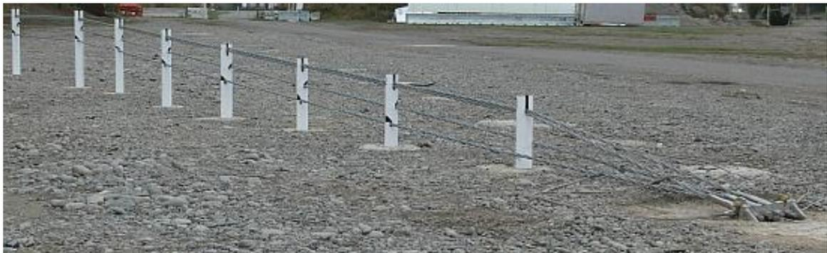
Photograph of Sentryline III end terminal installation.
