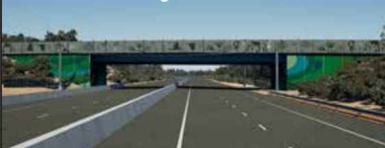
Yalinda Drive bridge
