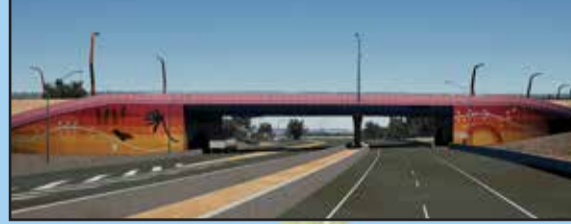
Paris Road and Clifton Road interchange
