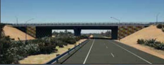
Raymond Road interchange
