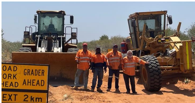
Above: J7M Contracting undertaking works in Yakanarra.
