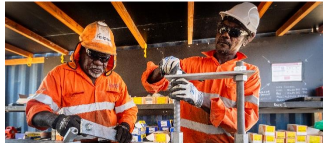
Above: Workers proofing bolts for the bridge.
