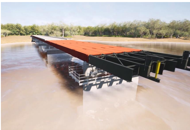
Above: Incremental launch bridge with launch nose
