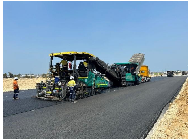
EME2 asphalt placement
