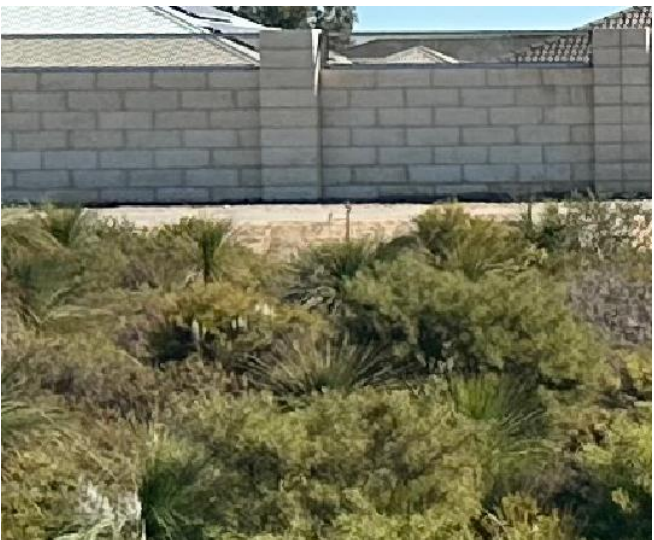
Top: LED lighting on the freeway; Middle: Eco-blocks used for noisewalls; Bottom: Vegetation saved.
