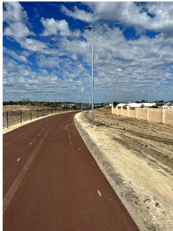
PSP being prepared for line marking.
