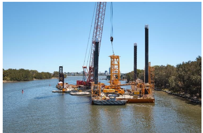
Figure 8 Piling in the river in the northern navigation channel
