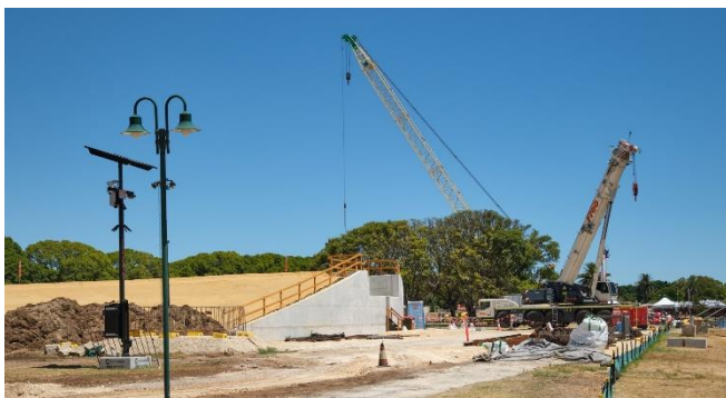
Figure 6 The bridge abutment constructed at McCallum Park
