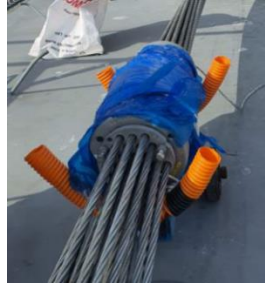
Figure 11 Each cable will have multiple steel strands inside.
