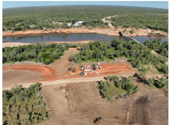
Above: Laydown yard on the west side of the river
