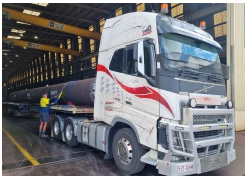
Above: Steel pile casing making its journey to site
