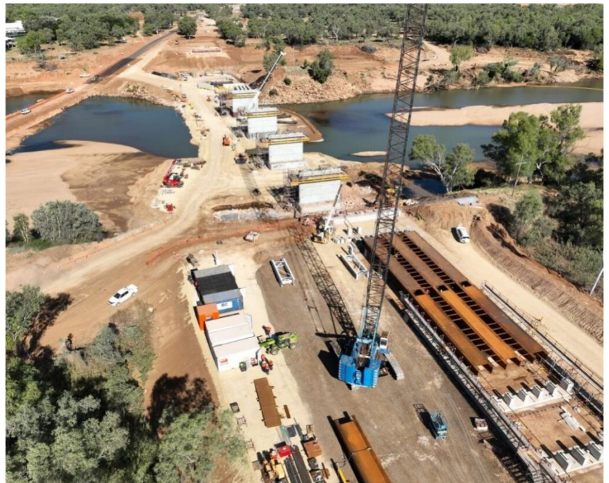
Above: Installation of the concrete pier shells underway
