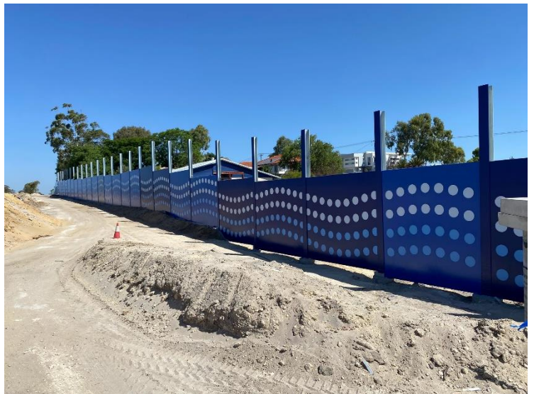
Painted noise walls behind Wyatt Road
