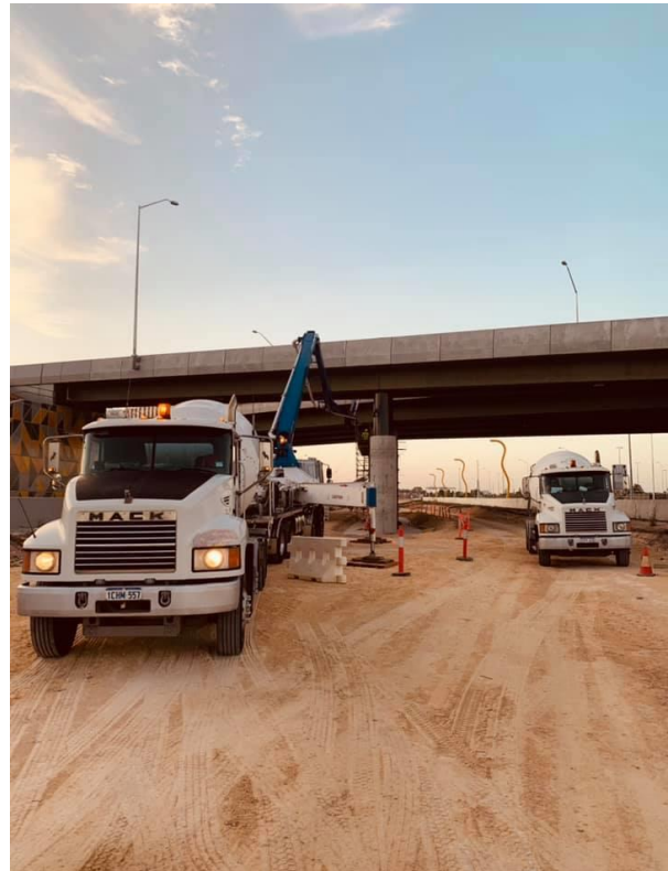
Concrete pours for pier protection
