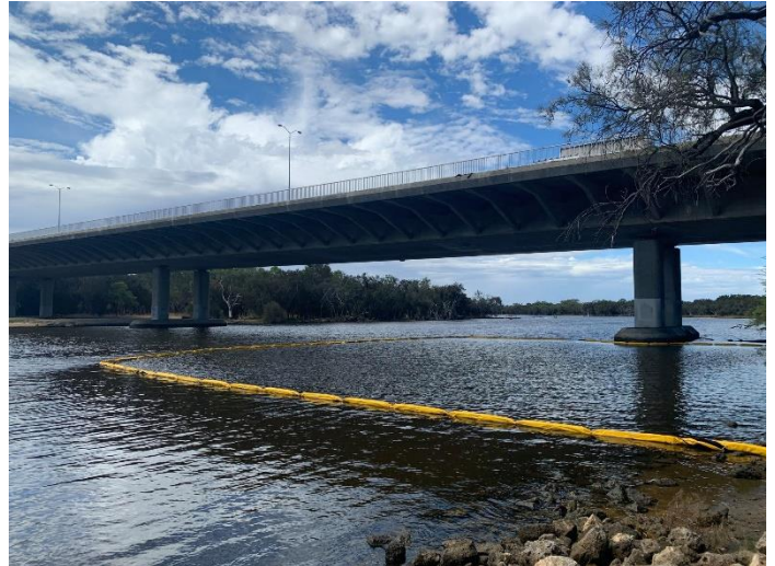
Silt curtain for cofferdam
