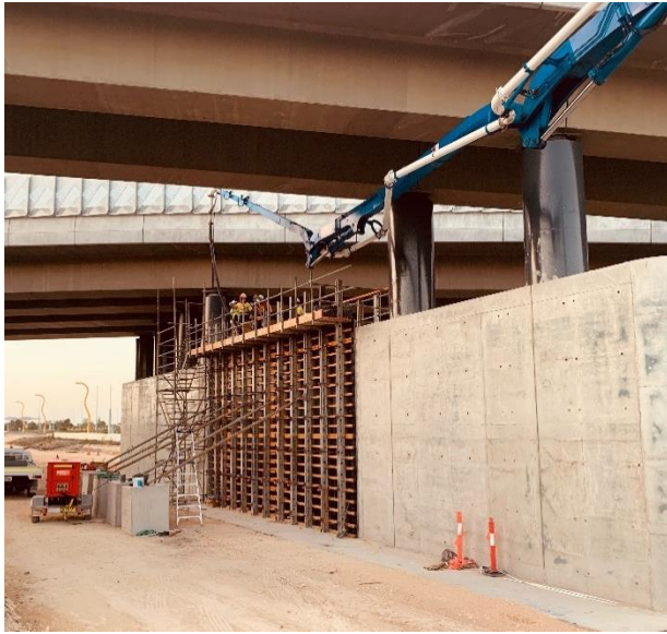
Concrete pours for pier protection
