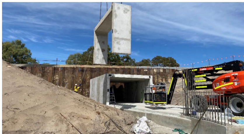
Benara Road Underpass
