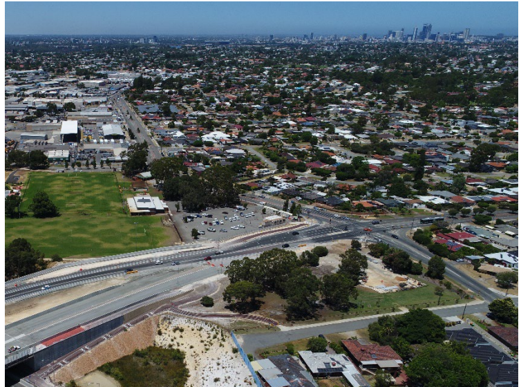
Broun/Embleton Avenue intersection works
