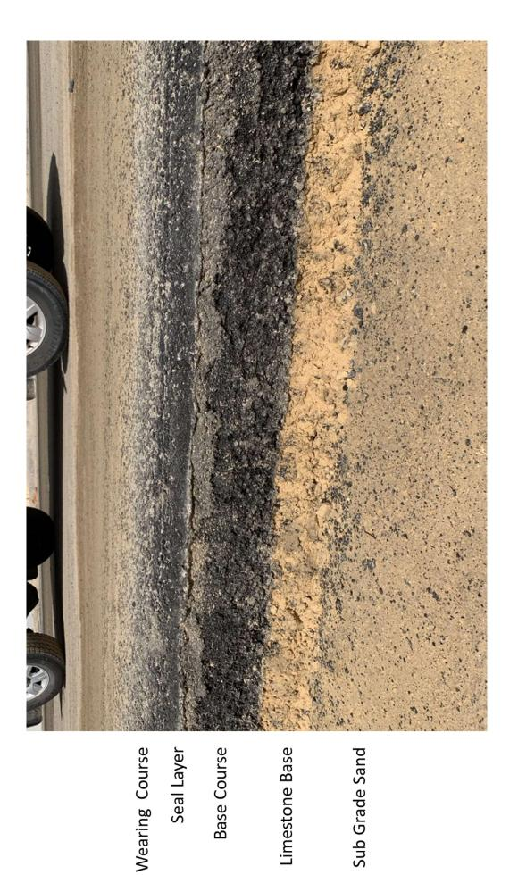
Representation of the layers required to construct the Mitchell Freeway southbound widening. Each layer requires compaction
