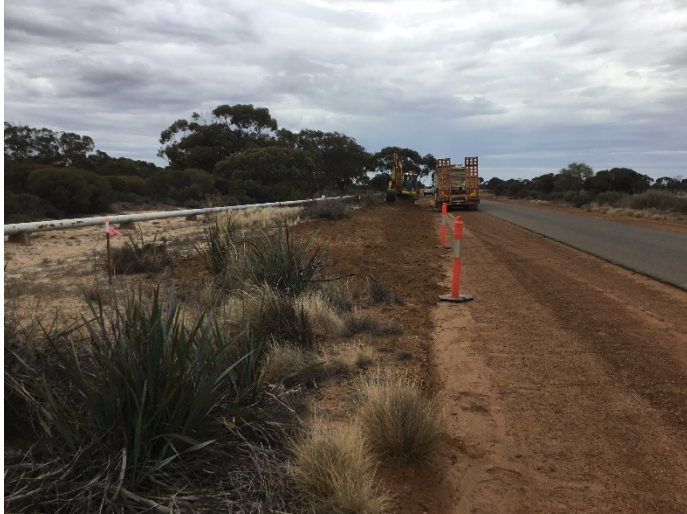
Photograph 1: Demarcation and topsoil stripping in location of Dampiera glabrescens prior to clearing
