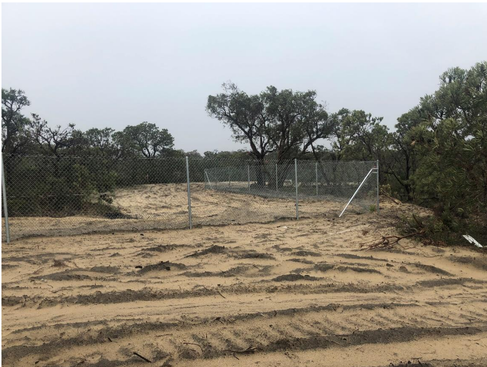
Evidence of fence installed, and an area of vegetation saved from clearing within the DE.
