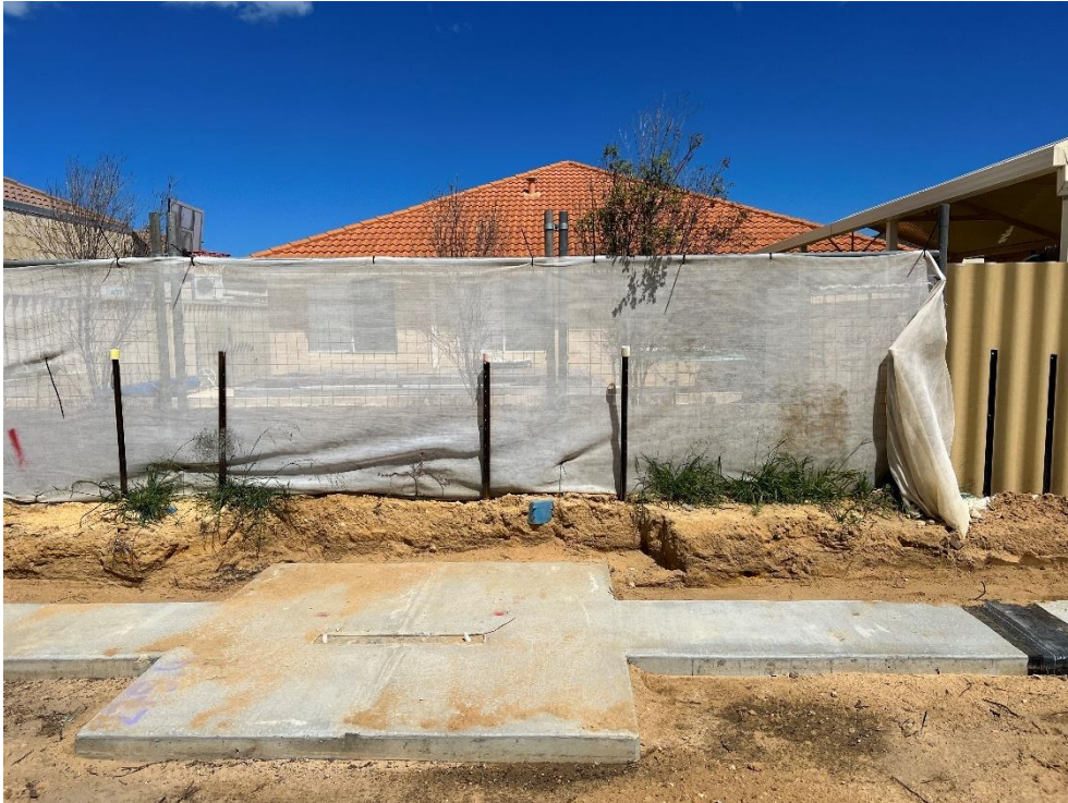
Dust netting erected on boundary between the project and residential neighbours
