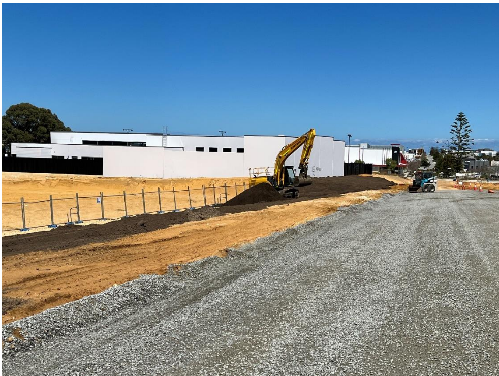
Topsoil spread at Butler Blvd
