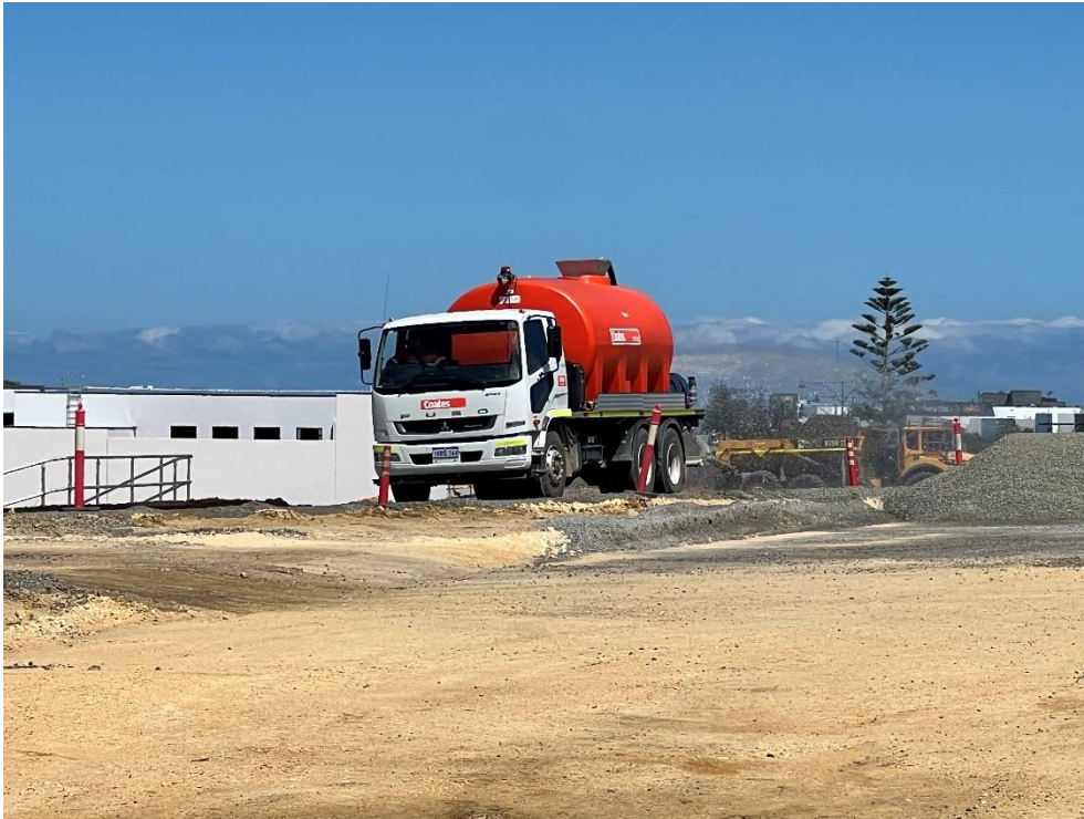
Water cart spraying general areas/batters
