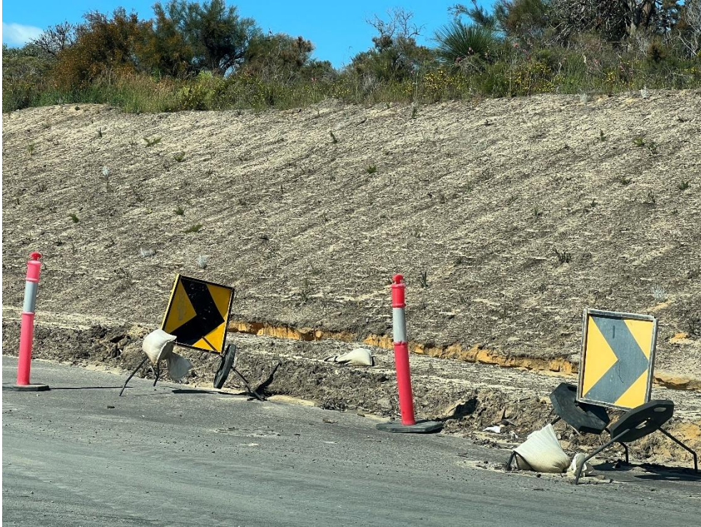
Batter along Mitchell Freeway that has been topsoiled/mulched and planted
