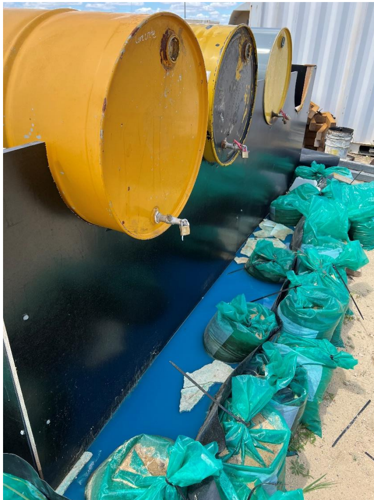
Observation No. 2 – bund for shuttering oil
