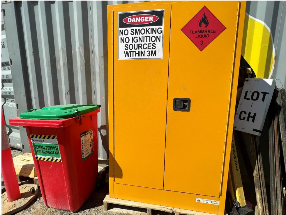
Hydrocarbons stored in a suitable cabinet at Romeo Rd compound. Spill kit adjacent.
