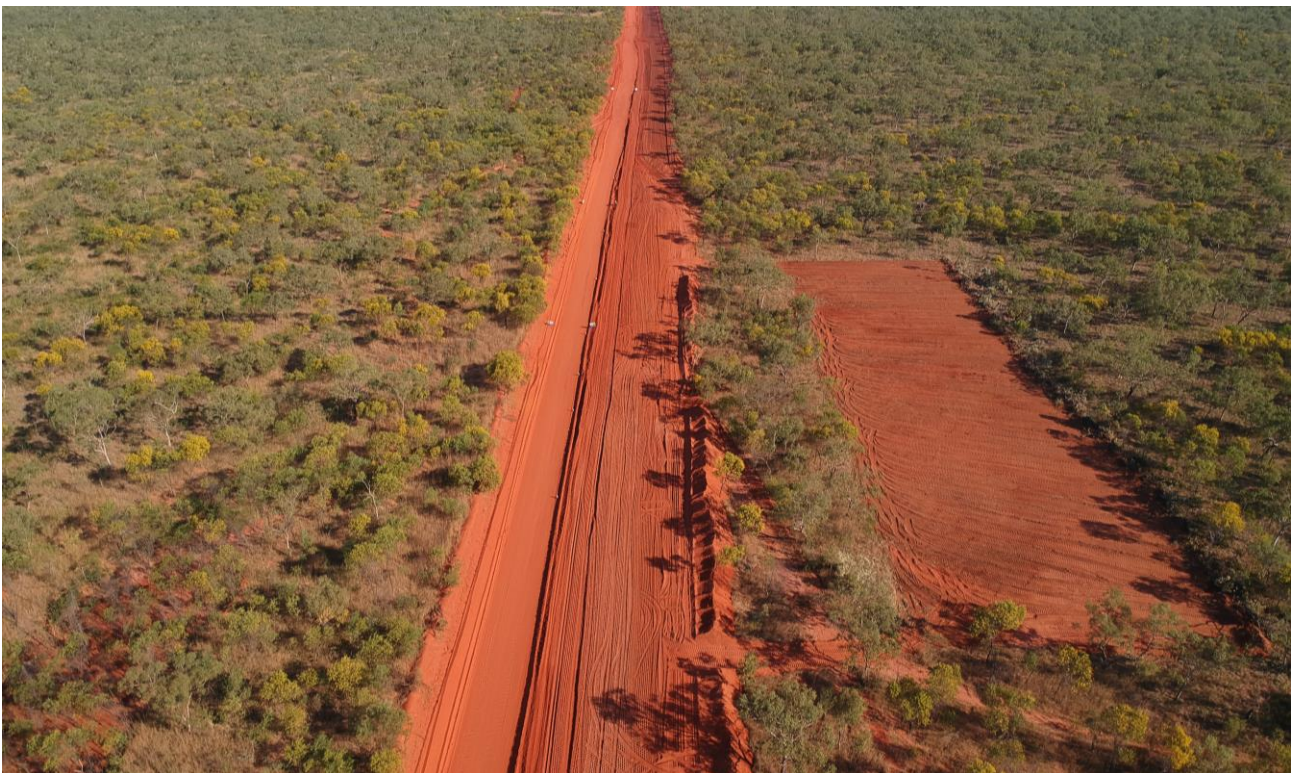
Figure 2. Aerial Imagery of clearing works at Design, and Construction Phases
